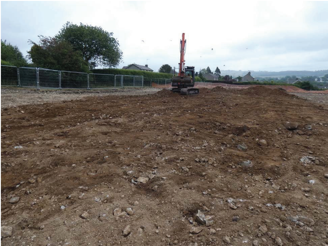
Plate 10: Removing deposit 122 by machine, viewed from the west
