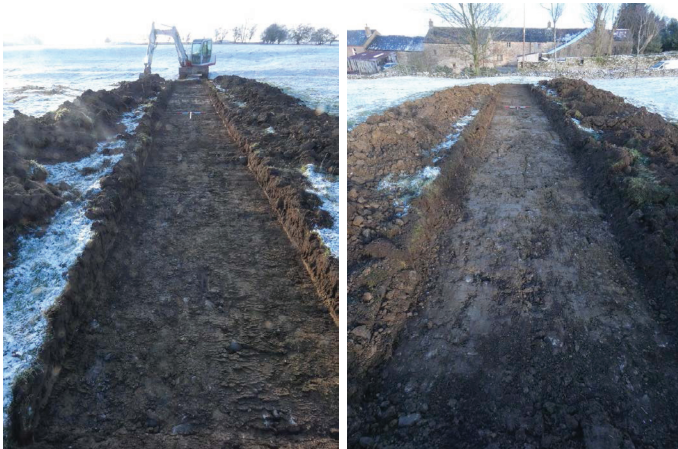
Plate 20 (left): Trench 5 viewed from the east
