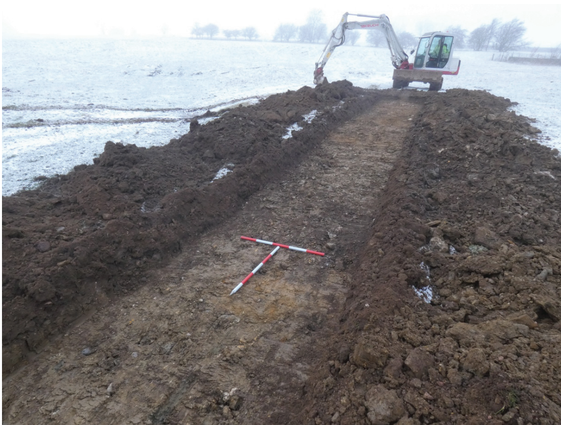
Plate 19: Natural (403) and darker patch of 402 in the centre of Trench 4
