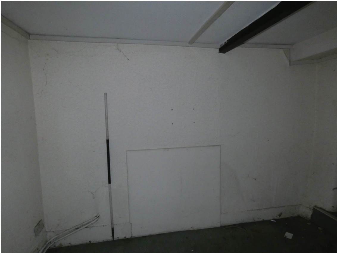
Plate 49: West elevation of G5
