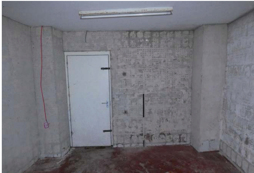
Plate 66: West elevation of G8
