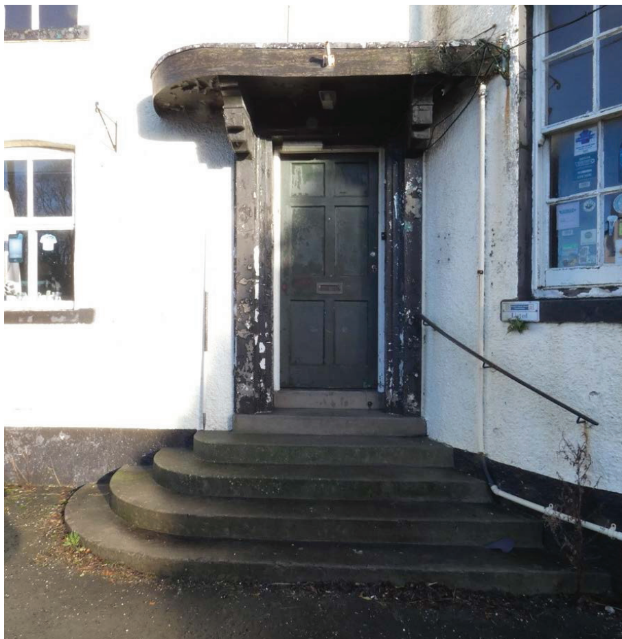
Plate 15: Central door on the south external elevation
