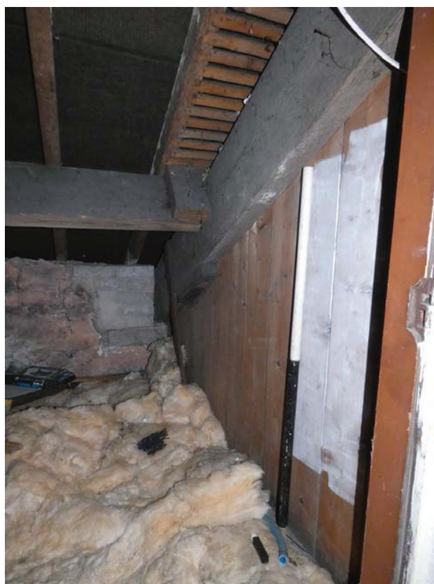
Plate 119: Roof space to the north side of S3
