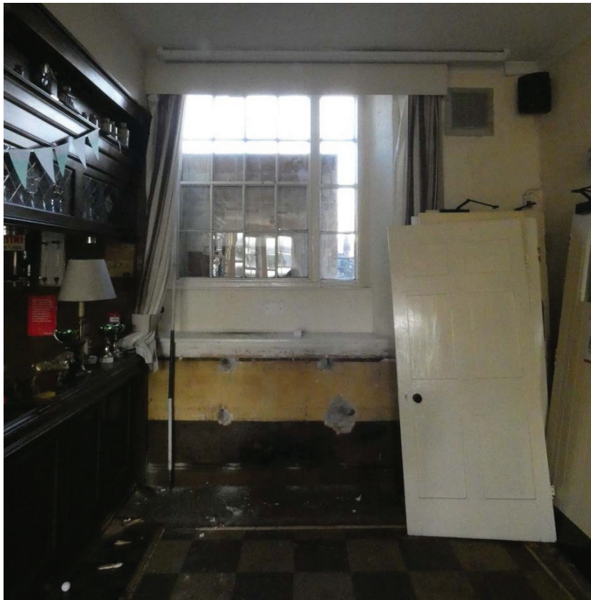
Plate 32: Window in the north elevation of G2
