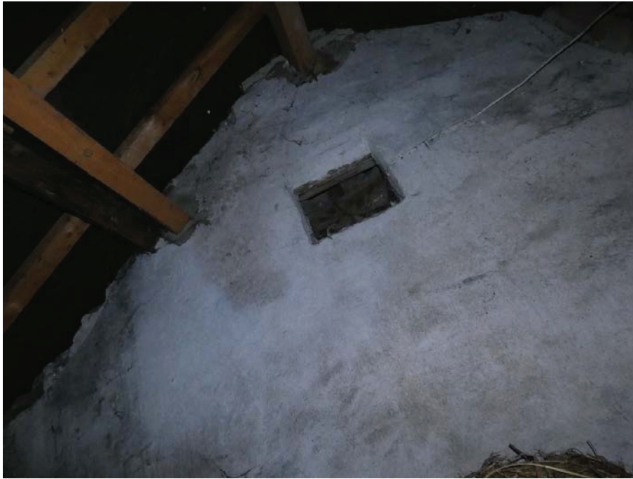
Plate 71: Roof space above G8, viewed from the south
