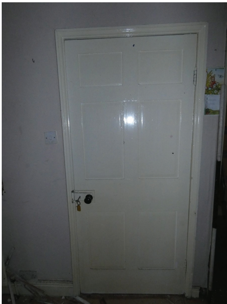
Plate 86: Door towards the north end of the east elevation of F3
