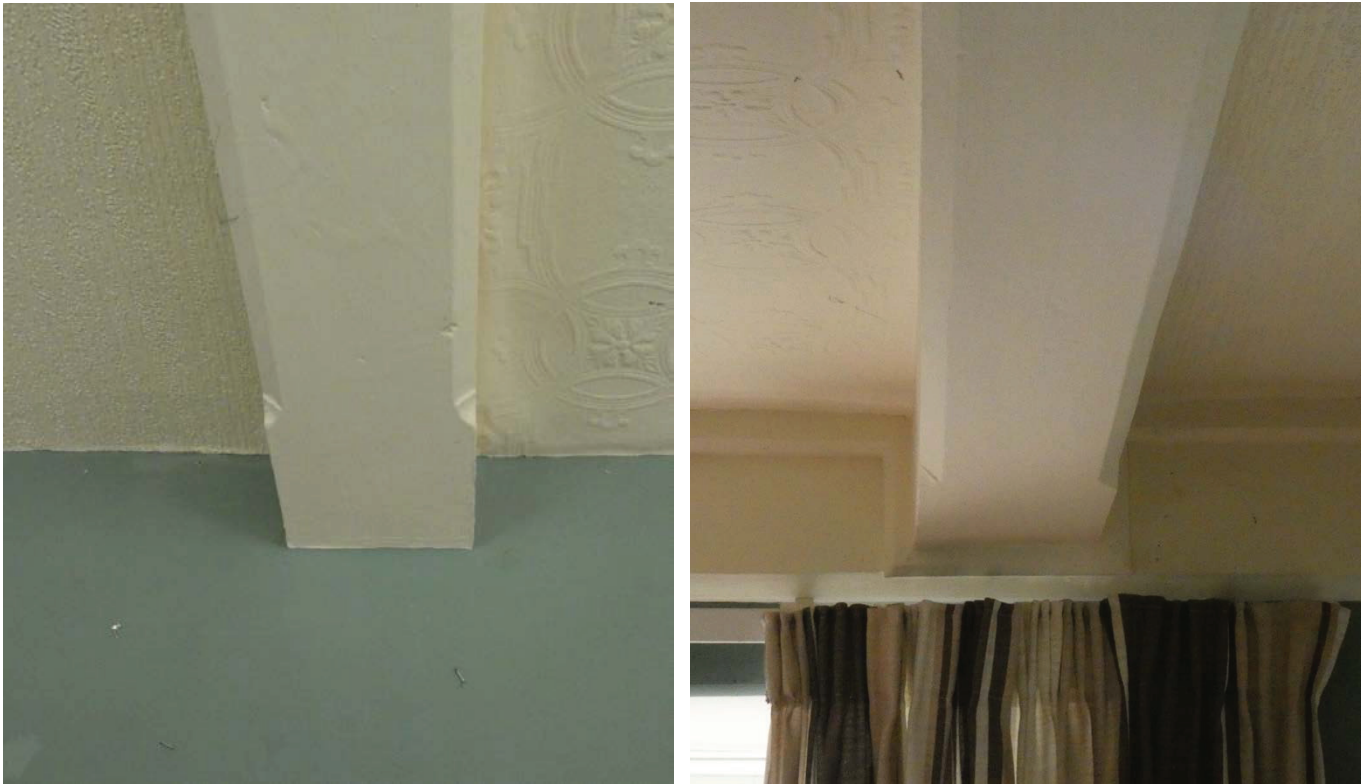
Plate 44 (left): Stop chamfer at the north end of the beam in G4
