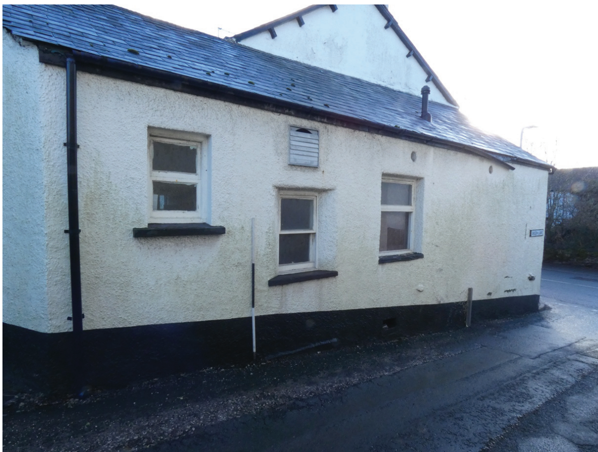
Plate 17: Central section of the west external elevation
