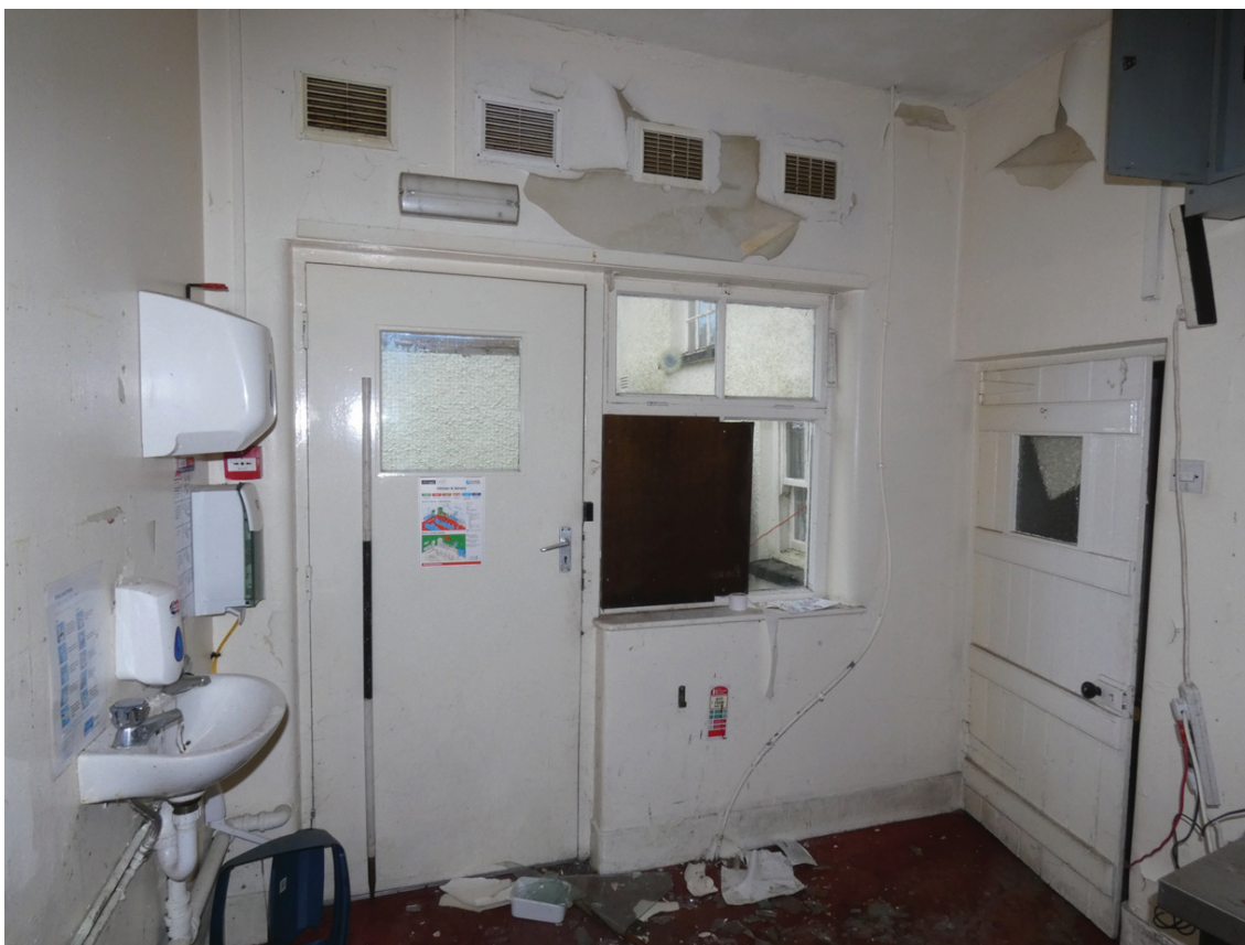
Plate 58: North end of the east elevation of G7
