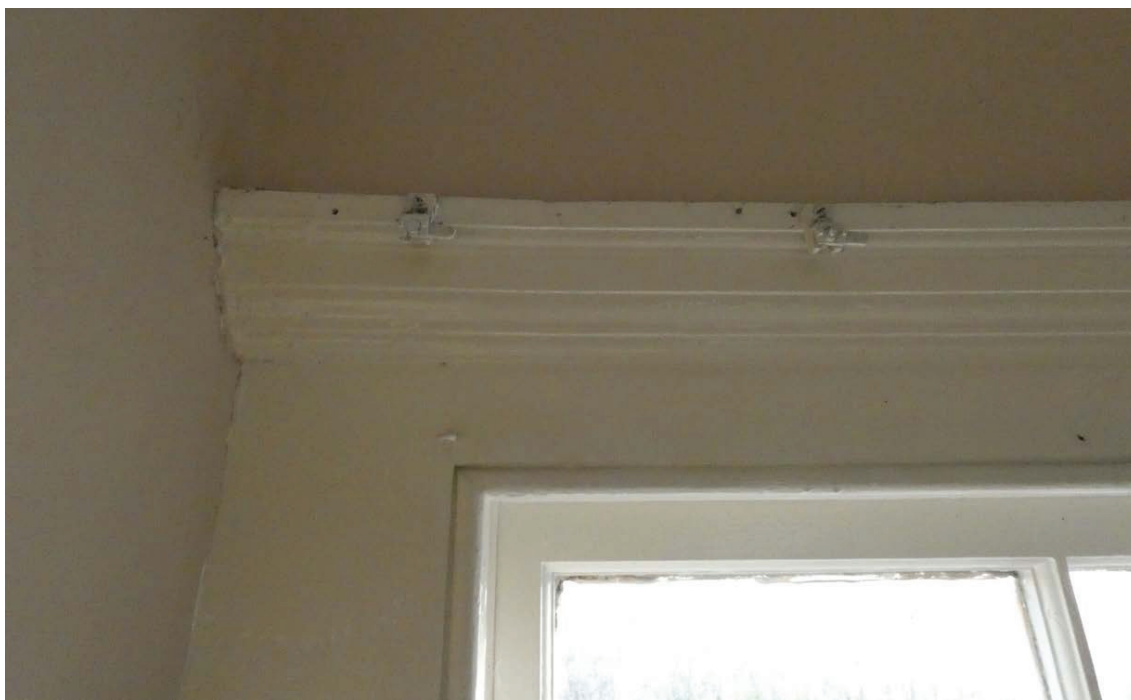
Plate 81: Moulding above the window in the south elevation of F2
