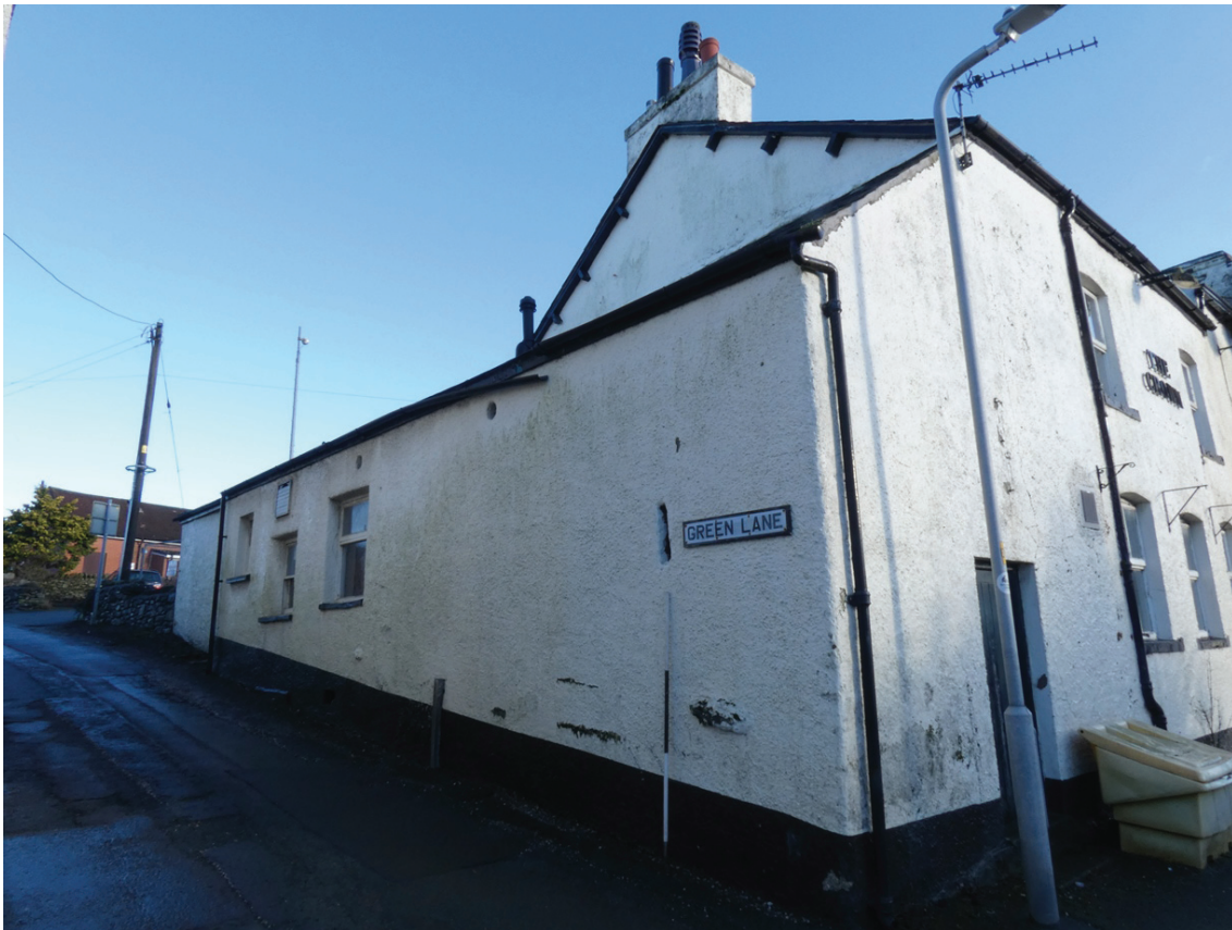
Plate 16: South end of the west external elevation
