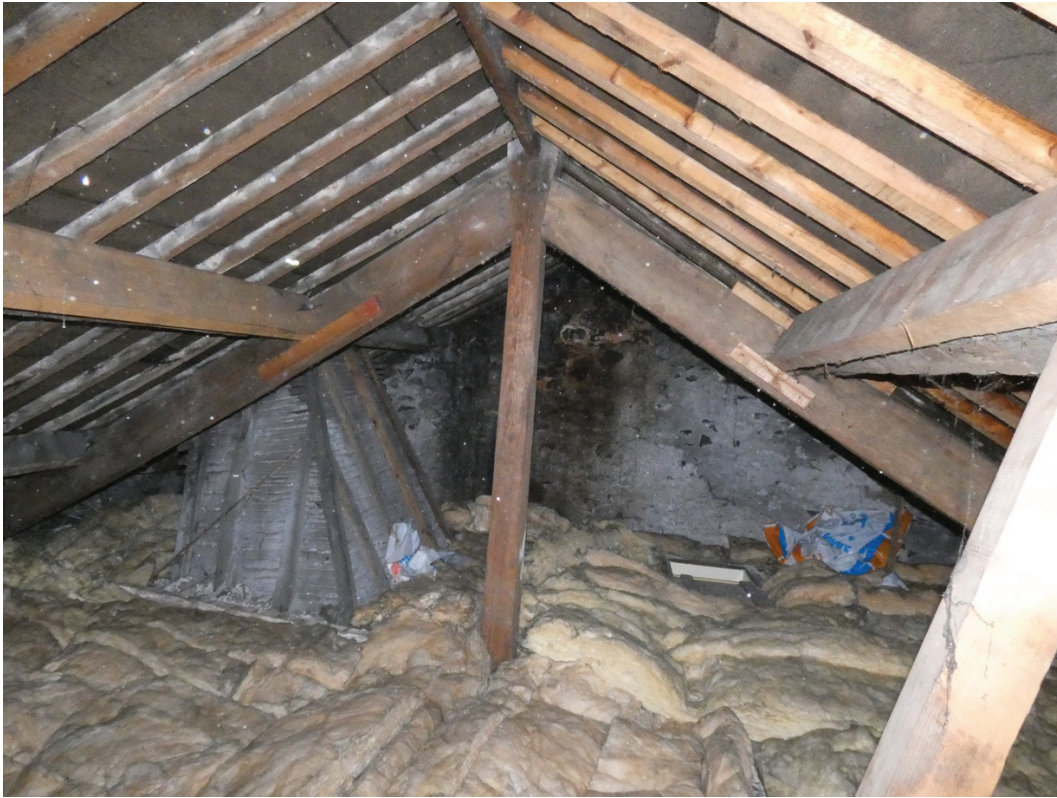
Plate 107: Truss above F2 and F3, viewed from the east
