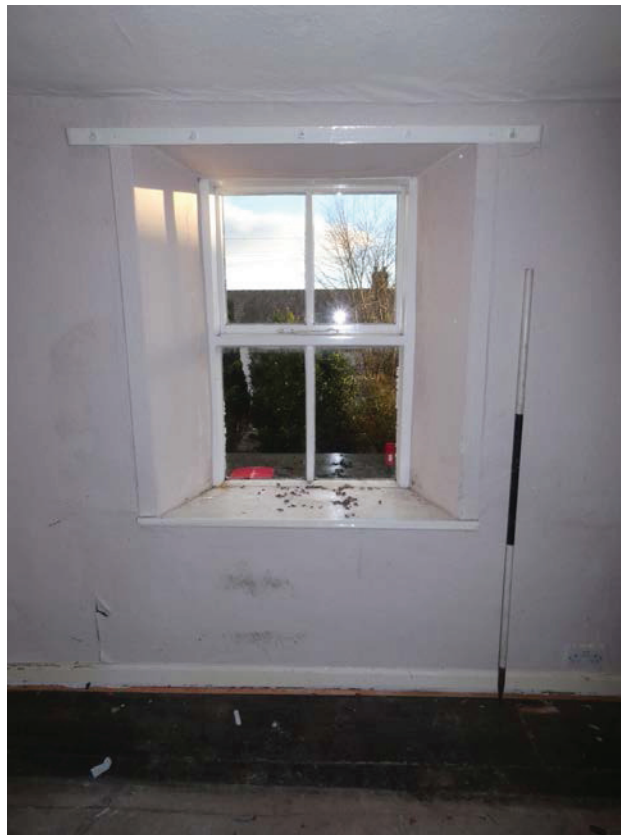
Plate 99: Window in the south elevation of F6
