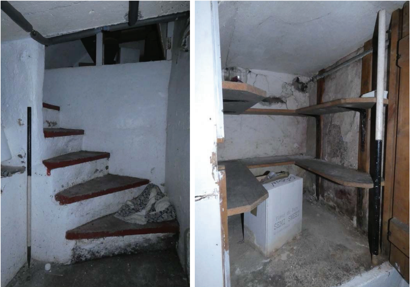
Plate 24 (left): Stairs to B2
