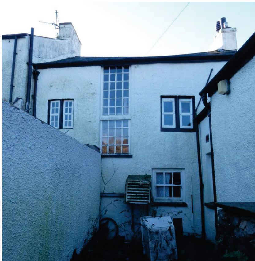
Plate 10: West side of the north external elevation of the main section
