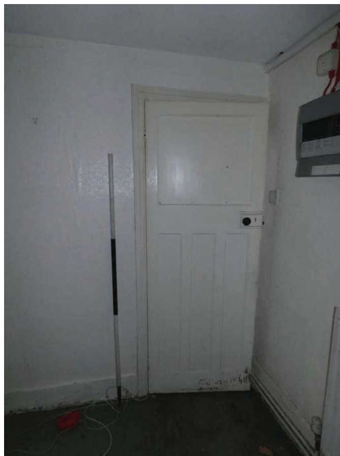
Plate 47: Door at the south end of the east elevation of G5
