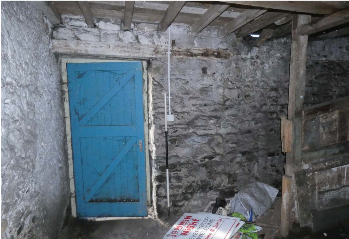
Plate 28: Door in the south elevation of G1
