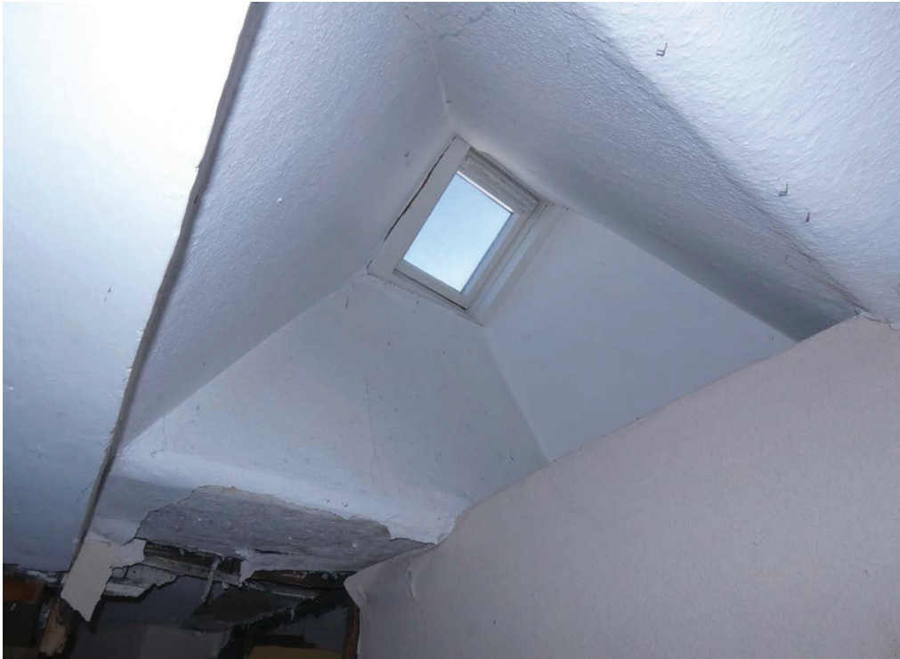
Plate 87: Skylight above F3
