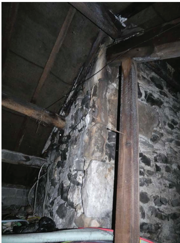
Plate 61: Quoins visible to the south-east in the roof space above G7
