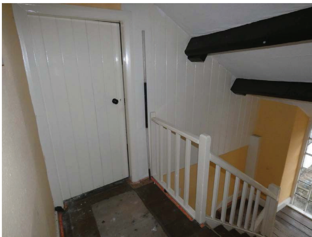
Plate 115: West elevation of S2
