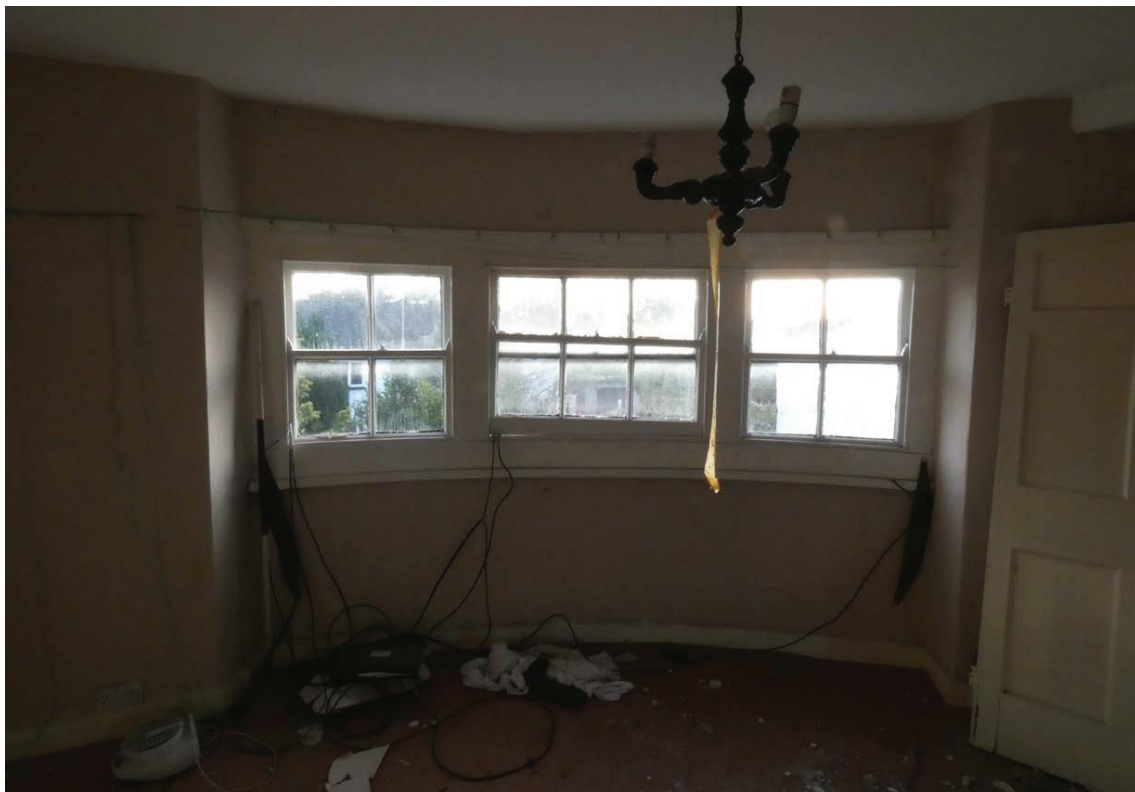
Plate 80: Window in the south elevation of F2
