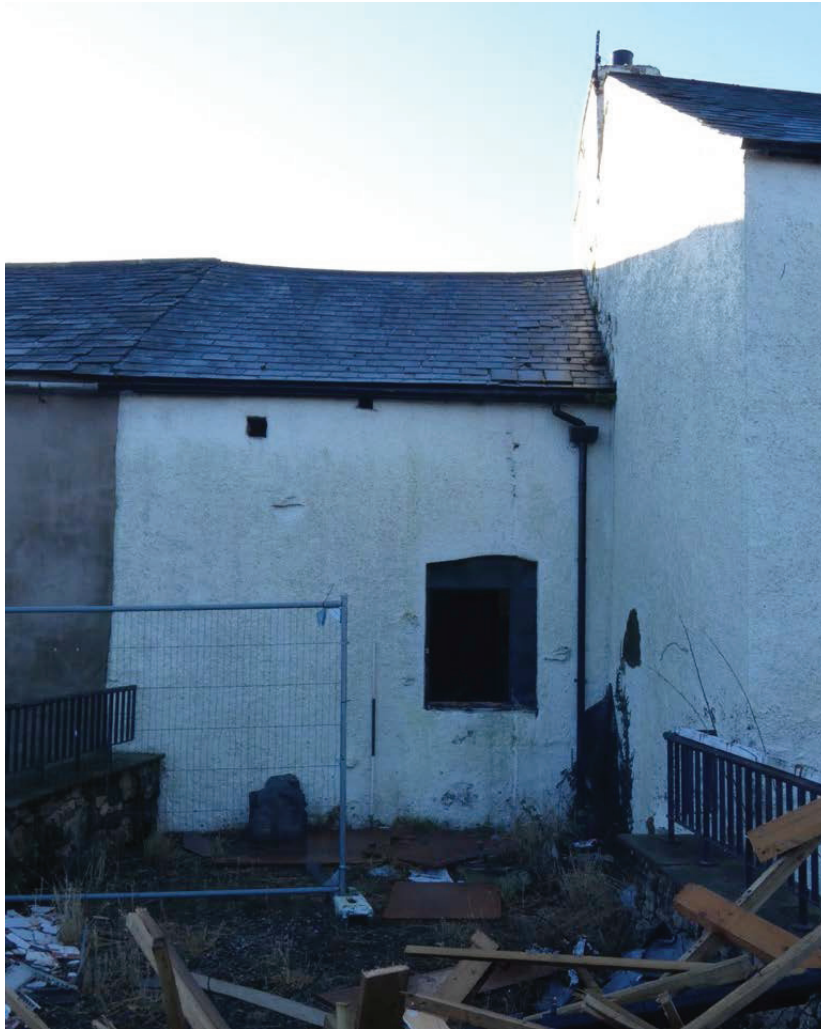
Plate 12: East end of the north external elevation
