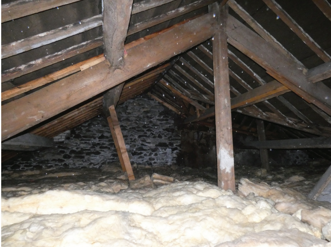
Plate 106: Truss above F2 and F3, viewed from the west
