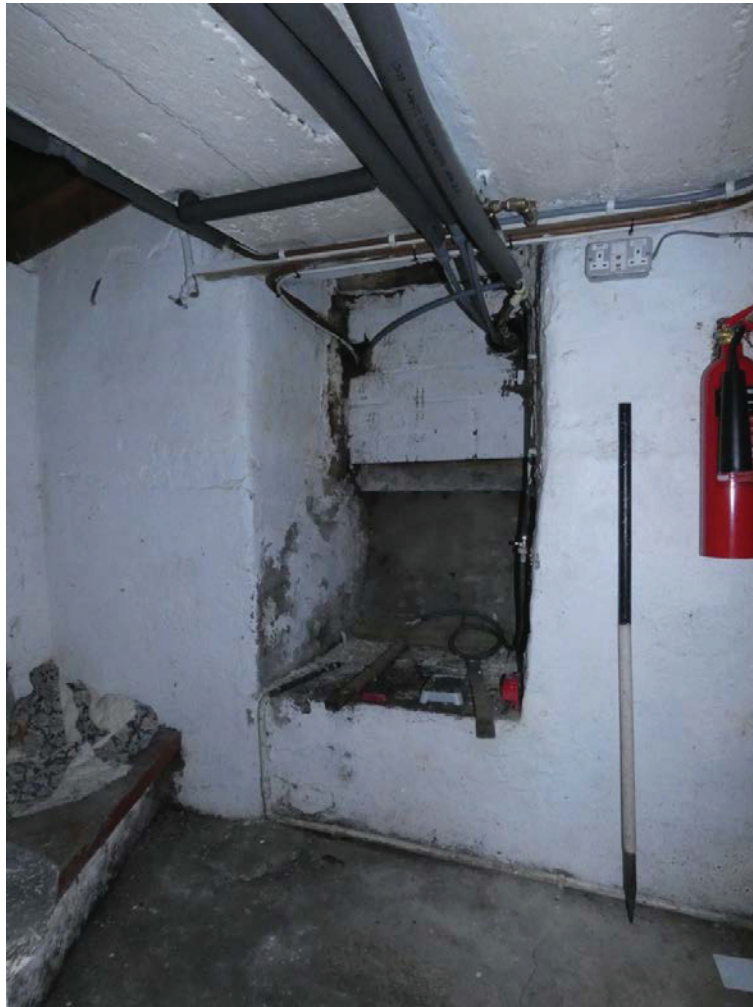
Plate 21: North elevation of B2
