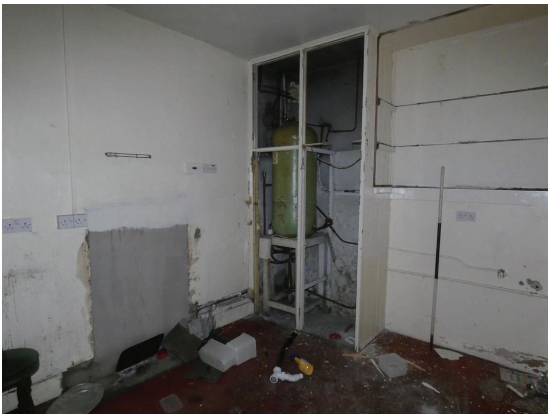
Plate 59: South end of the east elevation and south elevation of G7
