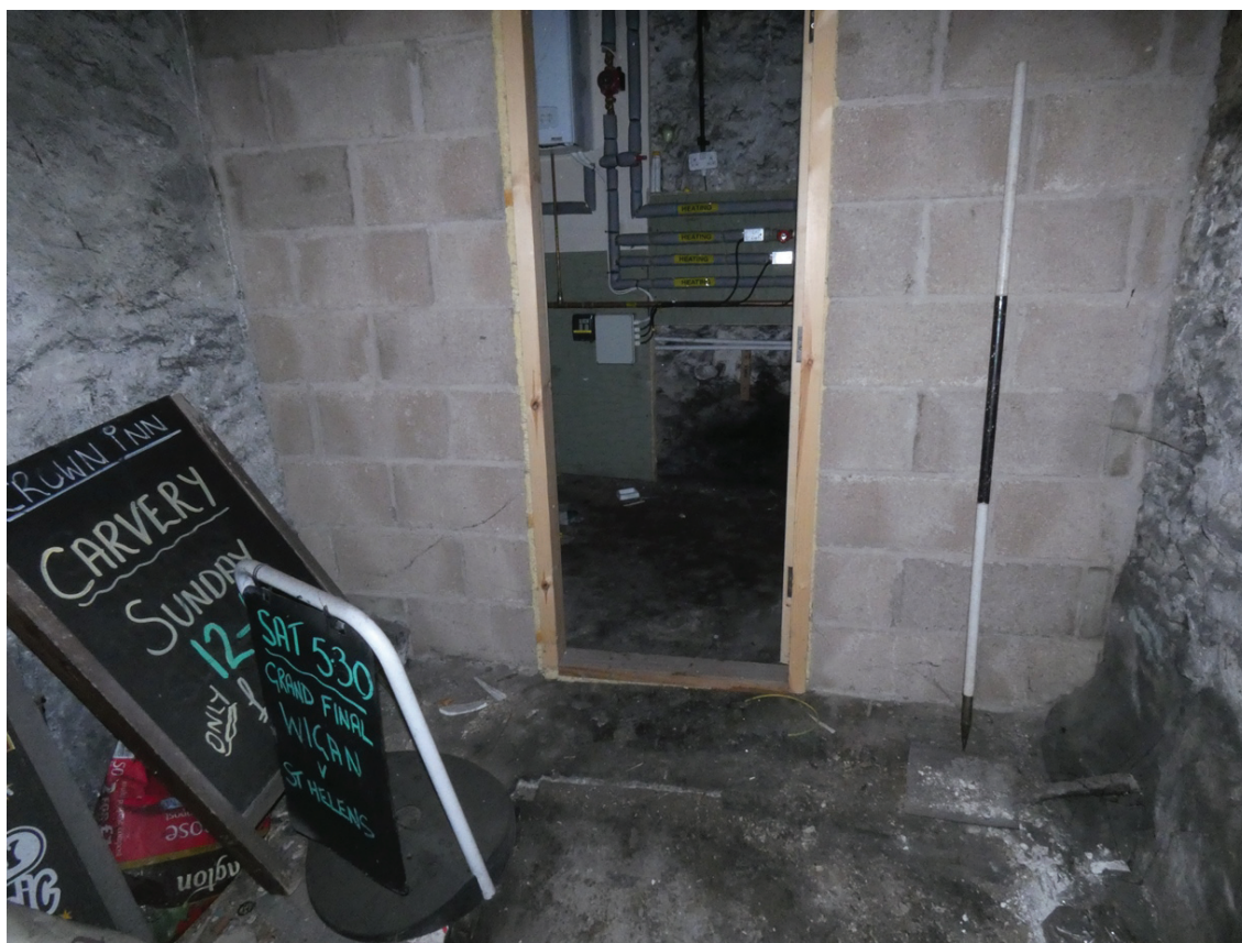
Plate 50: Partition wall in G6, viewed from the south side
