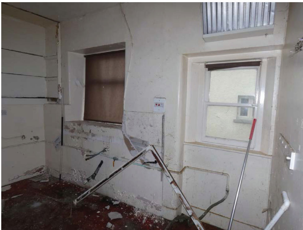
Plate 60: South end of the west elevation of G7
