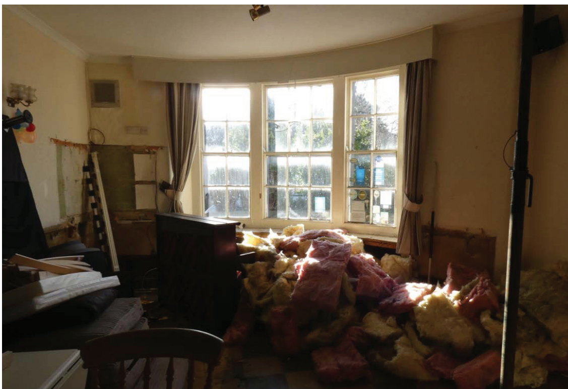
Plate 34: Window in the south elevation of G2
