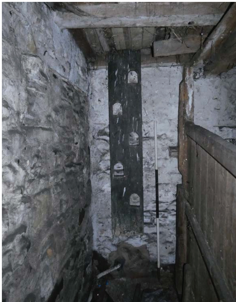
Plate 29: Ladder in the south-west corner of G1
