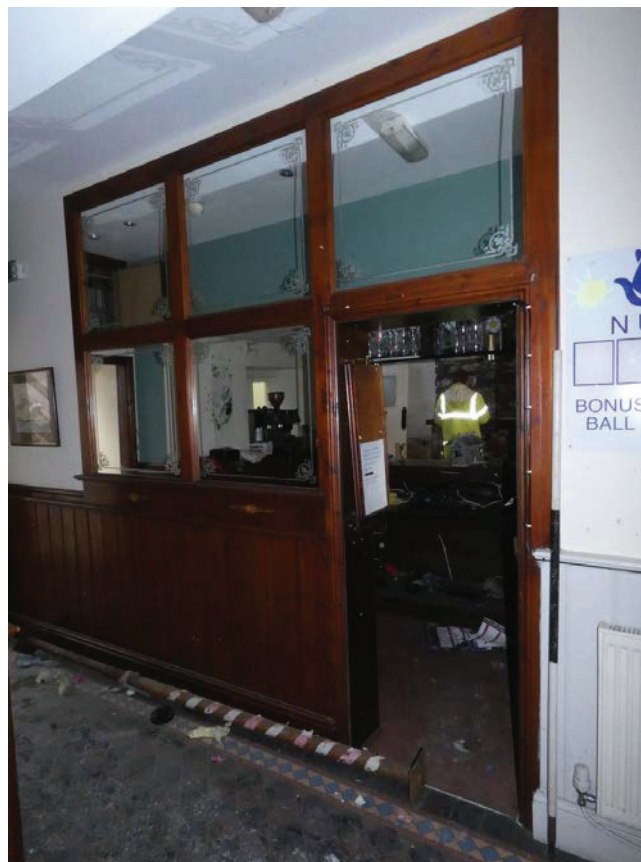
Plate 38: East elevation of G3
