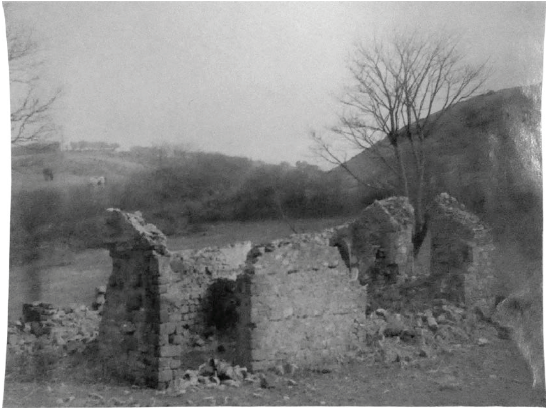
Plate 14: General view of the chapel from the south-west during or immediately after the removal of the windows (CAC(B) BAMH/2/53 1944-1957)
