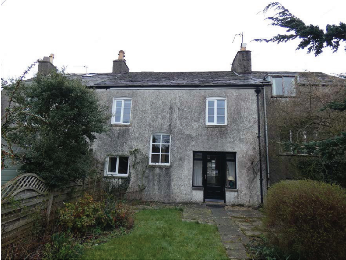
Plate 8: The west external elevation, viewed from the west
