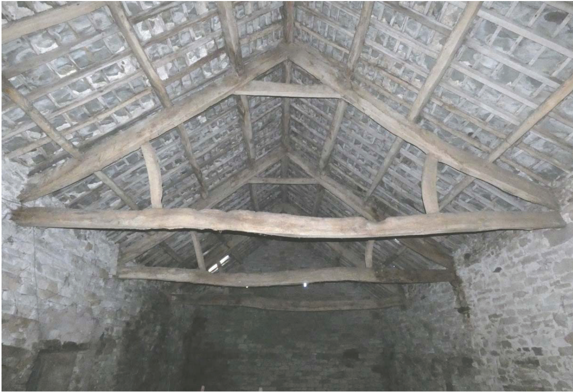
Plate 41: Trusses in Room U1, viewed from the north
