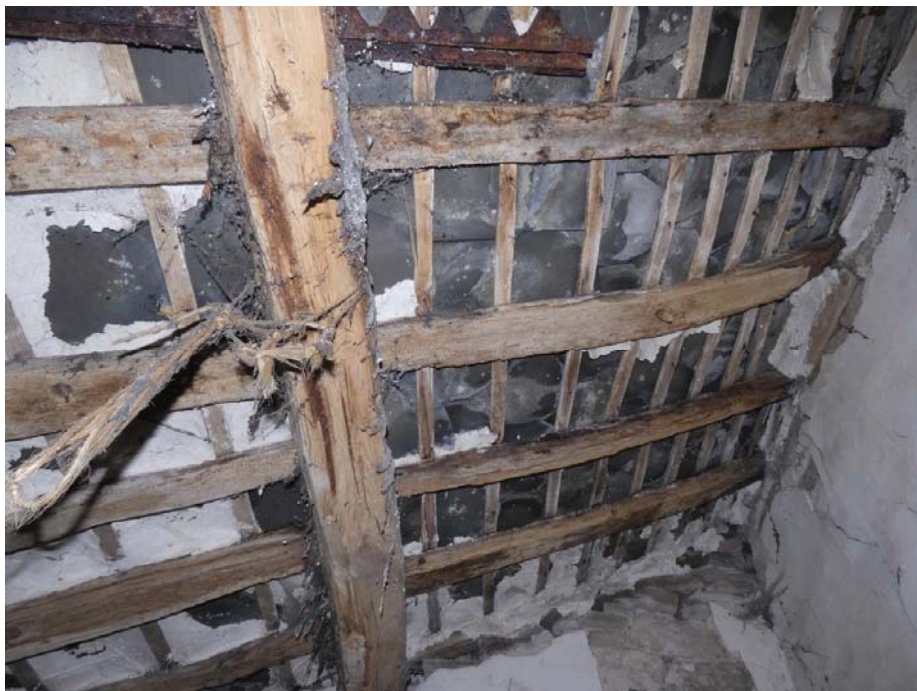
Plate 46: The roof in Room U2, viewed from the south
