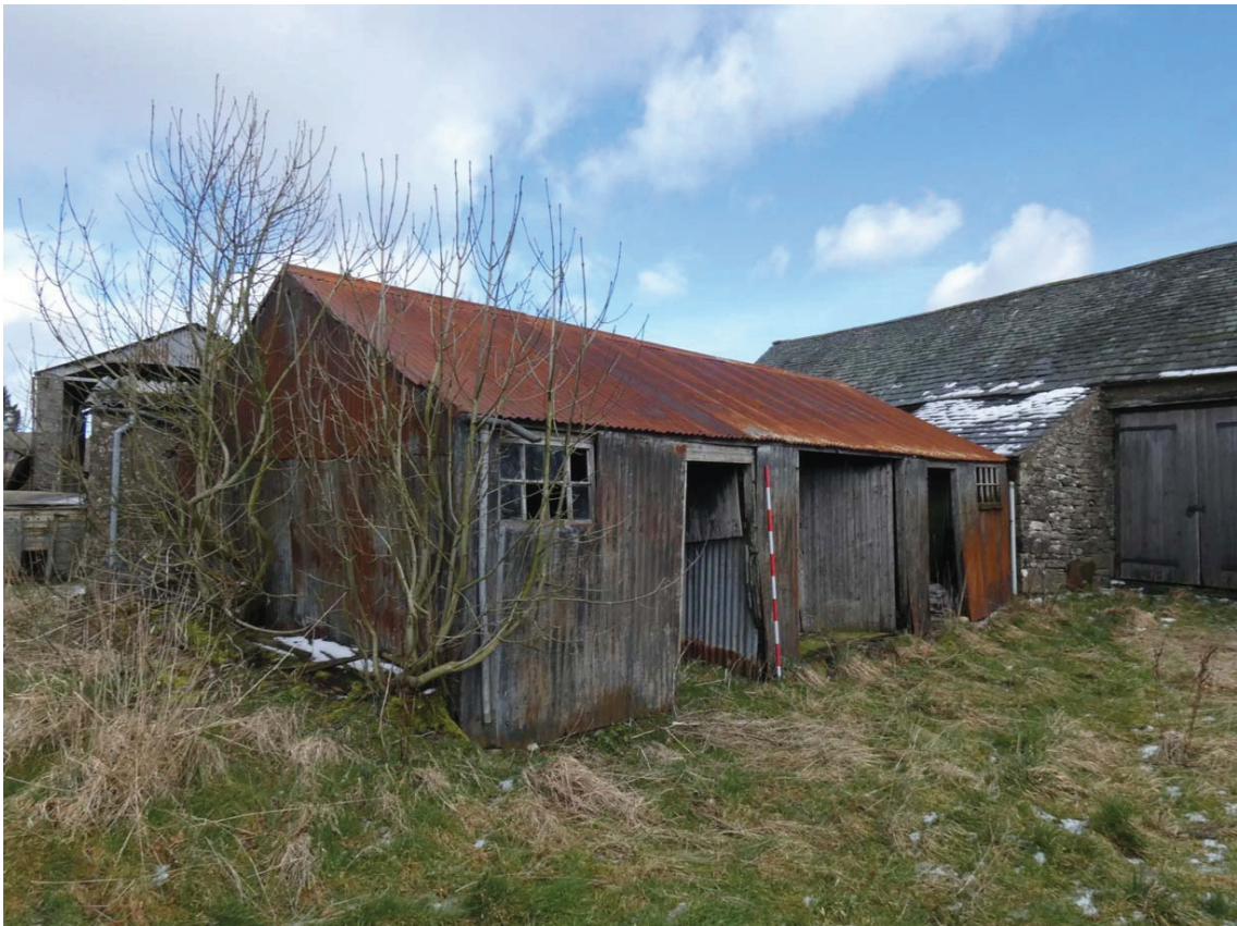
Plate 20: General view of the shed, from the south-west
