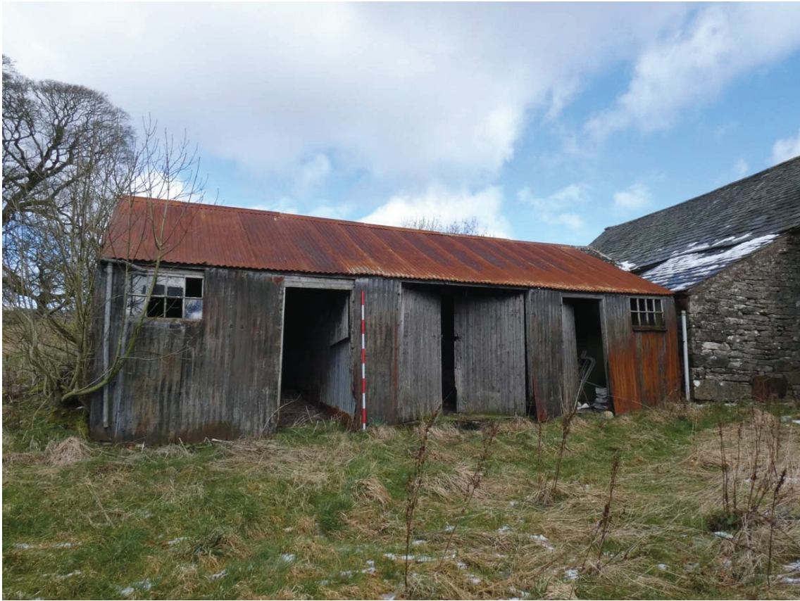
Plate 19: The south elevation of the shed, viewed from the south
