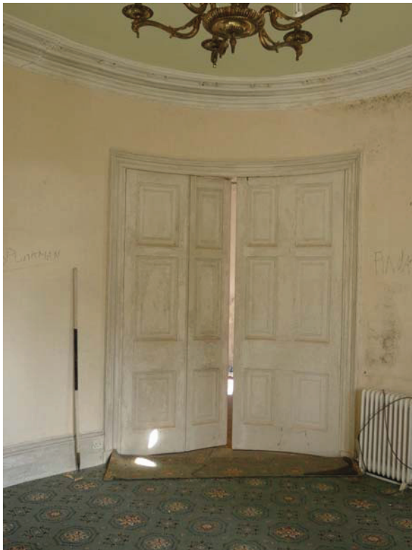
Plate 96 (left): Folding doors in the north-east elevation of Room G4, viewed from the south-west
