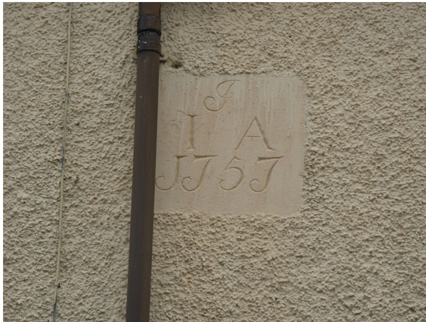
Plate 97: Datestone of 1757 on the west elevation of the cottages on Brewery Street
