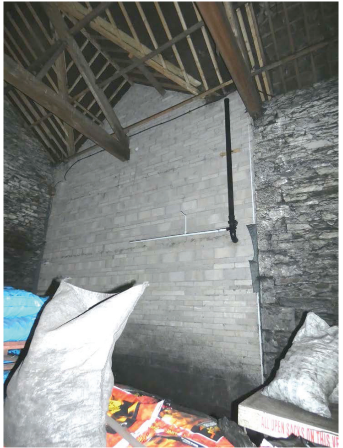
Plate 19 (left): Concrete ramp and associated block structure supporting the roof in the north-east corner, viewed from the south-west
