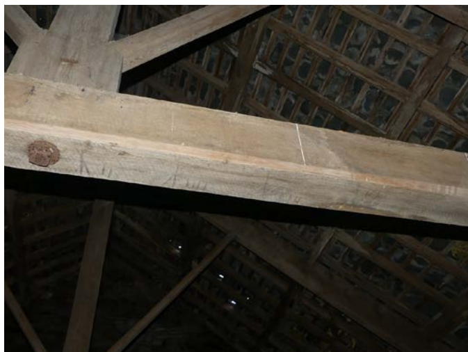
Plate 22 (left): Detail of Baltic marks on the central truss in upper ground floor Room 1, viewed from the north
