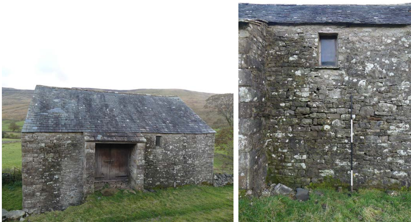
Plate 16 (left): West external elevation, viewed from the west
