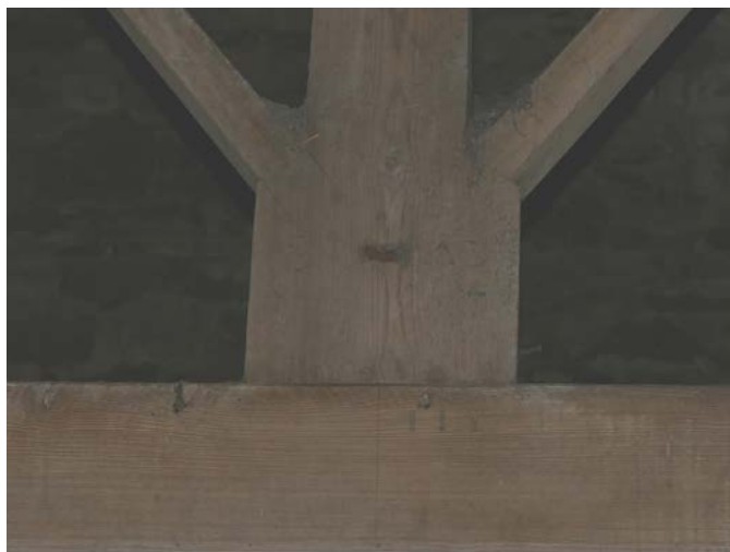
Plate 22 (left): Detail of Baltic marks on the central truss in upper ground floor Room 1, viewed from the north
