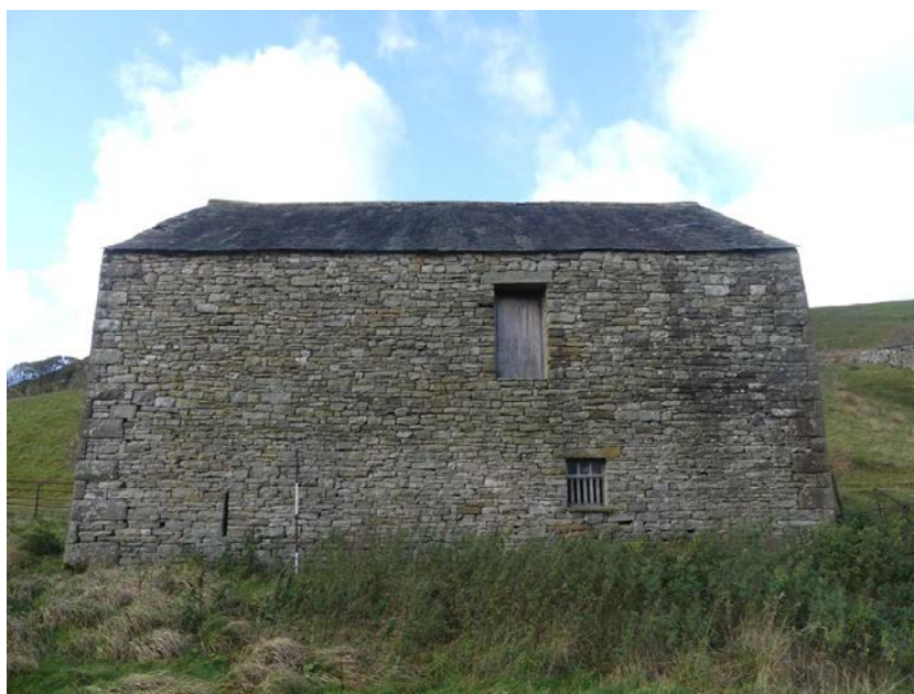
Plate 10: East external elevation, viewed from the east
