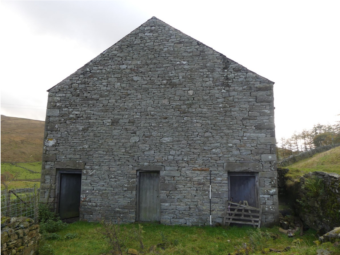
Plate 5: North external elevation, viewed from the north
