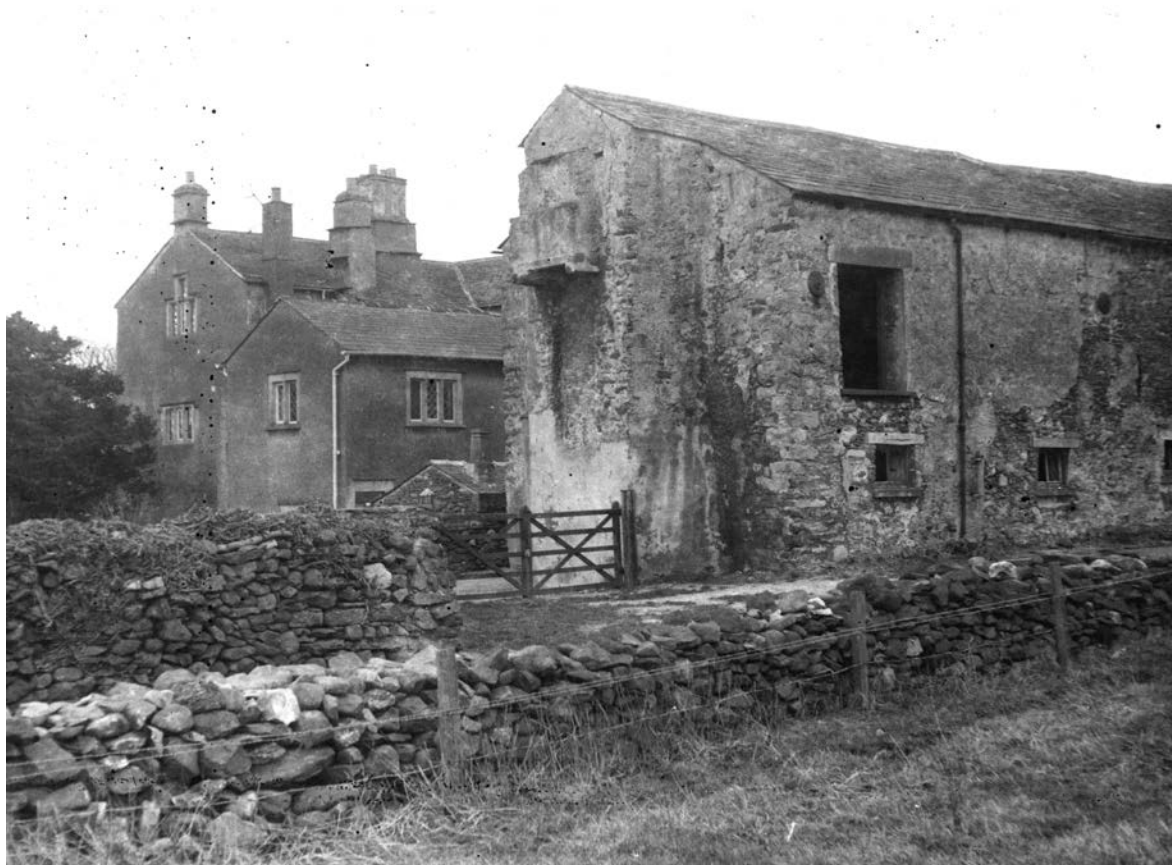
Plate 6: Mid 20 th century view of the north end with projecting chimney and corbled chimney stack
