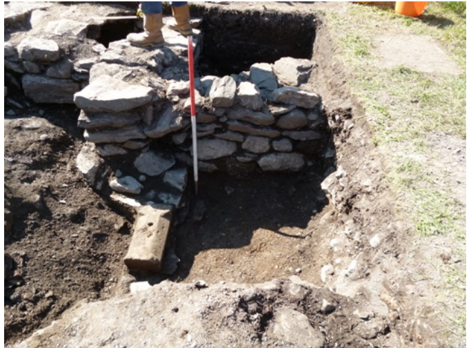
Plate 10 (right): Side elevation of wall 108 and sill for mullion window revealed in continuation of wall 109
