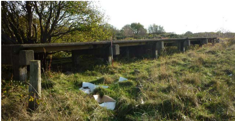
Plate 44: North view of the former platform
