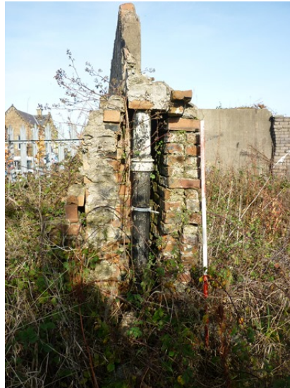
Plate 41: Cast concrete asbestos pipe
