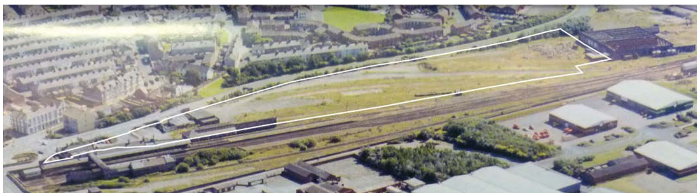
Plate 26: Extract from aerial photograph, 1999 (Byers 1999, 46), with the site boundary shown in the white
