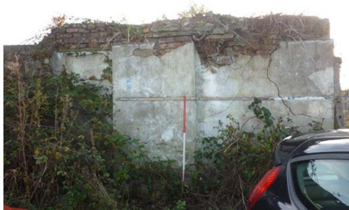
Plate 36: Plastered part at the west end of the central section
