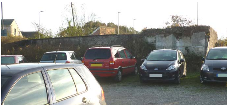
Plate 30: Central section and south-west end (visible in the sunshine to the right)
