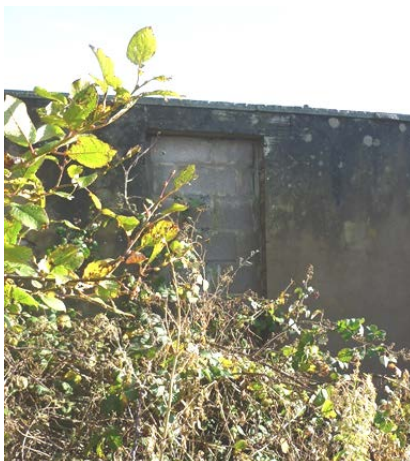
Plate 35: Recess in the north-west end section formed by the blocked door
