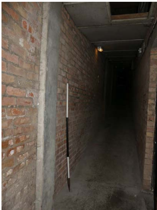
Plate 18: The south external elevation, inside the passageway, viewed from the west
