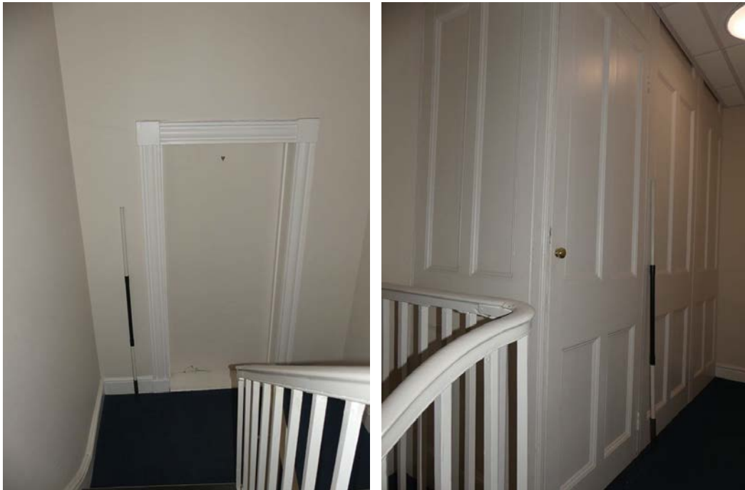
Plate 64 (left): Former window in the west elevation of Room S2, viewed from the east
