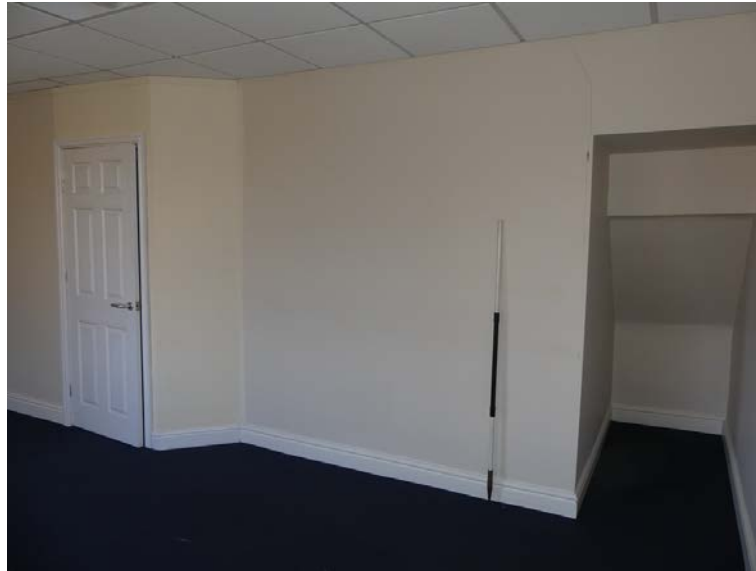
Plate 68: West side of Room S4, viewed from the north-east
