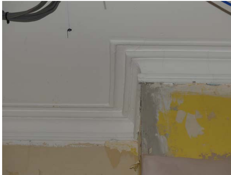
Plate 88: Cornice exposed in Room F3, viewed from the north
