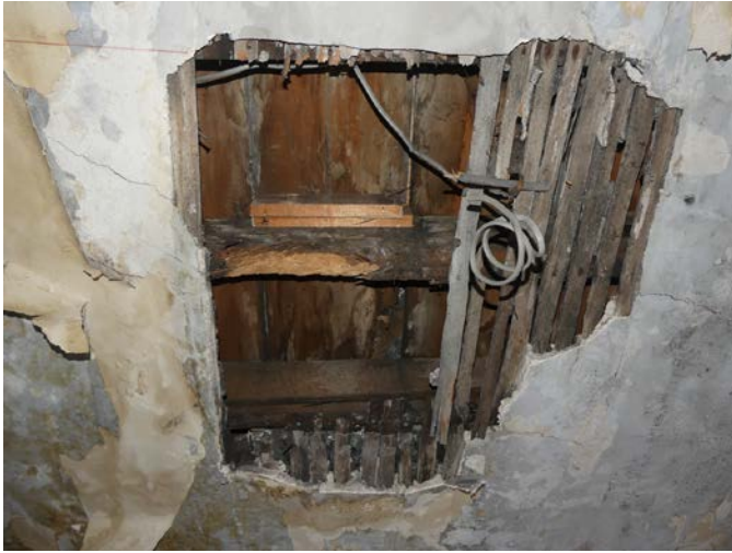
Plate 95 (left) Exposed joists and boards behind the lathe and plaster exposed in Room S1, viewed from the west
