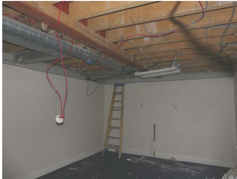
Plate 74: View of Room LG1 following soft stripping, viewed from the north-east
