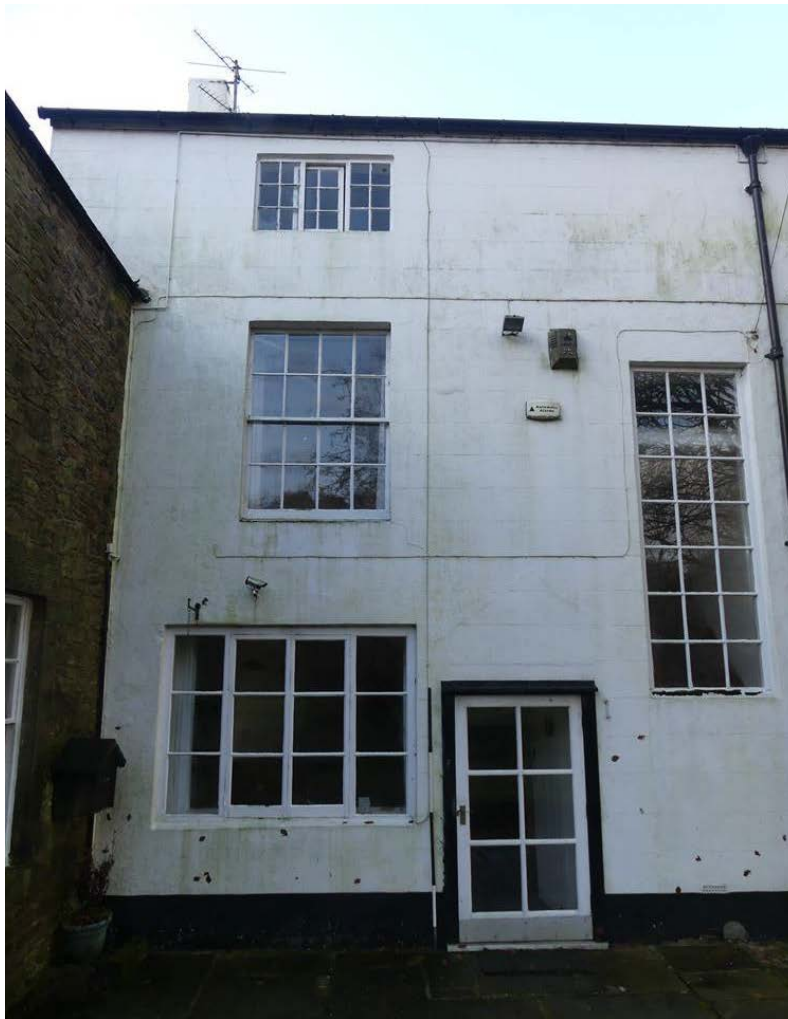
Plate 24 (right): North-east external elevation of the main house
