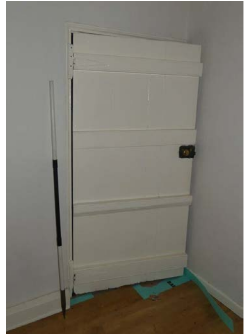
Plate 161 (right): Door in the south-west elevation of Room S5
