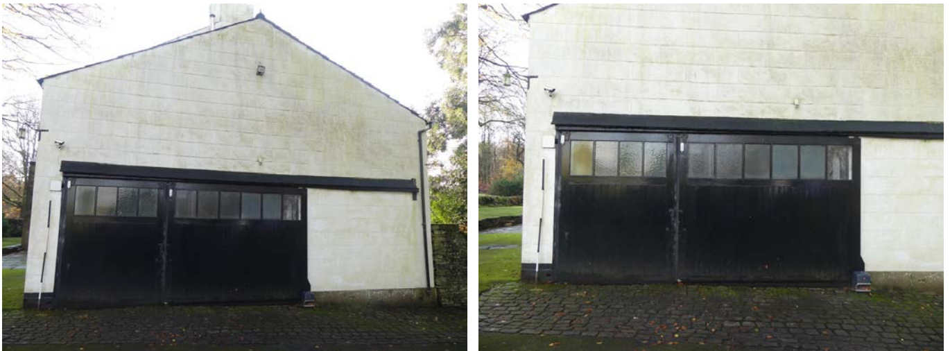
Plate 19 (left): North-west external elevation of the garage
