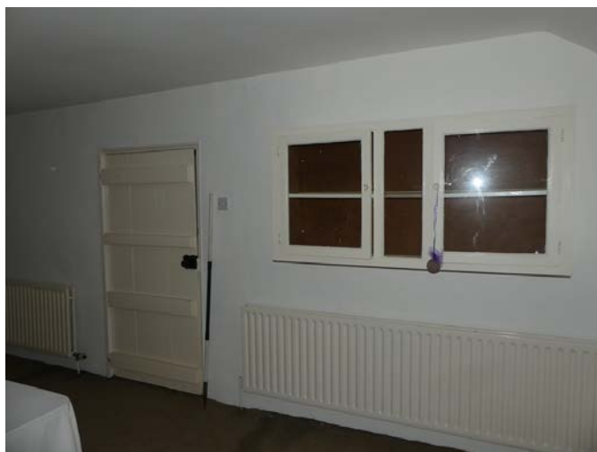
Plate 148: North-west elevation of Room S1
