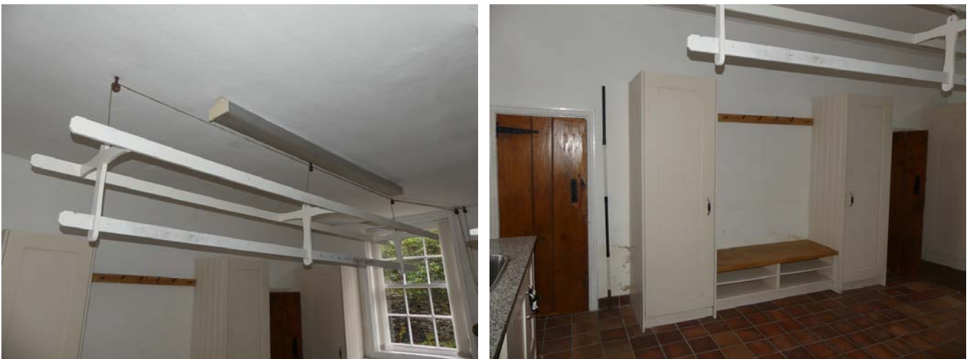
Plate 44 (left): Hanging timber drying rack in Room G1
