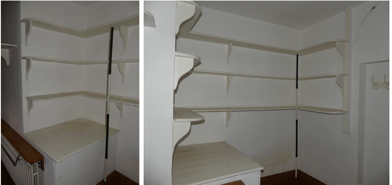
Plate 94 (left): Boxed section over the stairs in Room G7
