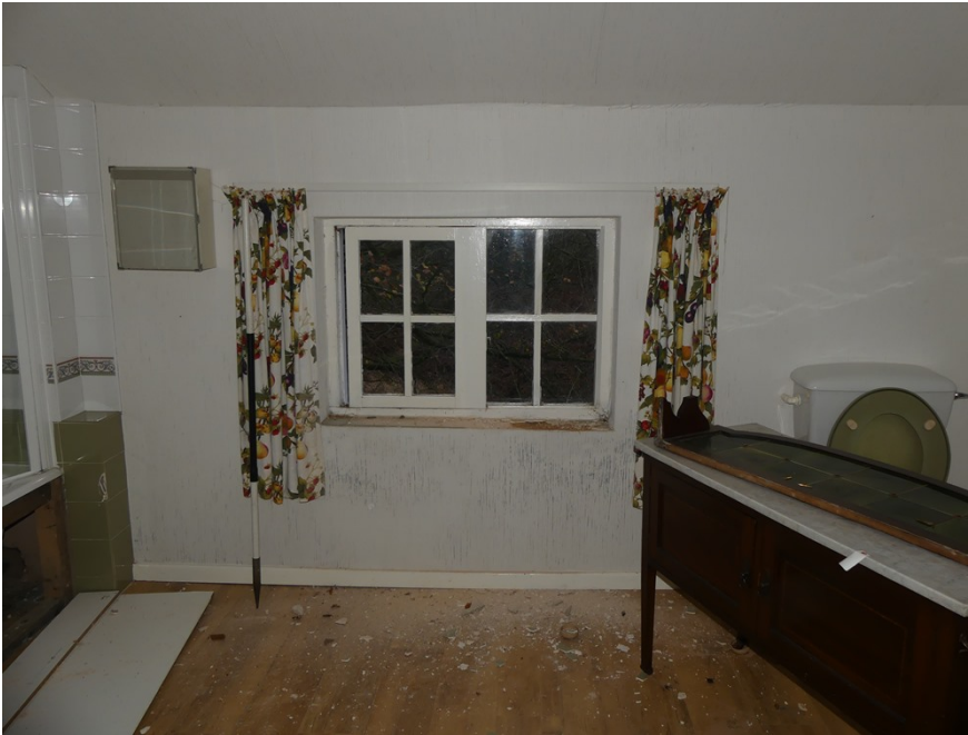
Plate 160 (left): North-east elevation of Room S5
