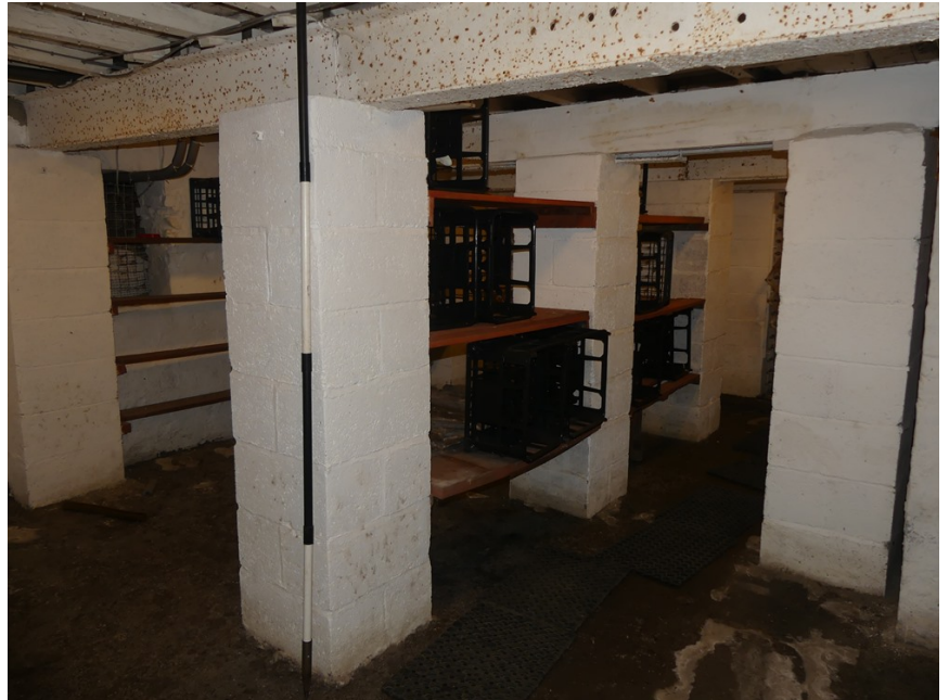
Plate 34 (left): I-beam supports in the basement
