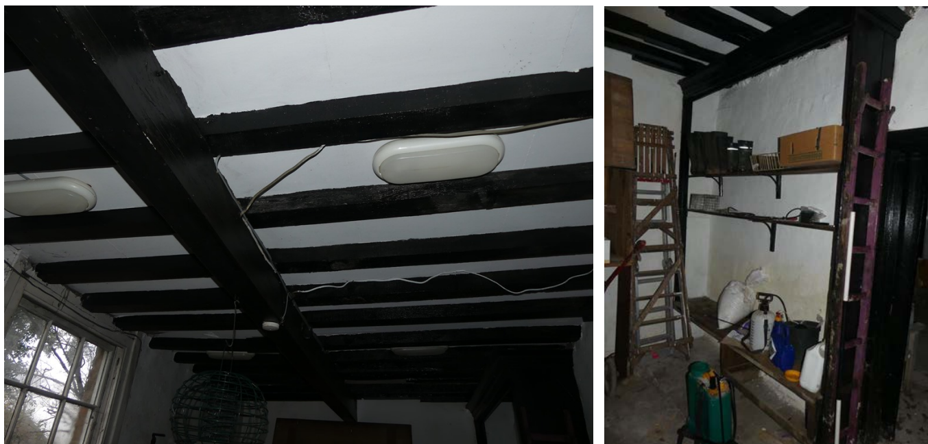
Plate 108 (left): Ceiling in Room G9
