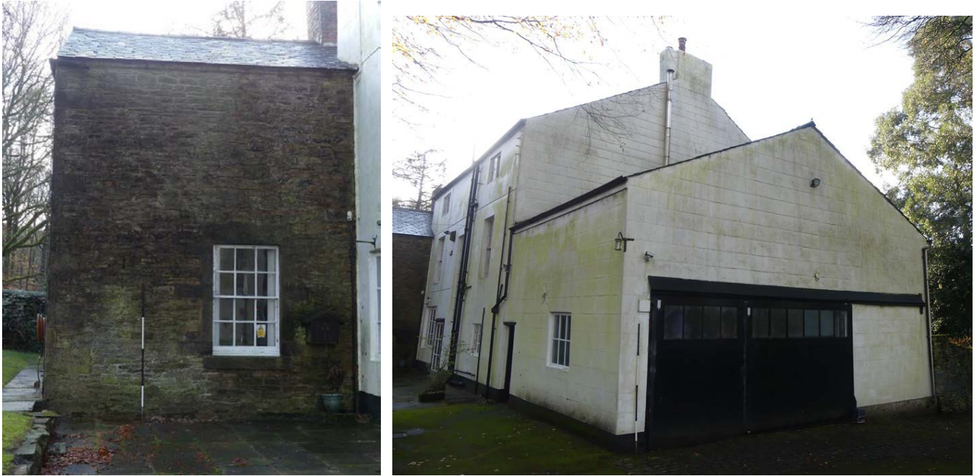
Plate 17 (left): North-west external elevation of the south-east extension
