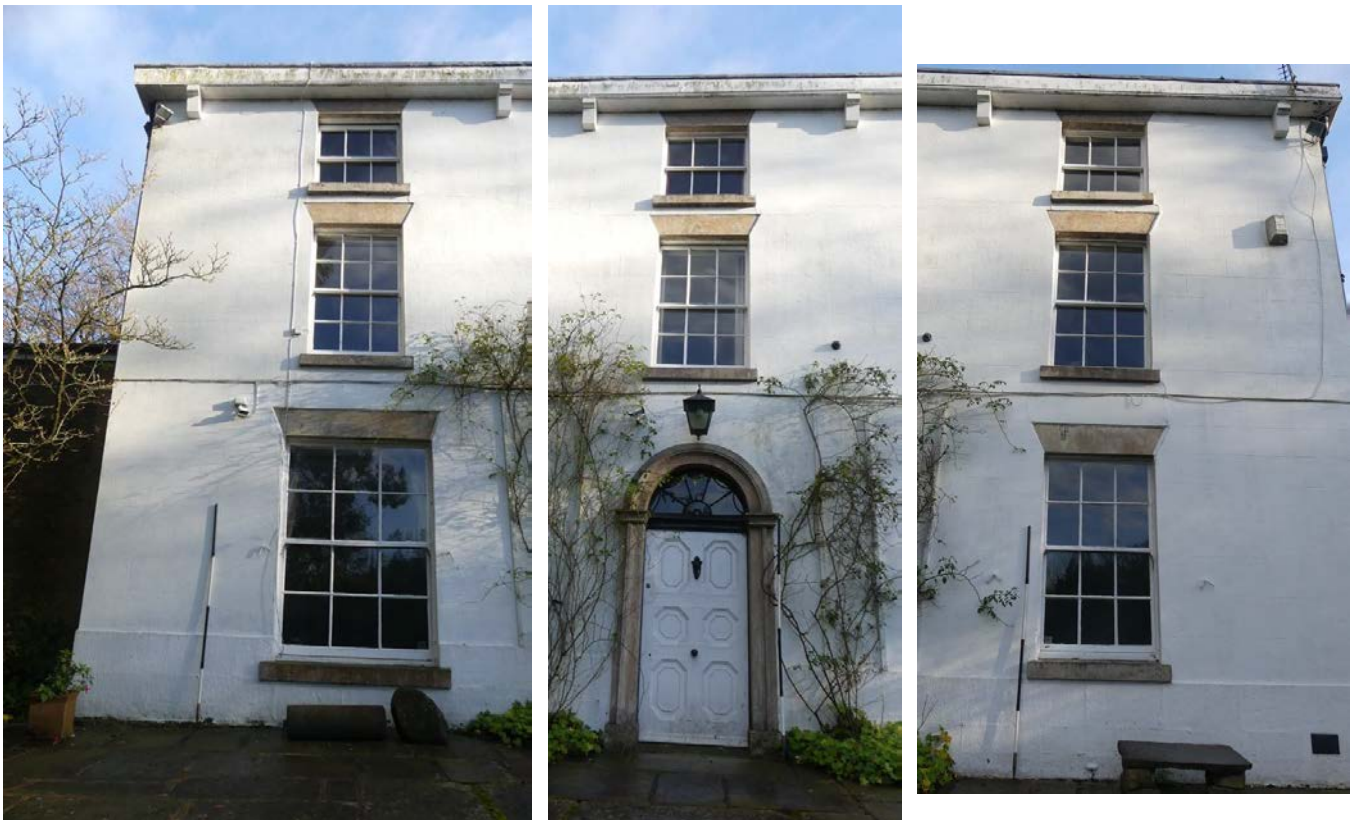
Plate 11 (left): North-west end of the south-west external elevation of the main house Plate 12 (centre): Central part of the south-west external elevation of the main house Plate 13 (right): South-east end of the south-west external elevation of the main house
