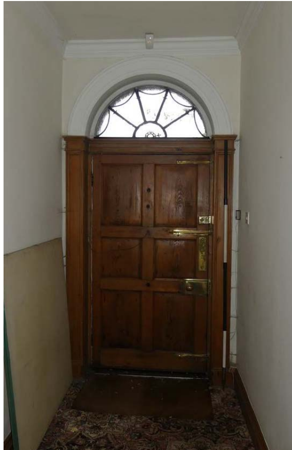
Plate 83: Door at the south-west end of Room G5
