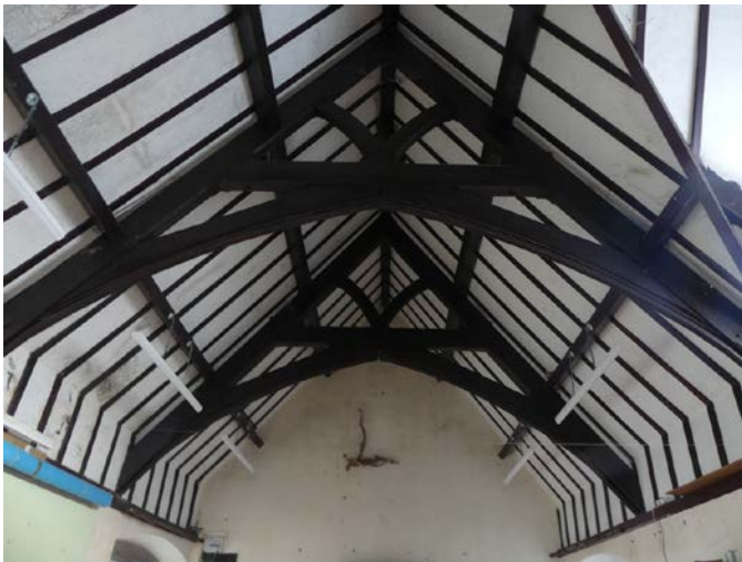
Plate 24 (left): Trusses at the north end of Room G1, viewed from the south
