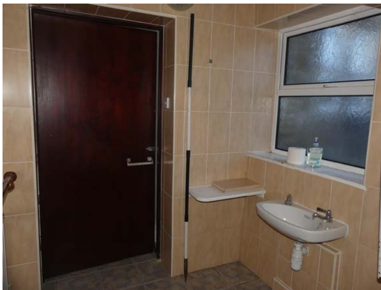
Plate 36: The north and west sides of Room G4, viewed from the south-east
