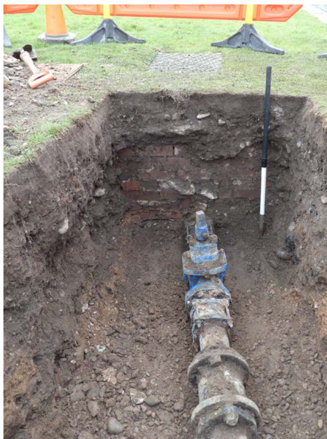
Plate 6: Brick in section forming the side of the inspection chamber to the south-east of the trench, viewed from the north-west
