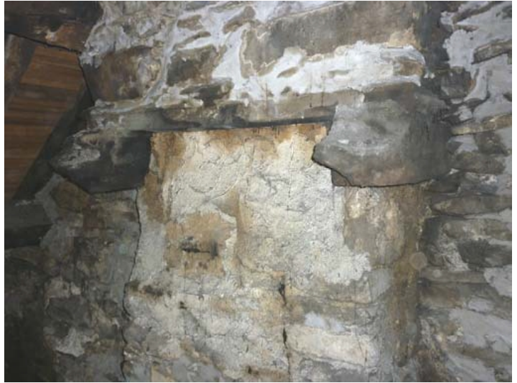
Plate 102 (left): Chimney breast in the roof space above F2
