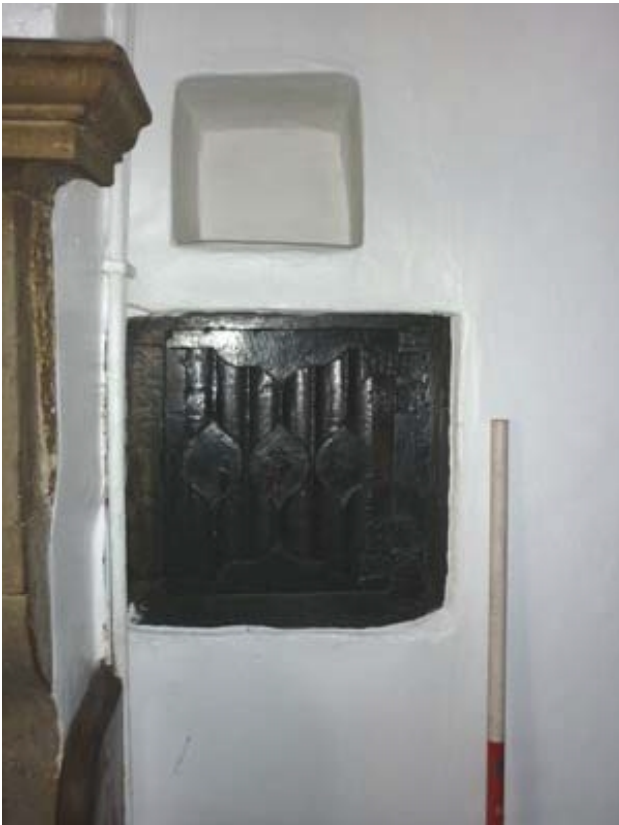
Plate 61 (left): Spice cupboard door and alcove above in the south-west elevation
