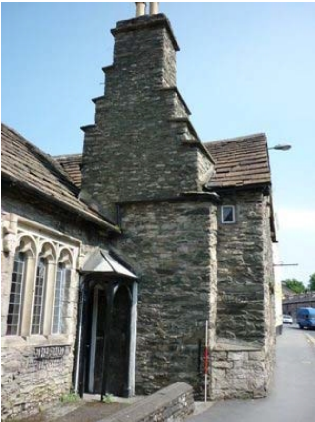
Plate 33 (left): Return at north-east end with projecting chimney stack
