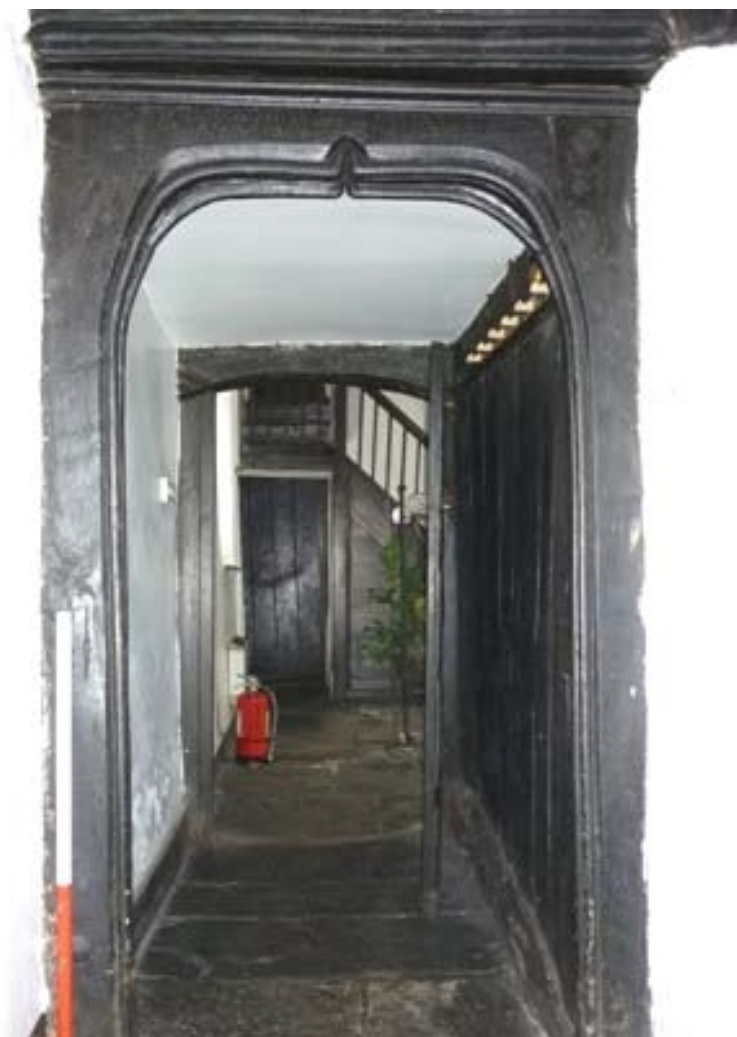
Plate 67: Moulded doorway in the north-east elevation
