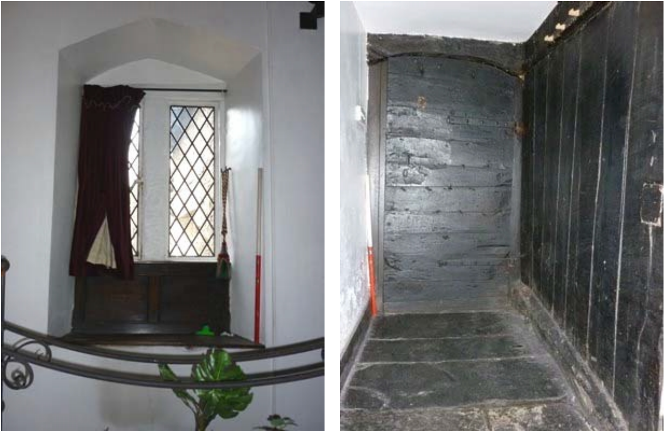
Plate 65 (left): Window in the north-west elevation
