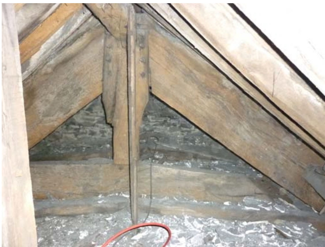
Plate 105: Modified truss in the roof space above F1
