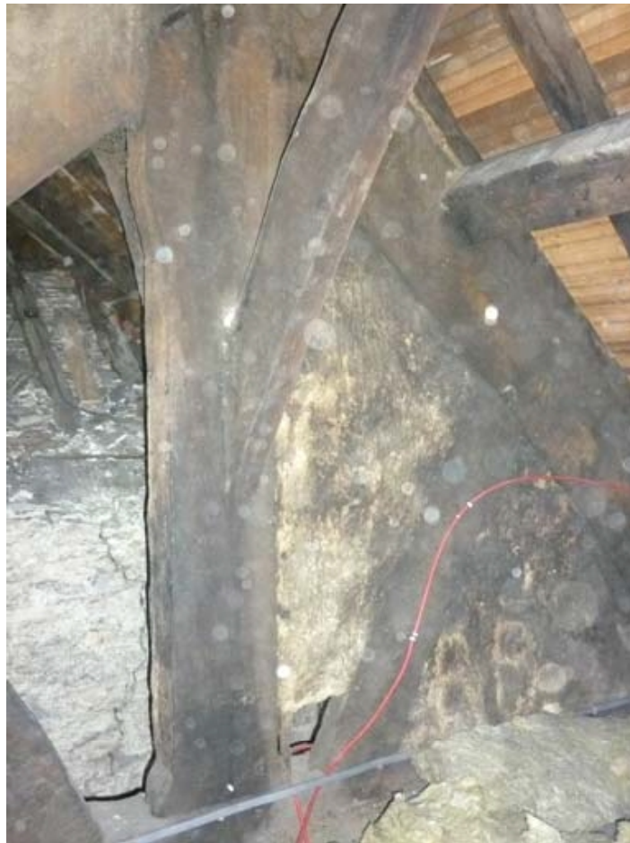
Plate 101: North-east truss in the roof space above F2 with wattle and daub infill
