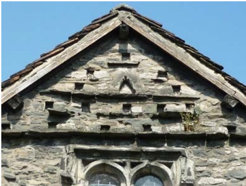
Plate 32: Top of the gable of the north-east wing
