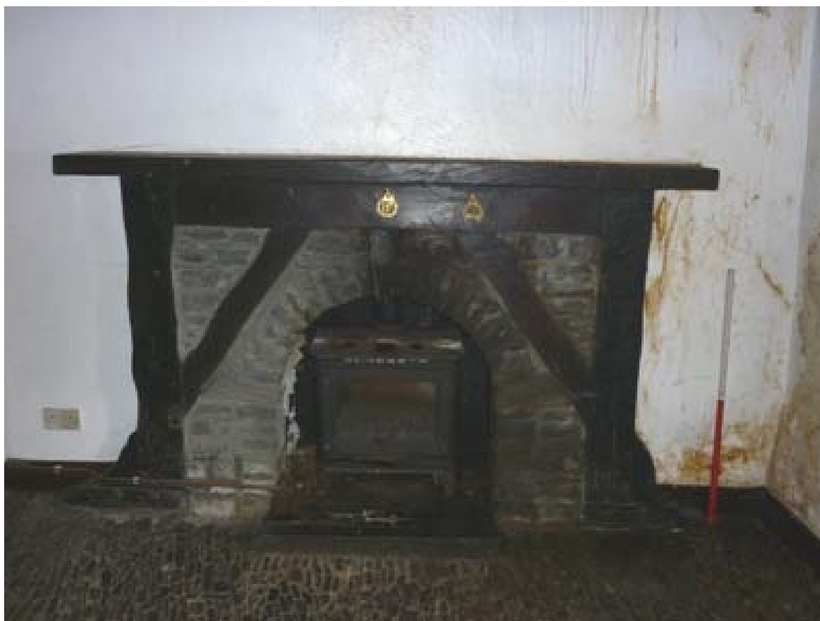
Plate 76: Modern fireplace in the north-east elevation
