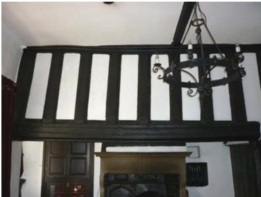
Plate 58: Screen above the bressumer beam at the south-west end of the room
