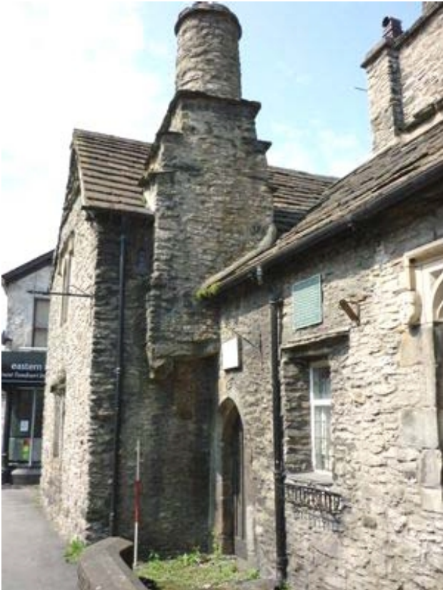
Plate 37 (left): Return at south-west end with projecting chimneystack at first floor level
