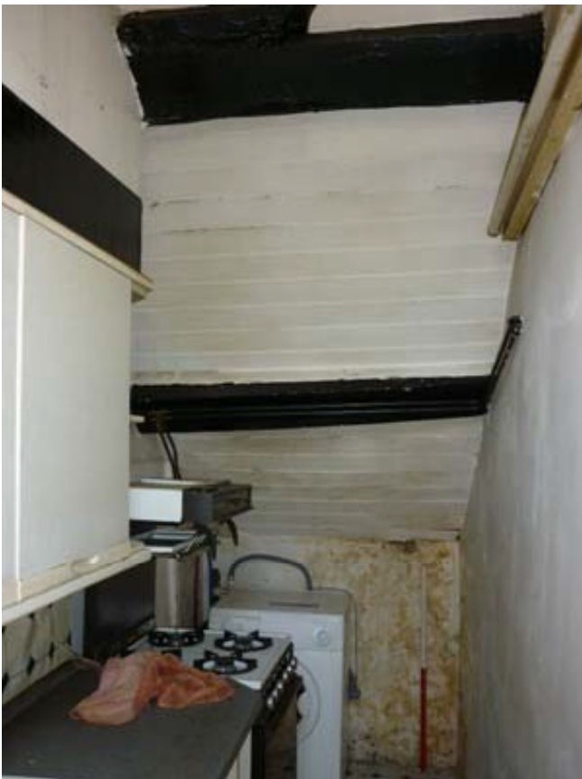
Plate 99 (left): Purlins on the south-east side of the room
