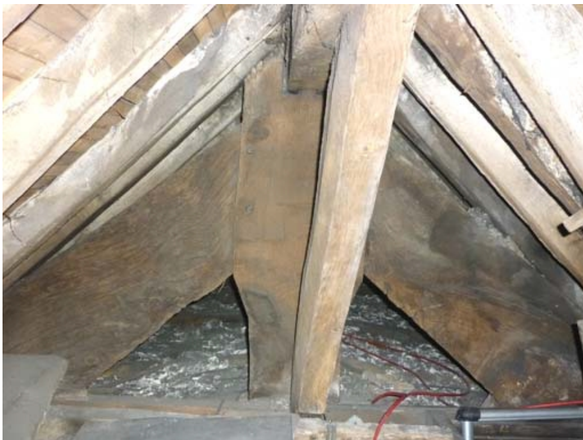
Plate 104: Top of the truss in the roof space above F2
