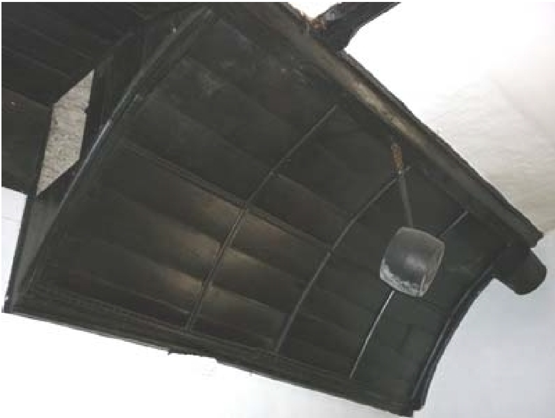
Plate 53: Barrel vaulted panelling against the north-east elevation
