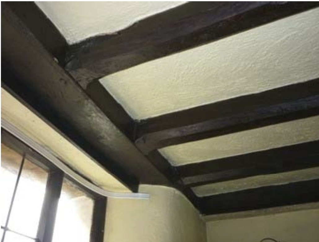
Plate 80: General view of the ceiling
