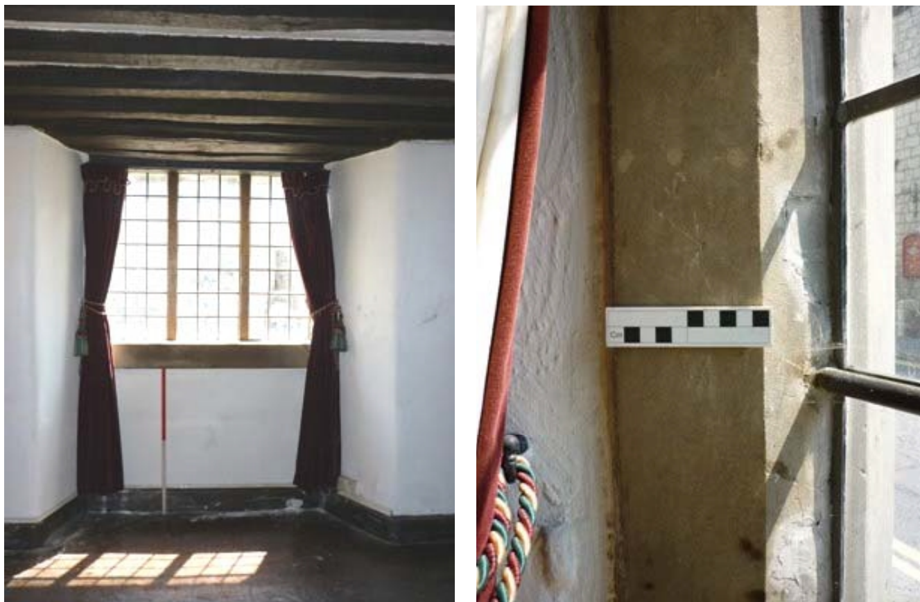
Plate 49 (left): Window in the south-east elevation
