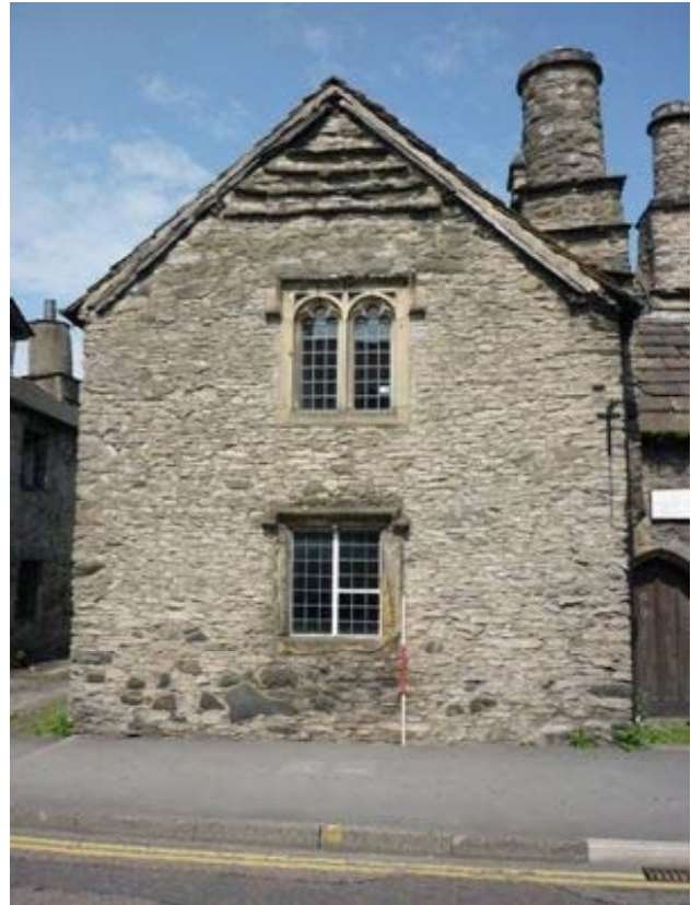
Plate 37 (left): Return at south-west end with projecting chimneystack at first floor level
