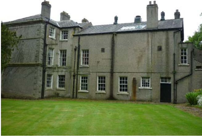
Plate 30 (left): Site 20 – general view of north elevation
