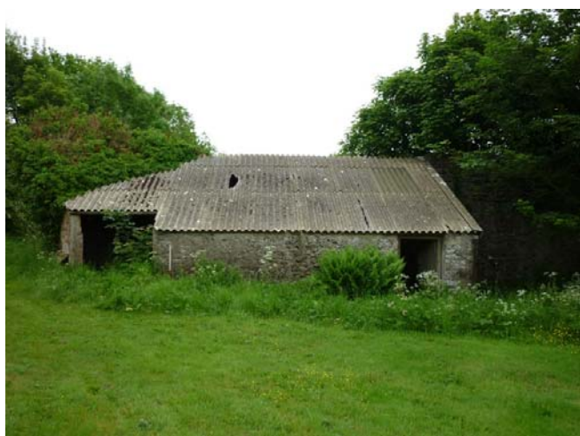
Plate 18 (left): Site 08 - external view from the north
