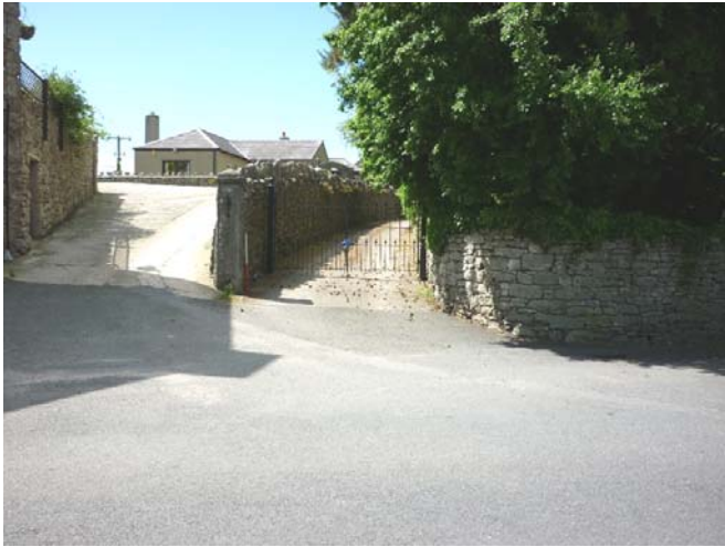
Plate 36: Site 22 - general view from east
