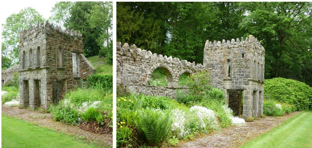
Plate 28 (left): Site 19 – general view from north-east
