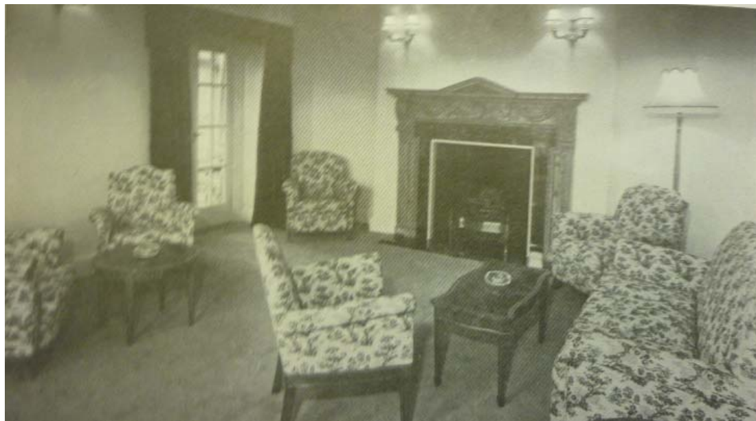
Plate 14: Interior view showing an elaborate fireplace in the lounge (after Melville 1959)
