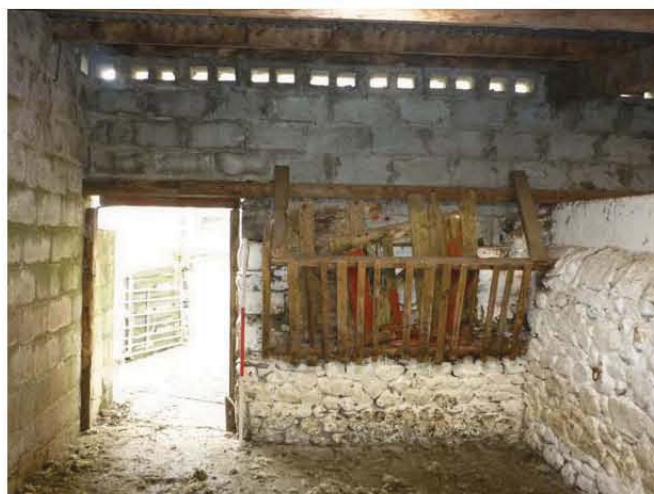
Plate 101: West elevation of Room 4 of the east outbuilding
