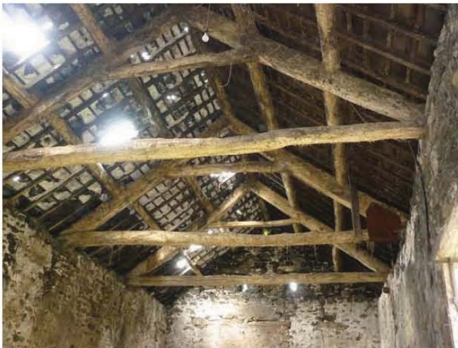
Plate 68: Roof structure of upper floor Room 1 of the barns
