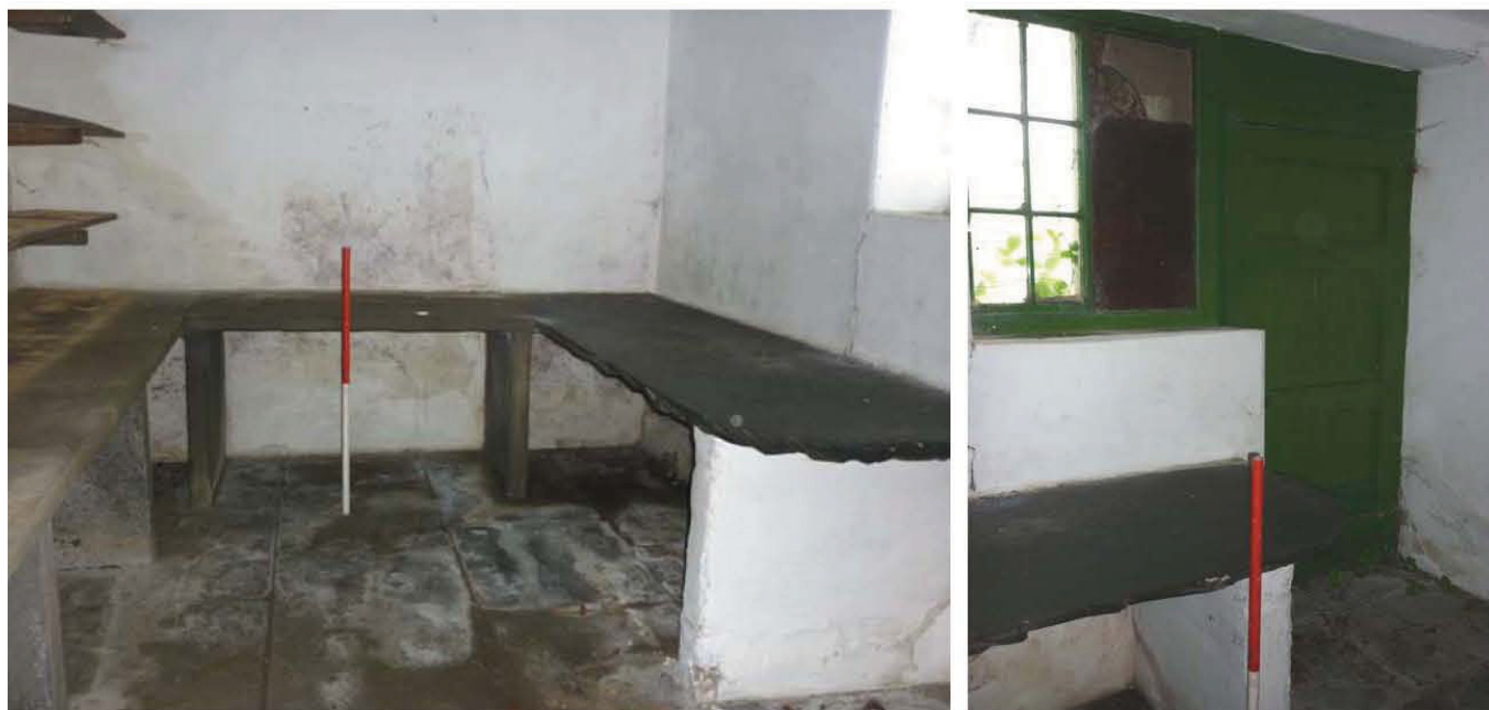
Plate 50 (left): Stone benches around the walls of ground floor Room 7 of the farmhouse
