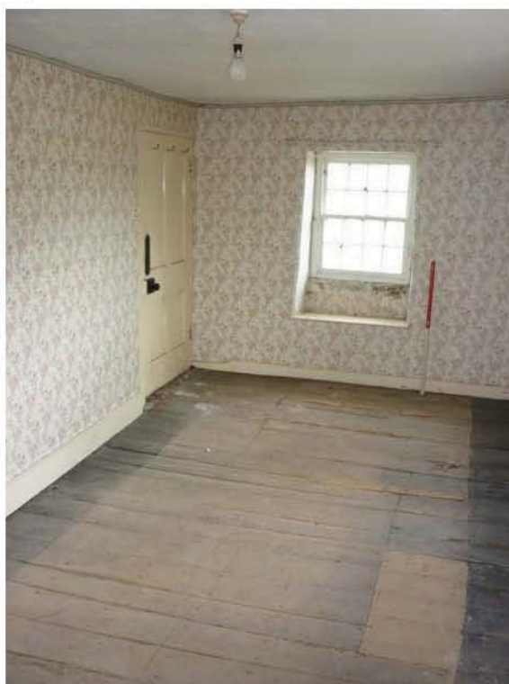
Plate 52: North-west corner of first floor Room 1 of the farmhouse
