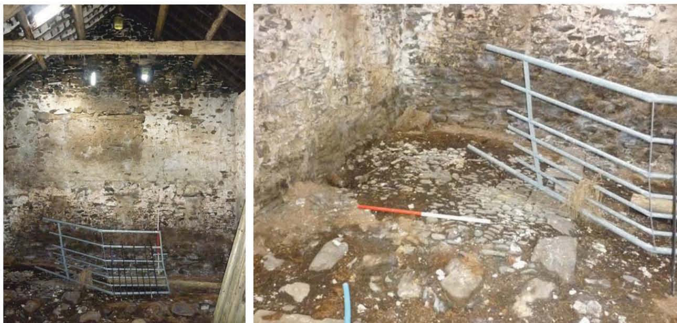
Plate 74 (left): West elevation of upper floor Room 1 of the barns
