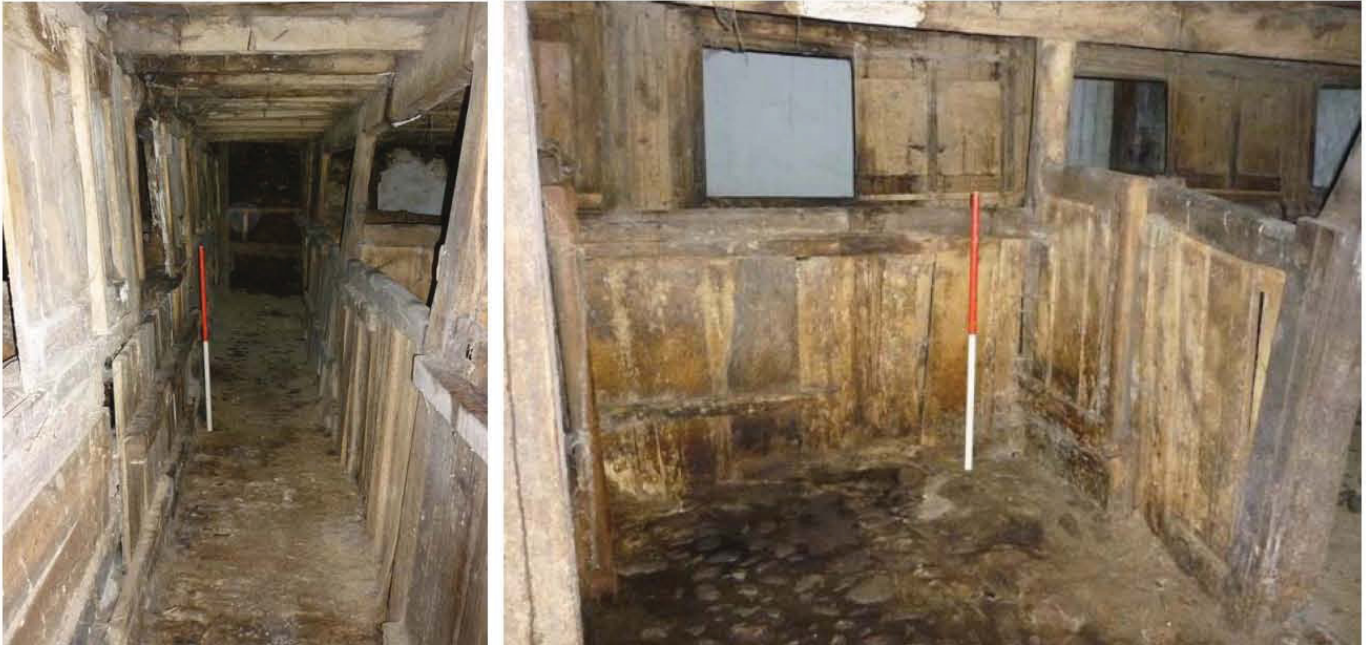
Plate 90 (left): Feeding passage between the rows of stalls in lower floor Room 3 of the barns
