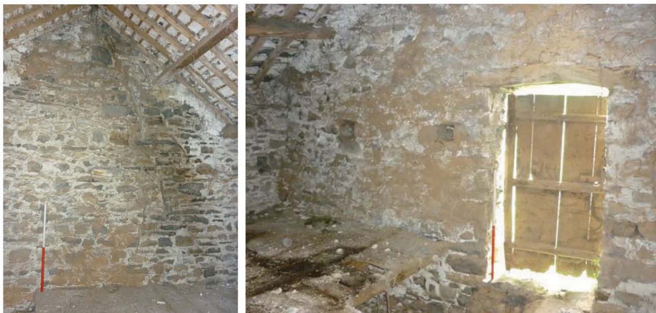
Plate 61 (left): East elevation of first floor Room 8 of the farmhouse
