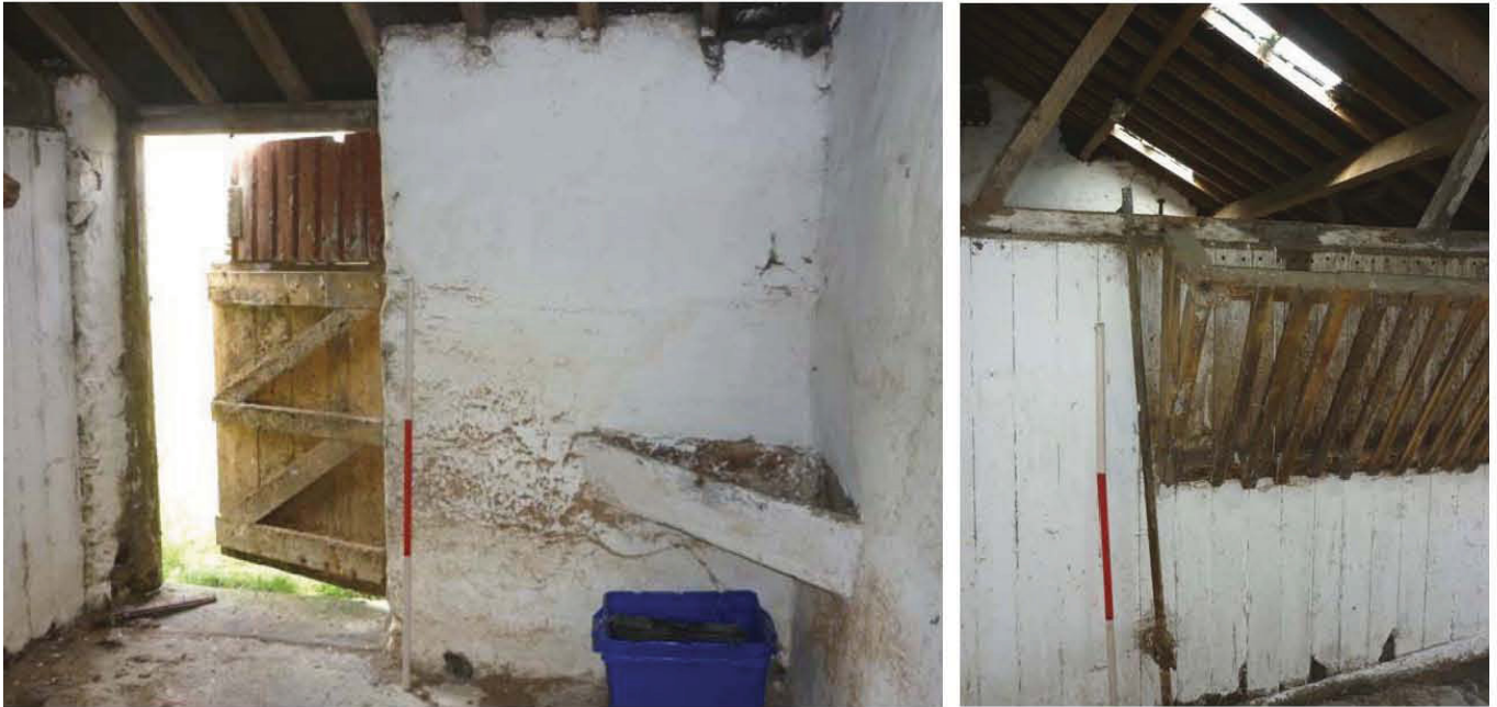
Plate 76 (left): North elevation of upper floor Room 3a of the barns
