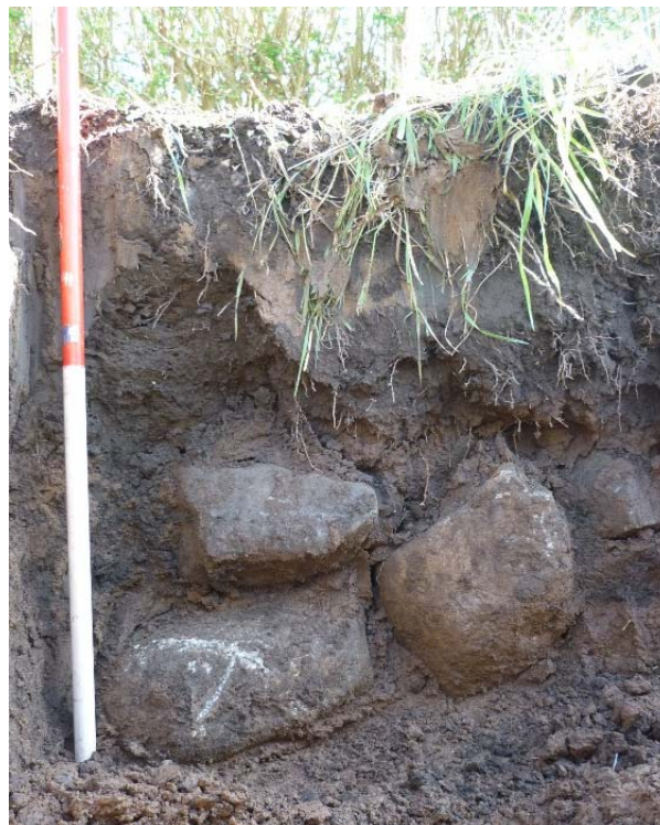
Plate 9 (above left): Excavation of the footings
