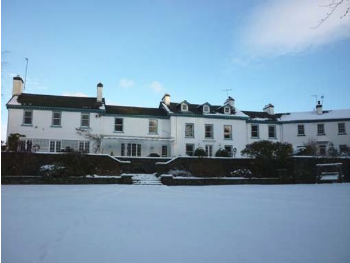
Plate 33: General view of the south external elevation of the house, with the veranda left of centre
