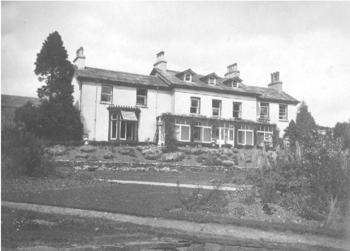
Plate 8: Photograph of the south elevation of the house dated 1923-1925
