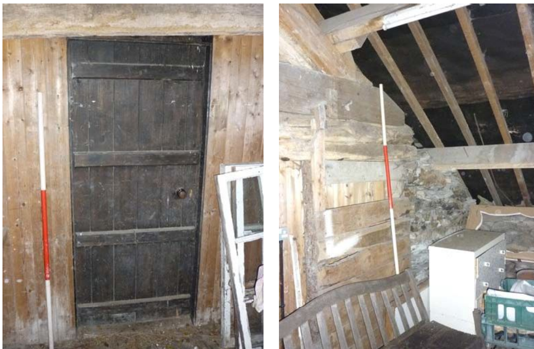
Plate 29 (left): Doorway to south-west, upper floor Room 2
