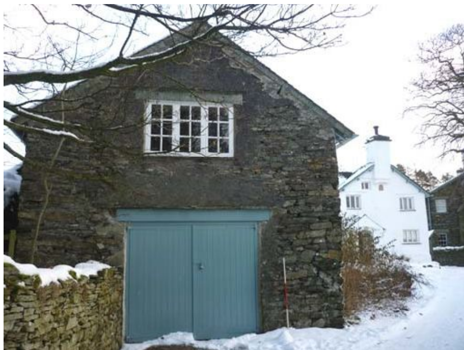
Plate 15: South-west external elevation, with The Cottage in the background
