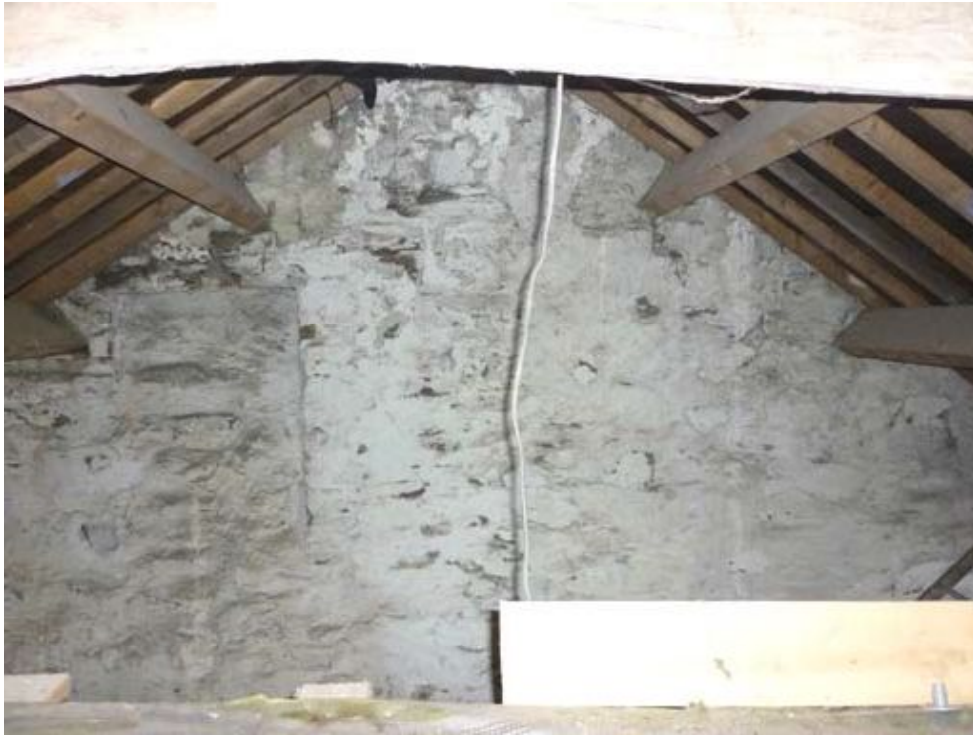
Plate 17: Upper part of the north-east elevation showing the blocked apertures
