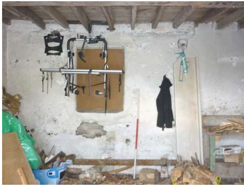
Plate 20: Window in the north-west elevation, lower floor Room 2
