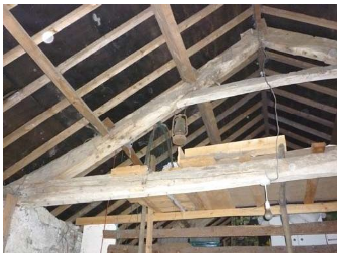
Plate 25 (left): Typical truss, north-east end of upper floor Room 1
