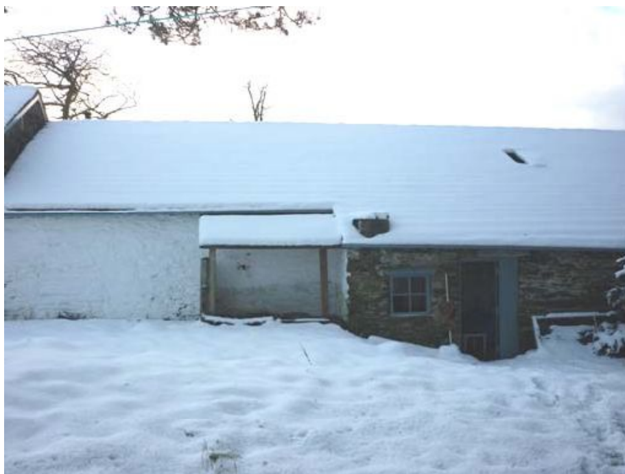
Plate 14: The north-east side of the north-west elevation
