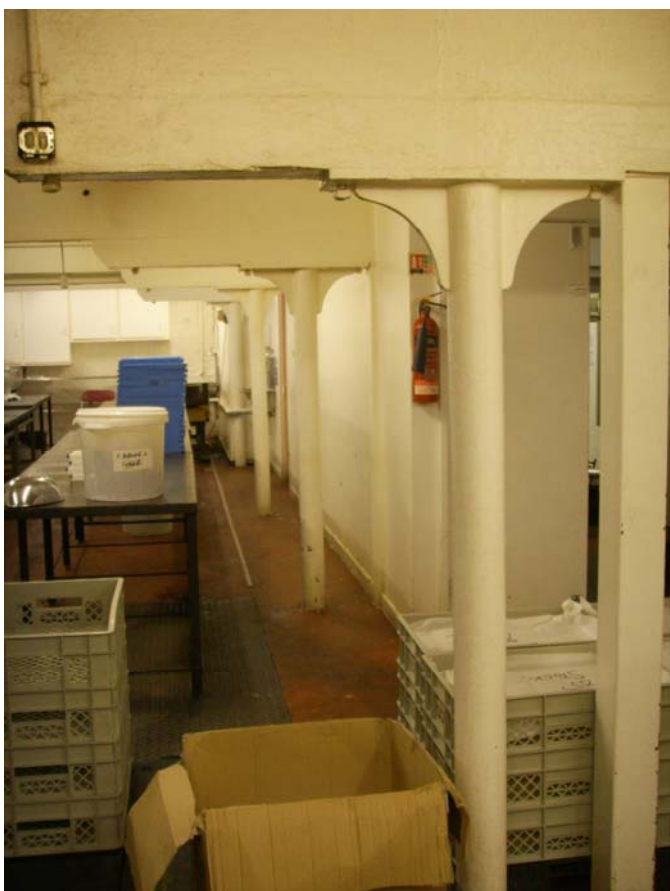
Plate 15 (left): Supporting columns on the ground floor
