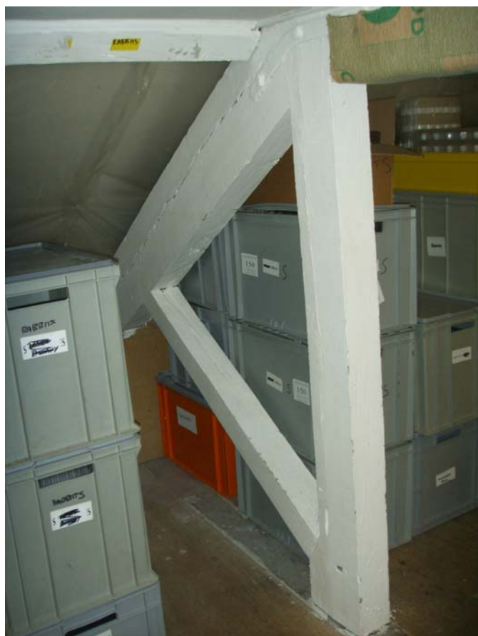
Plate 15 (left): Supporting columns on the ground floor
