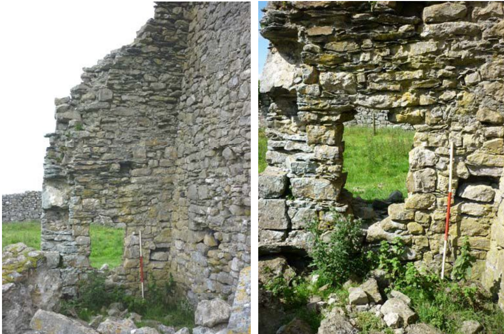
Plate 22 (left): North-east facing internal elevation of the Hall
