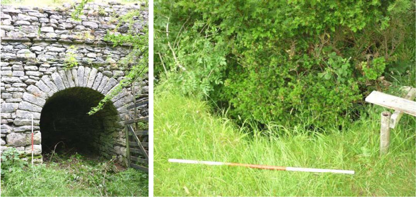
Plate 28 (left): South external elevation of the south kiln
