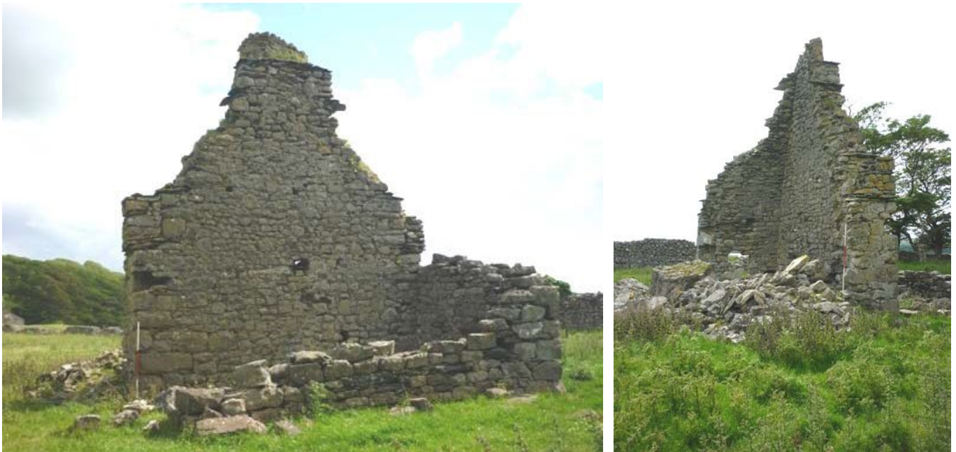
Plate 19 (left): North-west elevation of Frith Hall and the outshut
