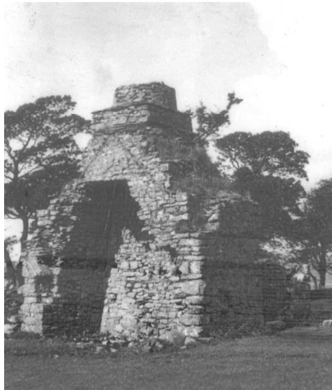
Plate 13: Photograph taken 14 th January 1969
