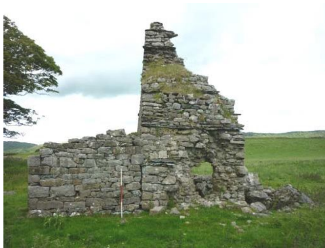
Plate 21: South-west external elevation of Frith Hall
