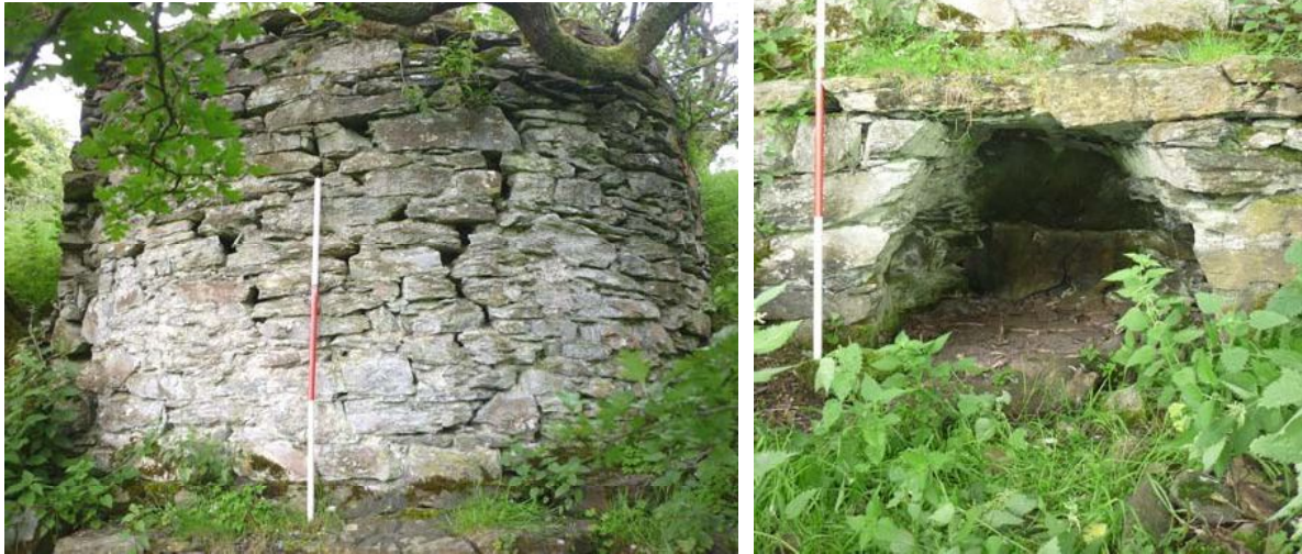
Plate 34 (left): Detail of the upper section of the north kiln
