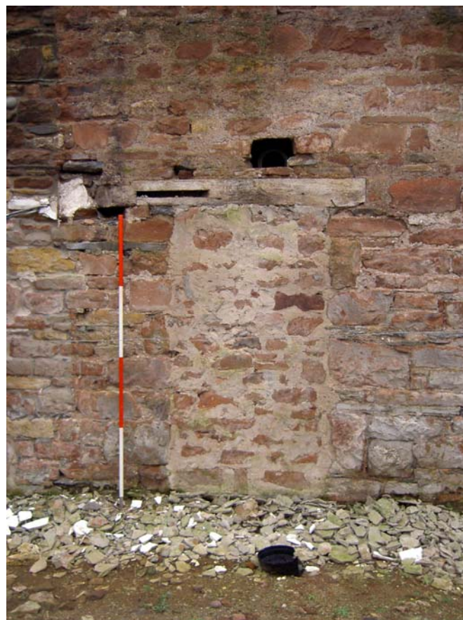
Plate 7: Re-used timber 2 used as a lintel above a blocked doorway in the north-east end of the north-west elevation of Building B
