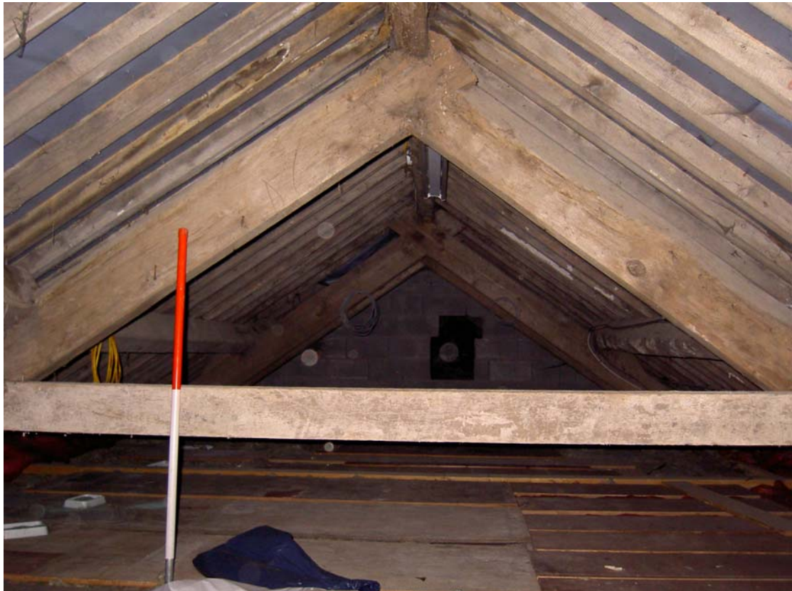
Plate 28: Truss 'III' showing the Baltic timber mark in the roofspace above the south-west end of Building B
