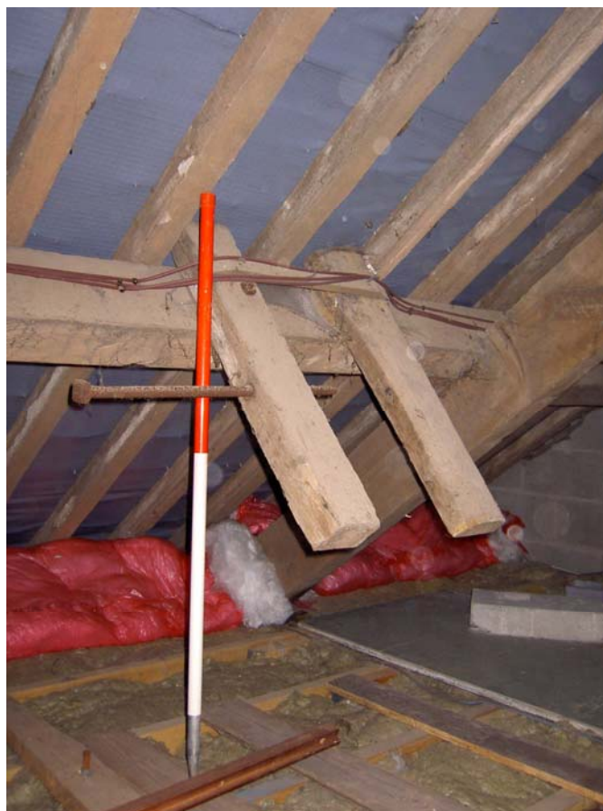
Plate 27: Hoist in the roofspace above the south-west end of Building B
