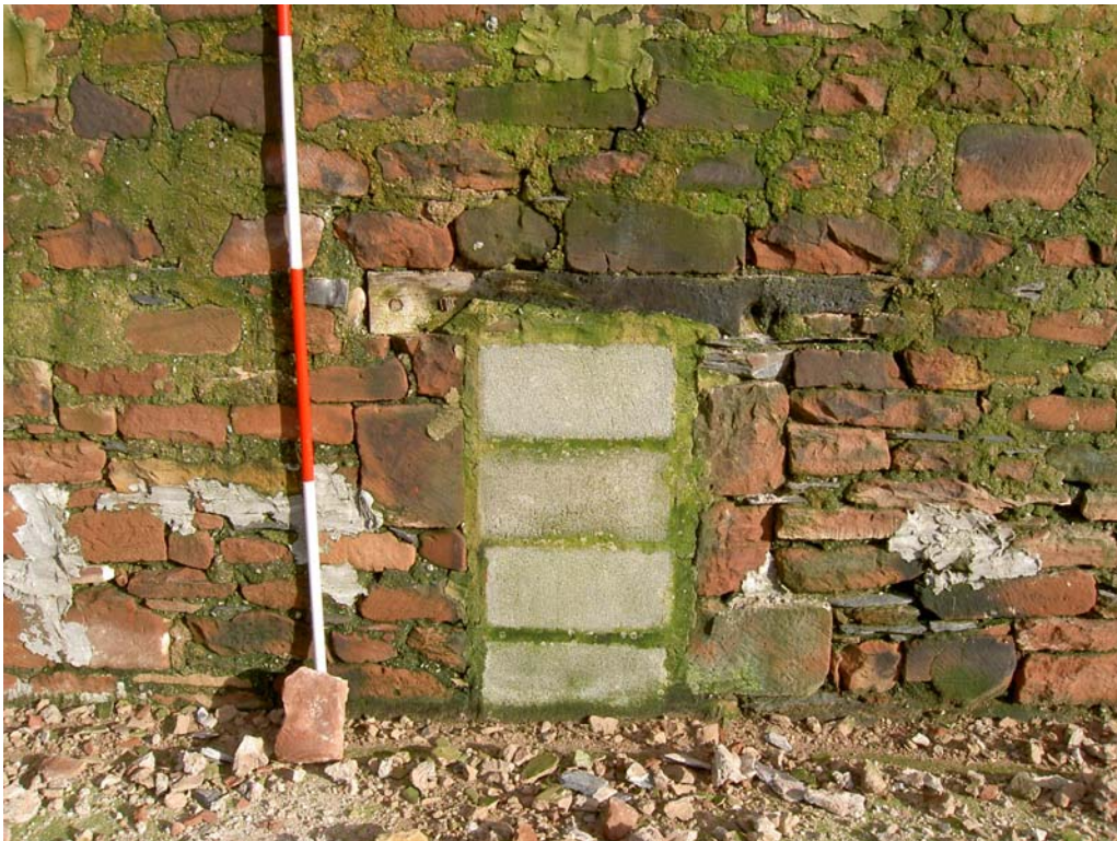
Plate 18: Re-used timber used as lintel to a ventilation slot in the north-east internal elevation of the first floor of Building A. Two masons' marks are present to the left (see plates 19 and 20)
