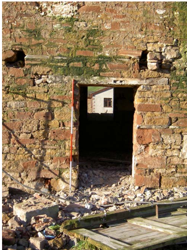
Plate 5: Re-used timber 1 used as a lintel above the south-western doorway in the north-east elevation of Building A
