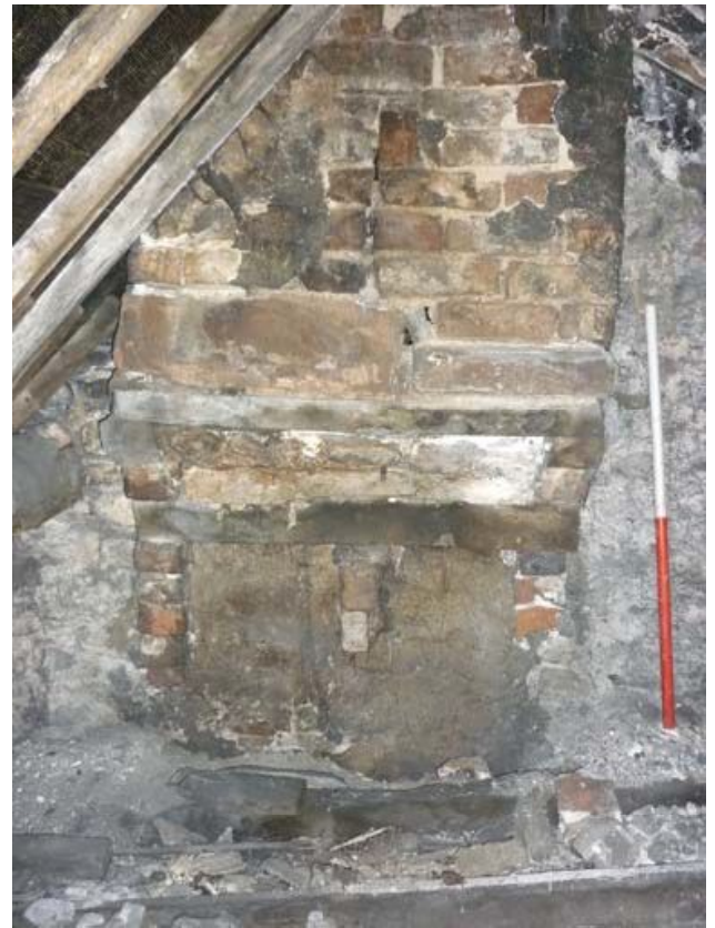
Plate 56 (left): Chimney breast in the western bay of the north roof space
