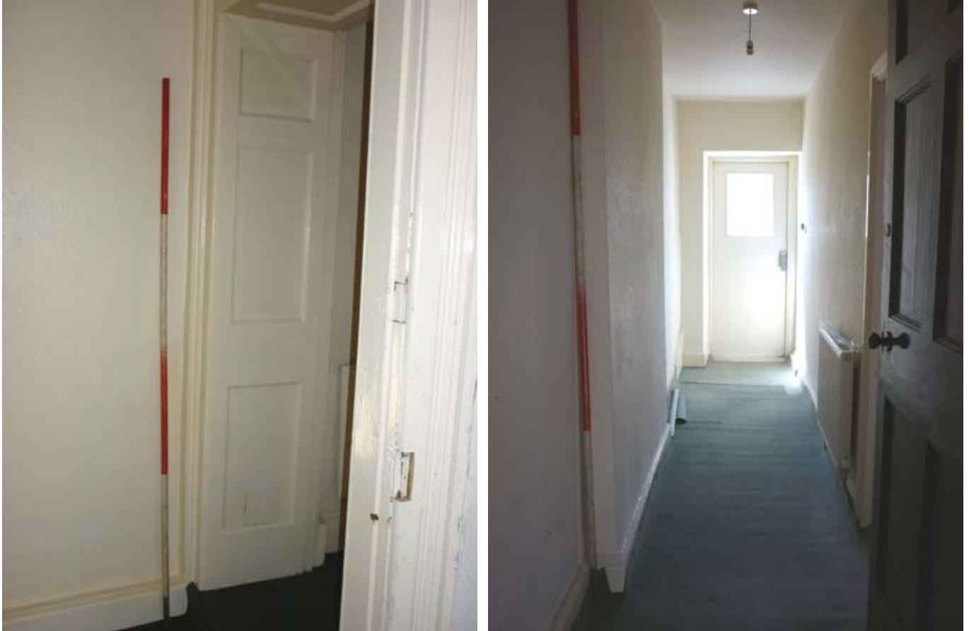
Plate 52 (left): Panelled door jamb in Room F8
