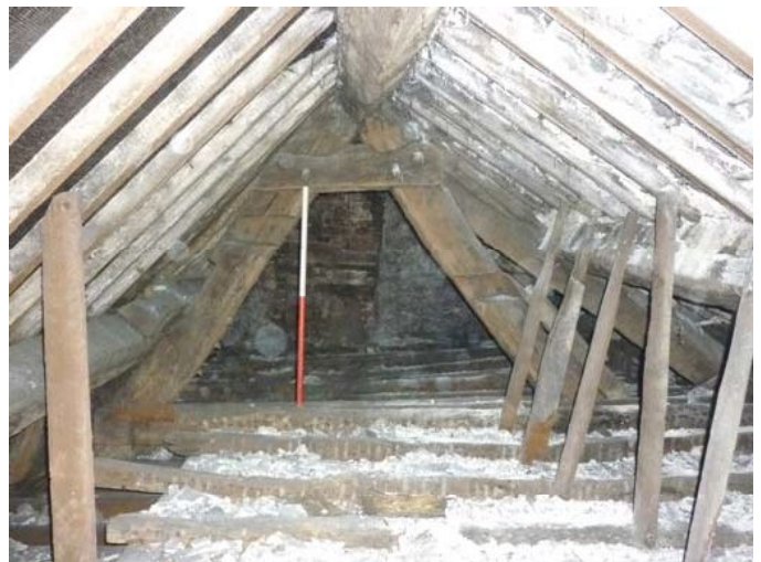
Plate 58 (left): West face of the western cruck truss
