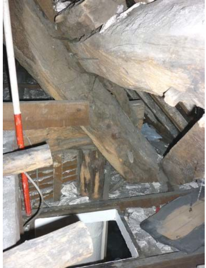
Plate 60 (left): West face of the east cruck truss
