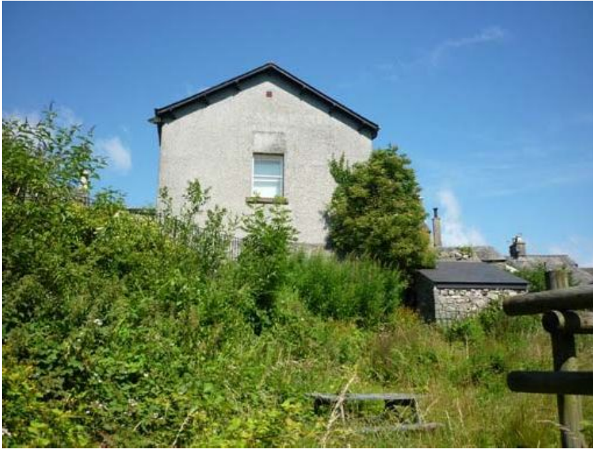
Plate 17: General view of the south external elevation and outshut
