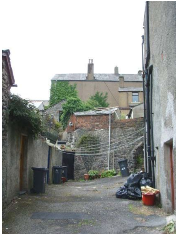
Plate 18: General view of the east external elevation
