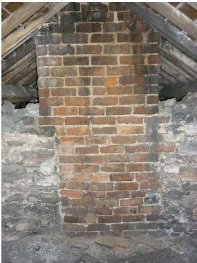
Plate 69 (left): Brick chimney stack on north side of south roof space
