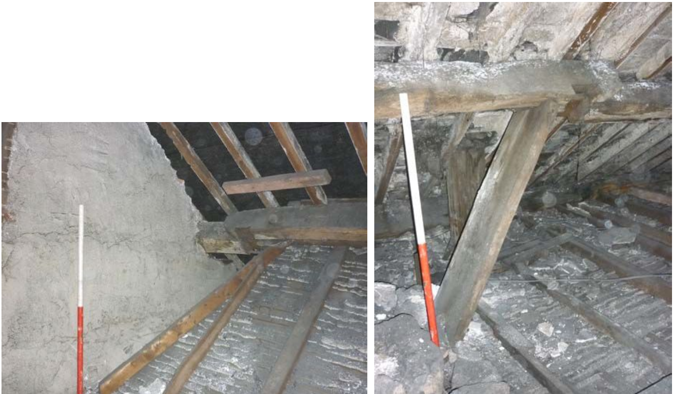
Plate 64 (left): Inserted brick wall and empty slot for truss
