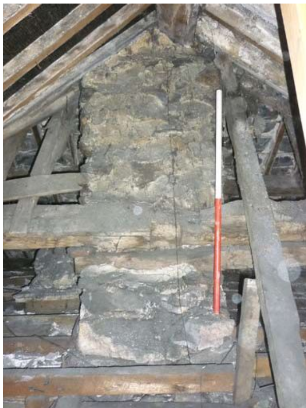
Plate 66: Wall in north roof space showing inserted purlins
