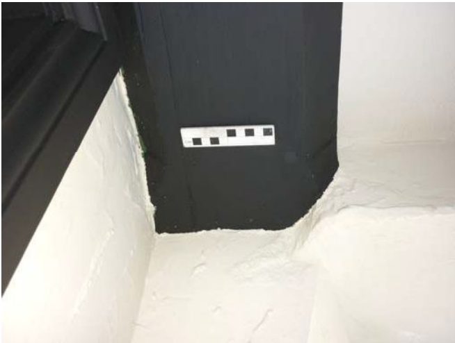
Plate 23 (left): Detail of stop-chamfer decoration
