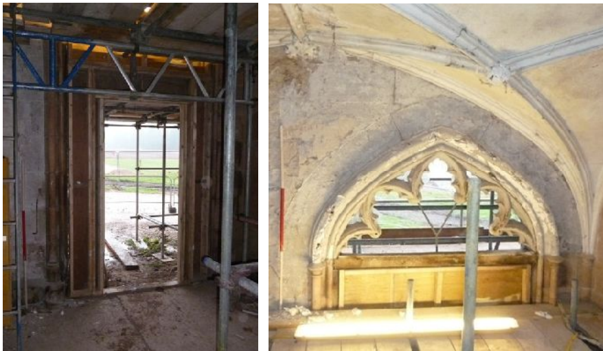
Plate 74 (left): Doorway in the south elevation of Room 5
