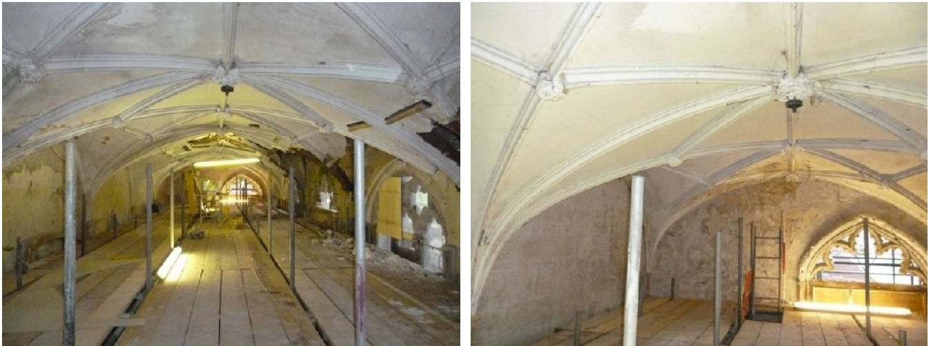
Plate 66 (left): View of the ceiling in Room 5, looking south
