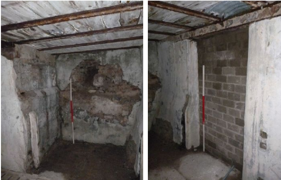
Plate 35 (left): The east and south elevations of the basement
