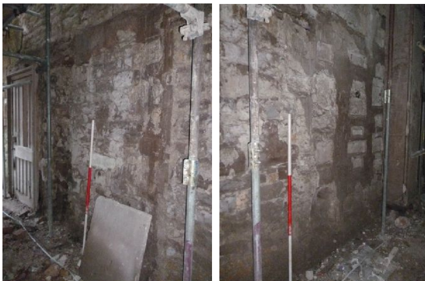
Plate 45 (left): Doorway with keystone
