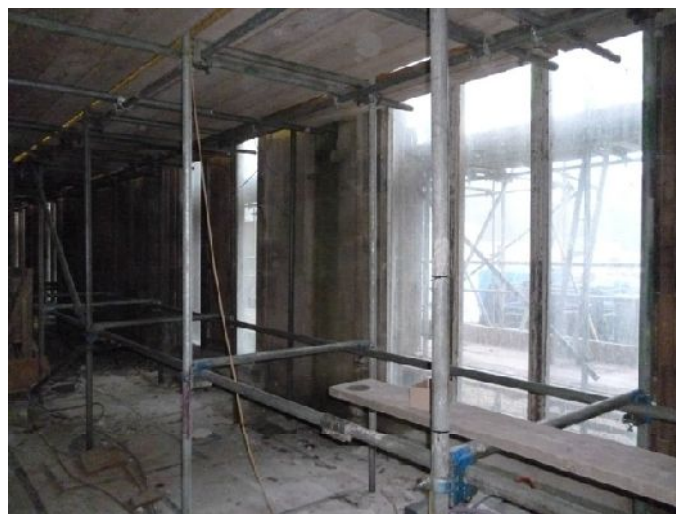
Plate 76: East elevation of Room 5
