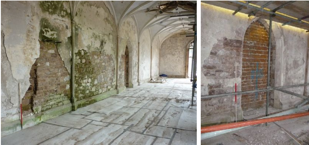
Plate 72 (left): East elevation of Room 5 (photograph taken 25 th August 2011)
