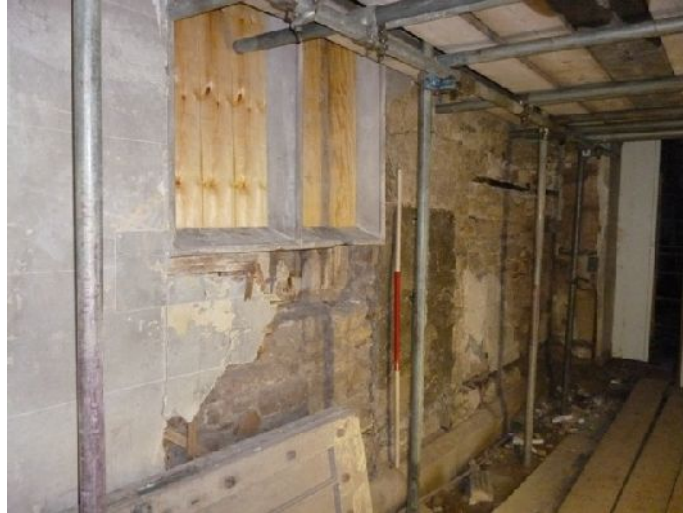
Plate 60: The west elevation of Room 3
