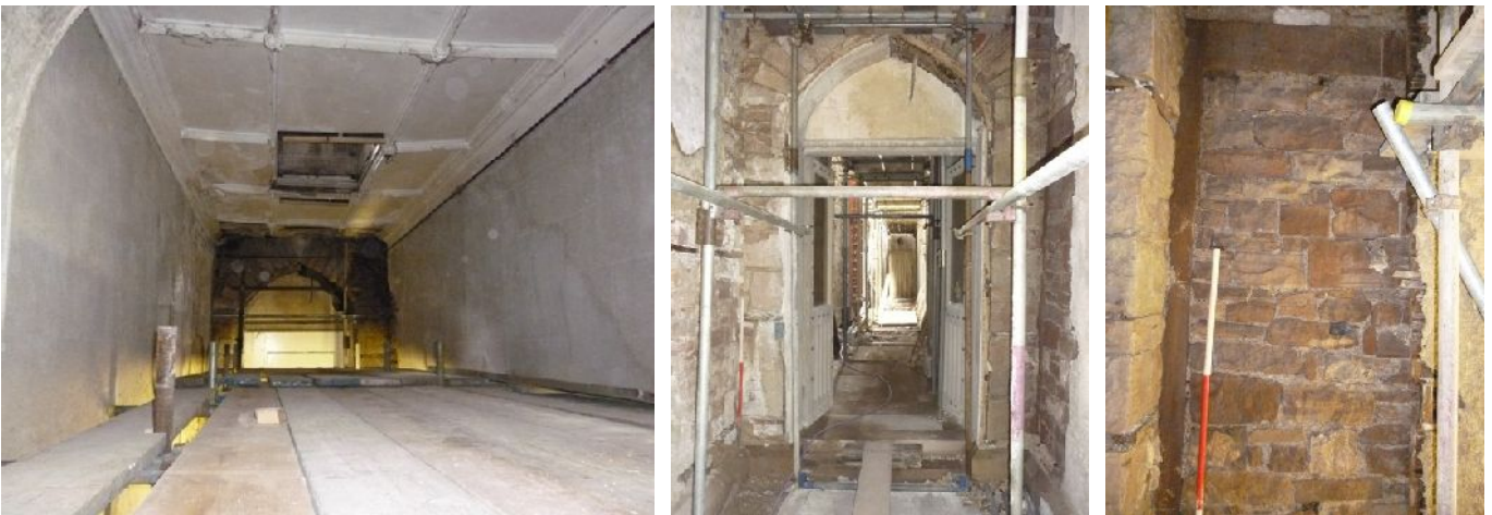
Plate 57 (left): Ceiling in Room 3
