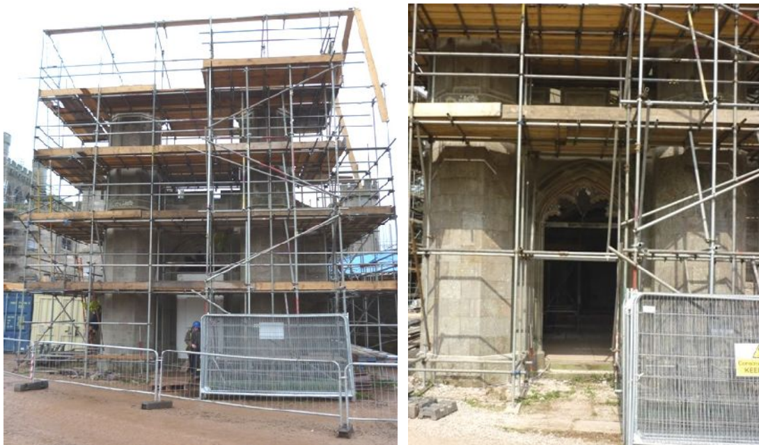
Plate 12 (left): The south external elevation
