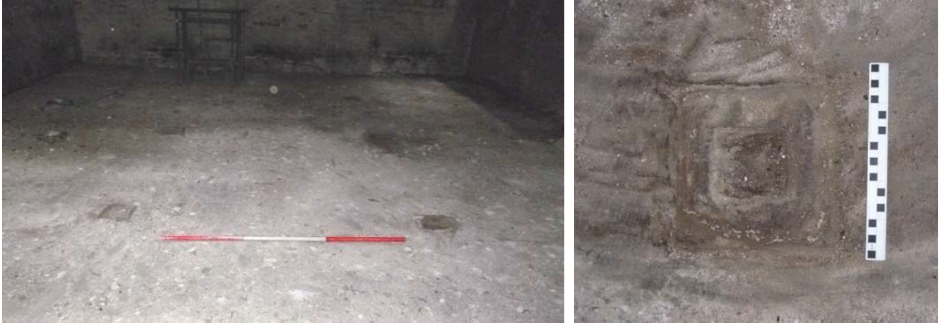
Plate 9 (left): Square sockets in the concrete floor
