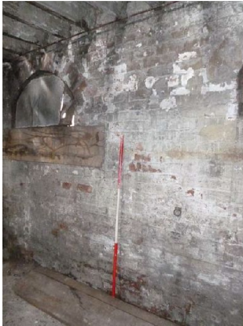
Plate 20: Iron tether ring on the south-west elevation
