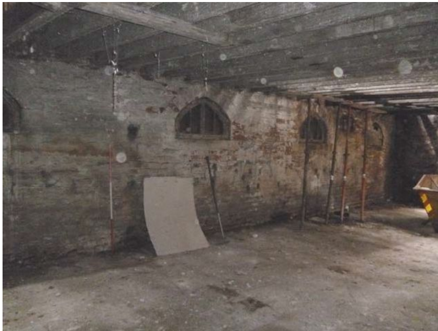
Plate 15 (left): Brick-arched windows in the south-east elevation
