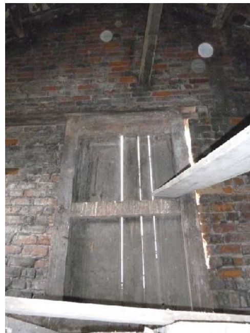
Plate 22 (left): Upper floor level loading door on the south-west elevation
