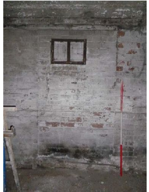
Plate 14 (right): Detail of the blocked doorway on the north-east elevation
