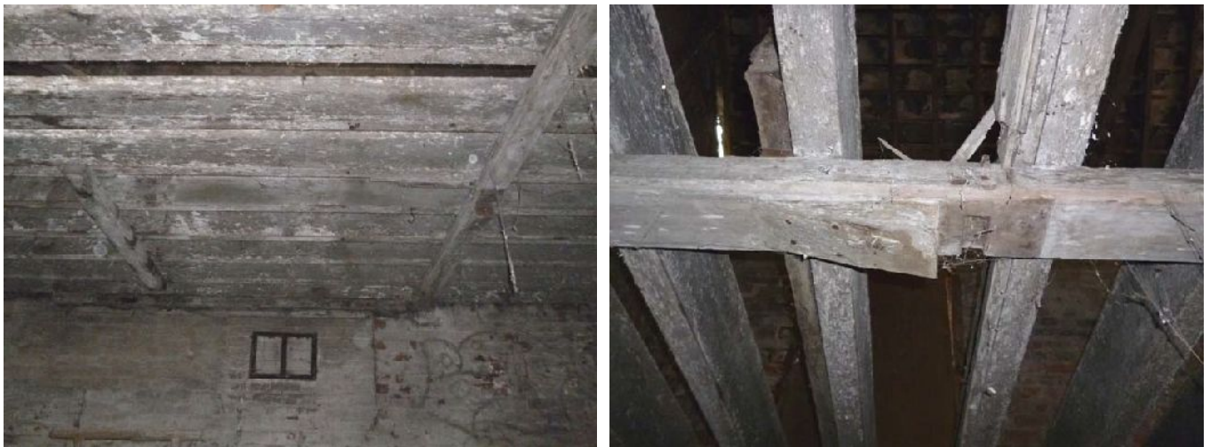
Plate 11 (left): Timbers attached below the joists at the north-east end
