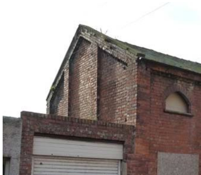
Plate 4: North-east external elevation visible above the attached garage
