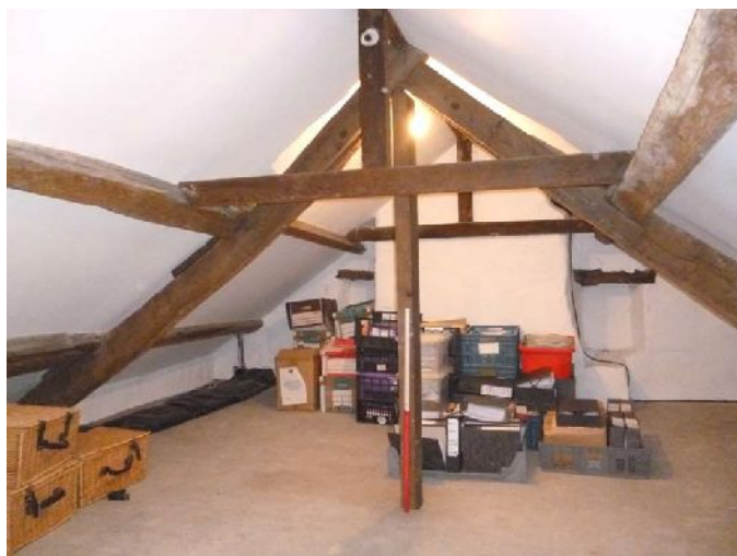
Plate 32 (left): Truss in southern section of roof space
