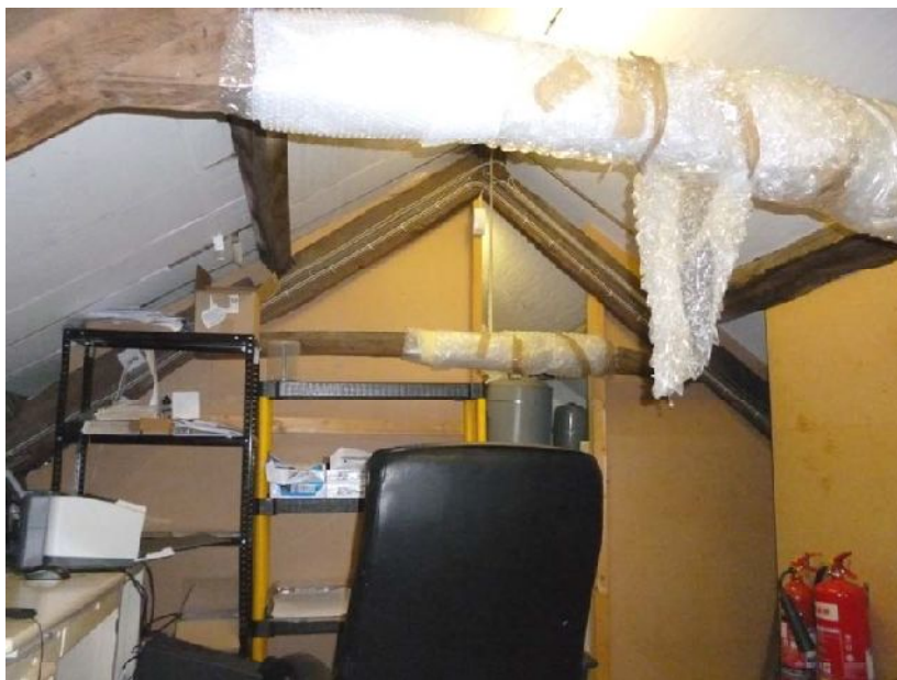
Plate 49: Truss in roof space, Rogan's
