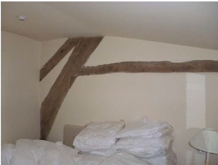
Plate 26 (left): End of cruck blade with collar and packing piece exposed in east elevation, Room F3
