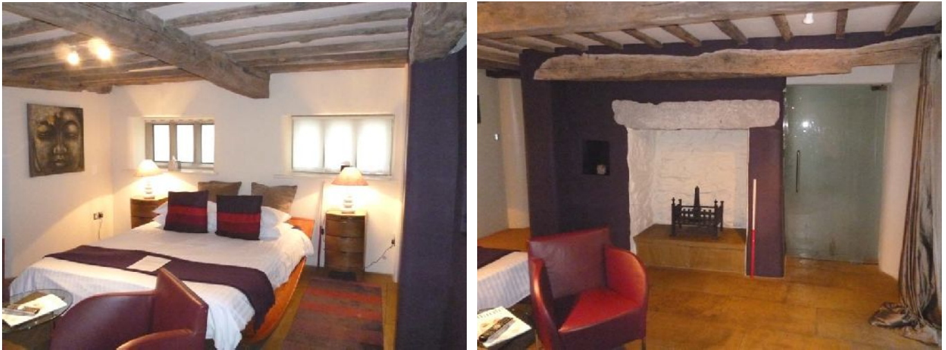
Plate 20 (left): East elevation, Room G2, showing mullion windows
