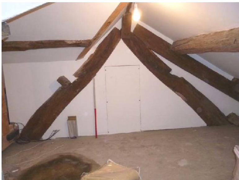
Plate 30 (left): Upper part of cruck truss within roof space
