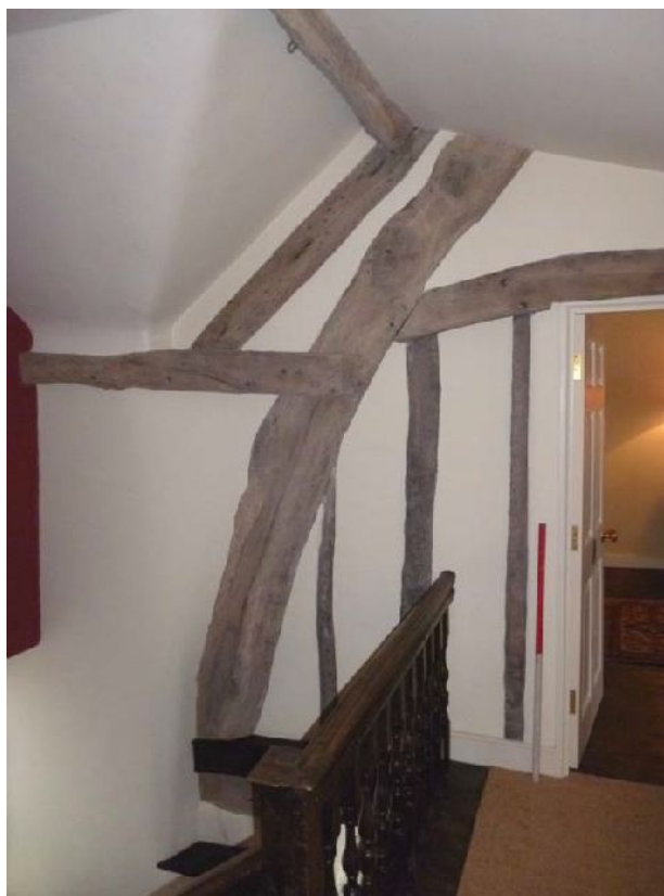
Plate 24 (left): End of cruck blade exposed in east elevation, Room F1
