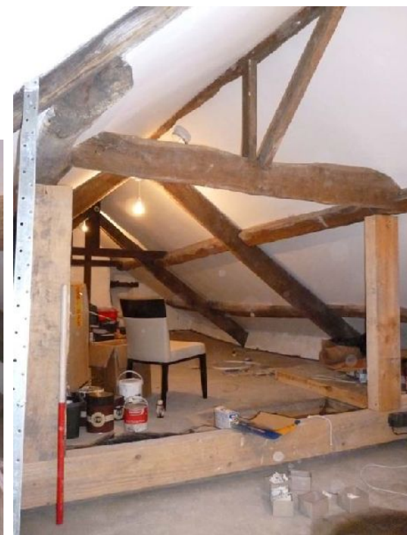
Plate 30 (left): Upper part of cruck truss within roof space
