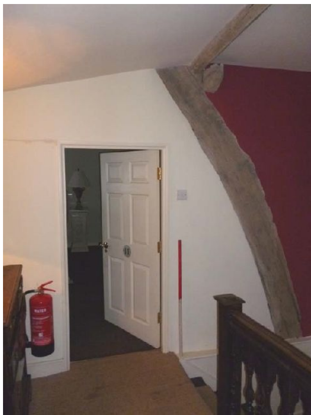
Plate 24 (left): End of cruck blade exposed in east elevation, Room F1
