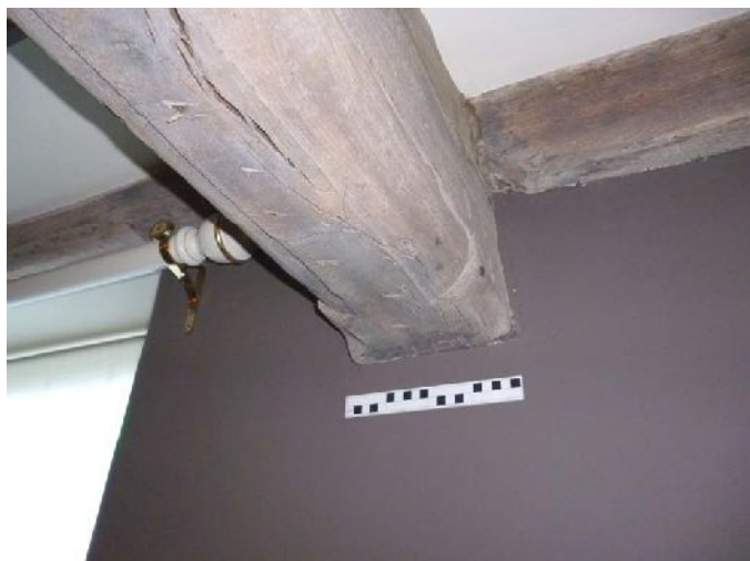
Plate 16 (left): Detail of typical moulding and stop chamfer at north end of central beams in Room G1
