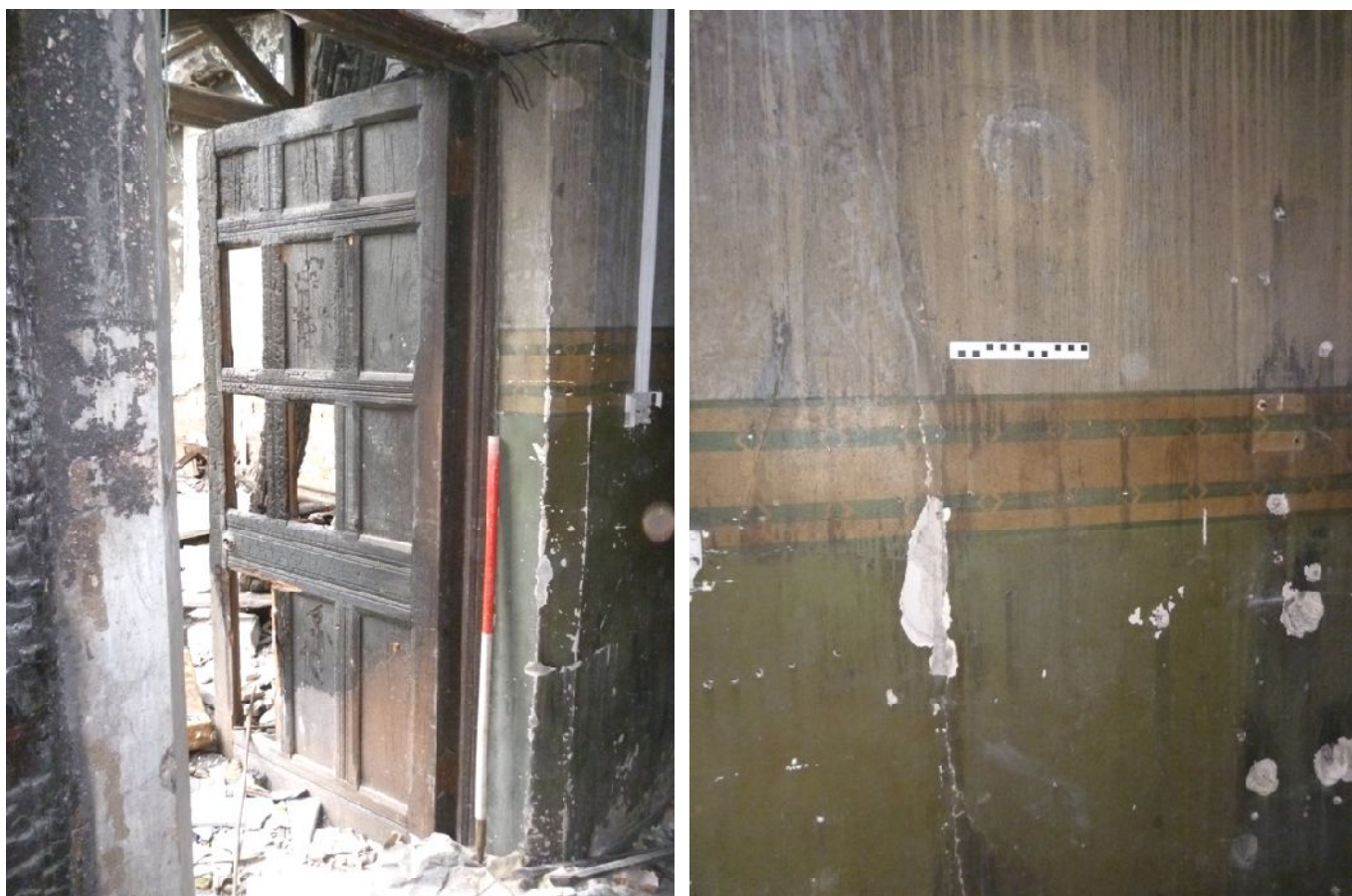
Plate 37 (left): Door in south-west elevation, Room G2
