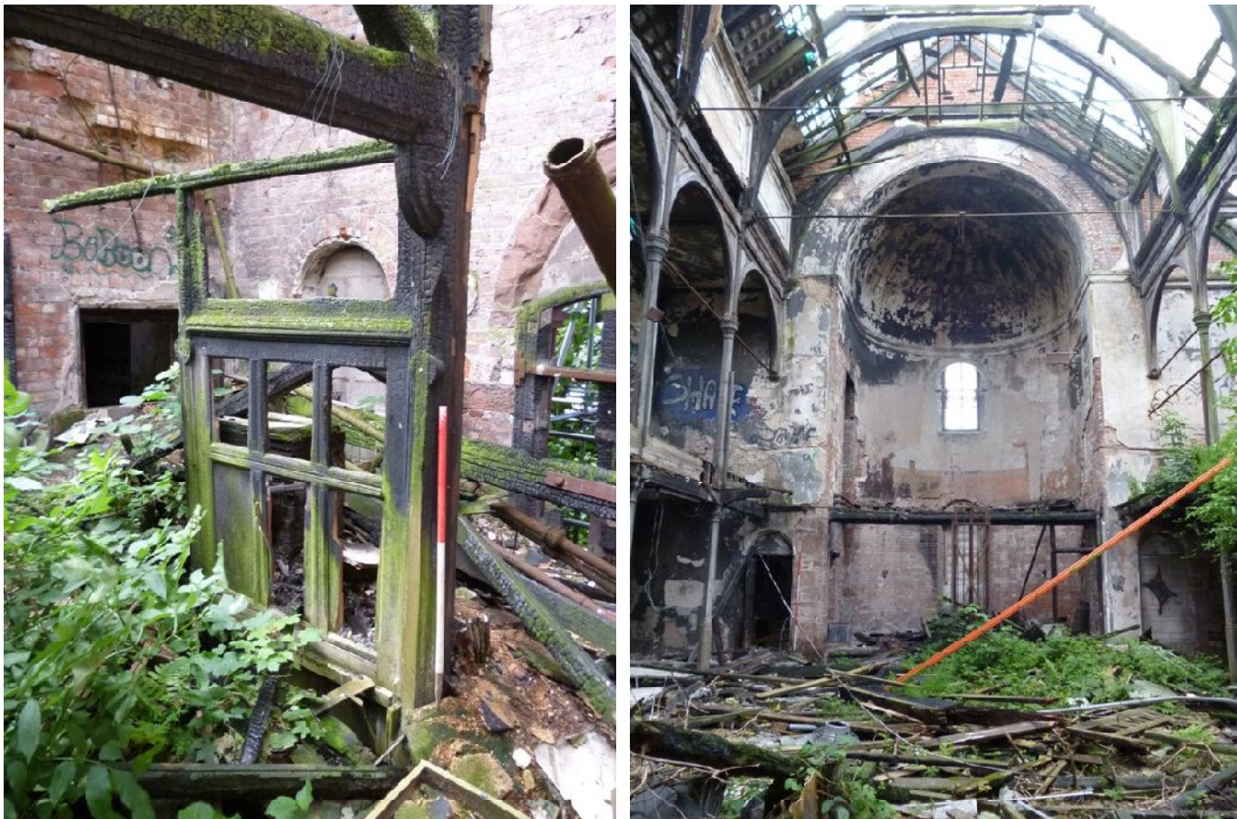
Plate 31 (left): Surviving section of stud wall at south-west end of Room G1
