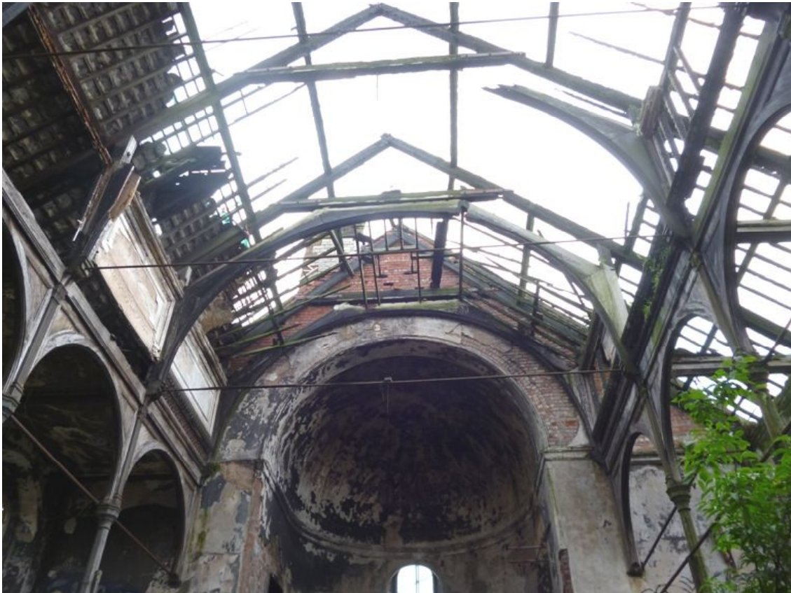
Plate 56: Typical roof trusses, Room F1
