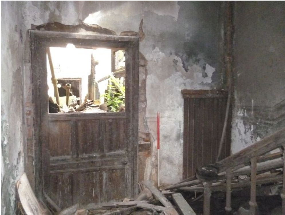
Plate 47: North-west elevation of Room G4 showing door and iron pipes
