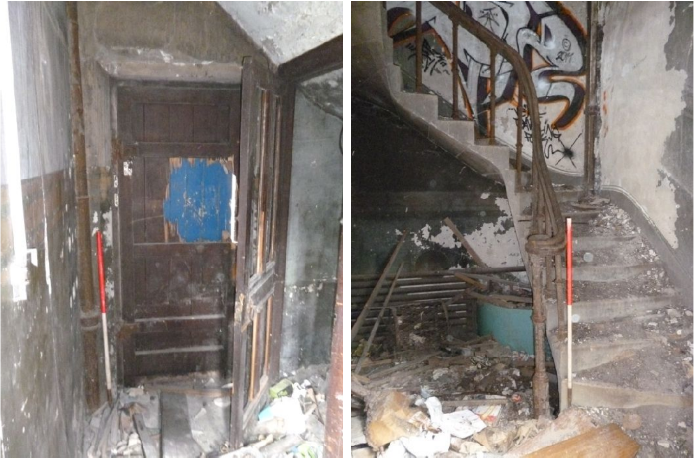
Plate 39 (left): Door in north-west elevation, Room G2
