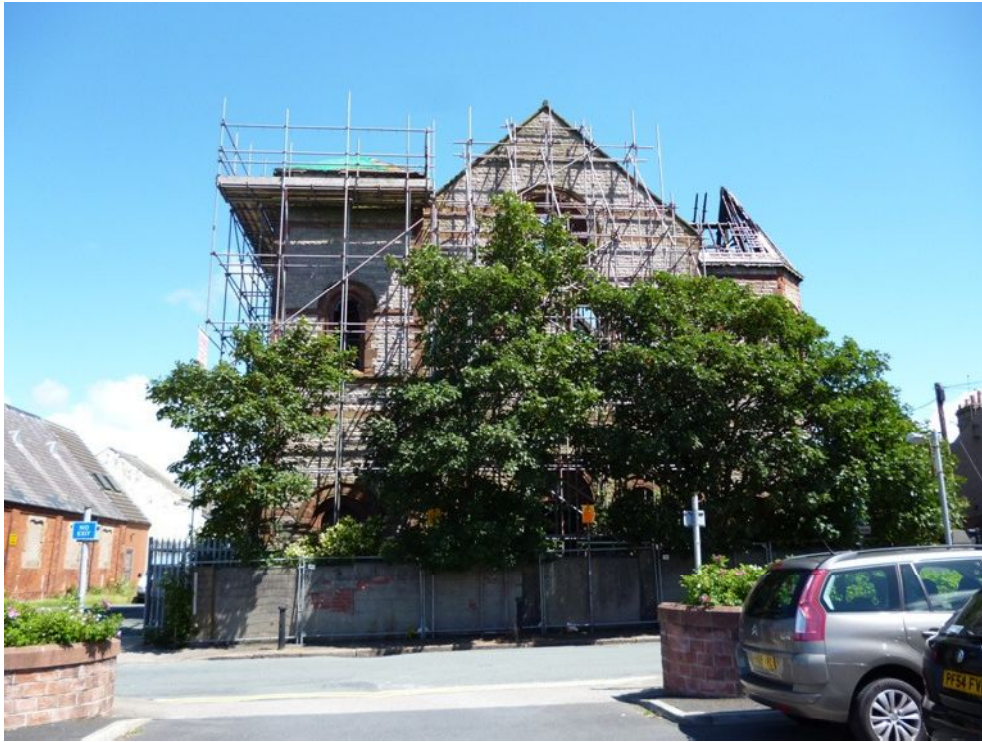
Plate 19: General view of the south-west external elevation
