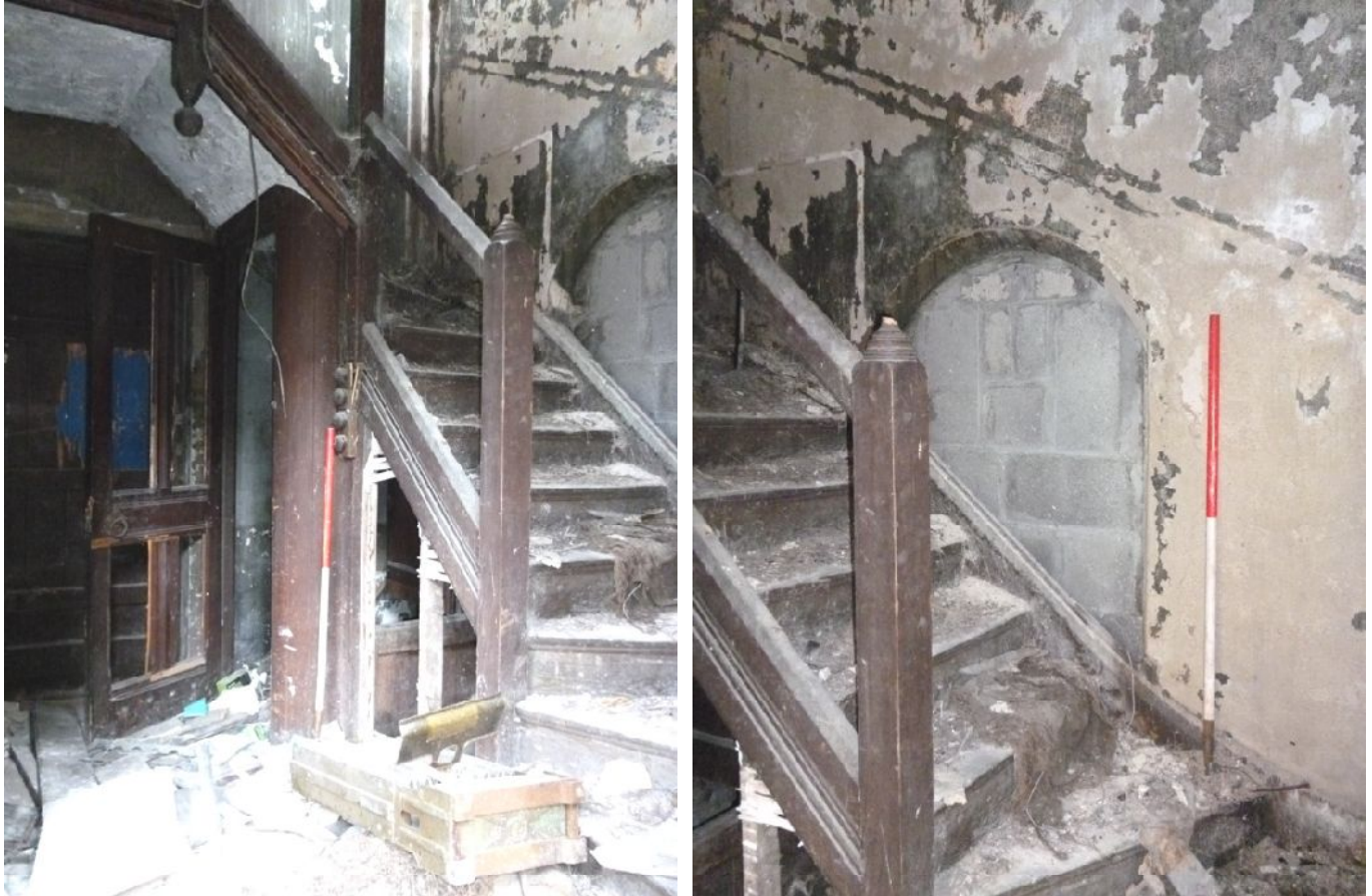
Plate 35 (left): Staircase in Room G2
