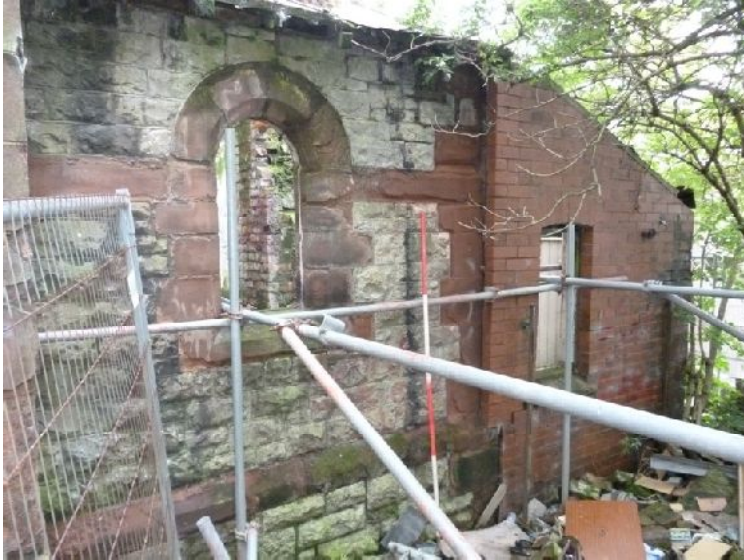
Plate 17 (left): Brick extension and outshut at north-east end
