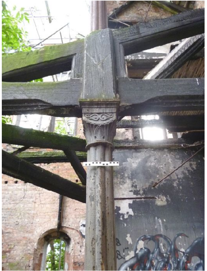
Plate 27 (left): General view of arrangement of columns and beams supporting gallery, north-west side of Room G1
