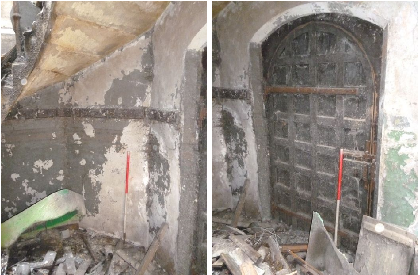
Plate 45 (left): Timber bracket forming coat hook around south corner of Room G4
