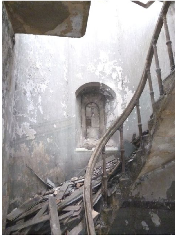
Plate 61: Small window in south-east elevation of Room F4
