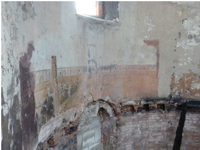
Plate 57 (left): Paint scheme within the apse, north-east end of Room F1
