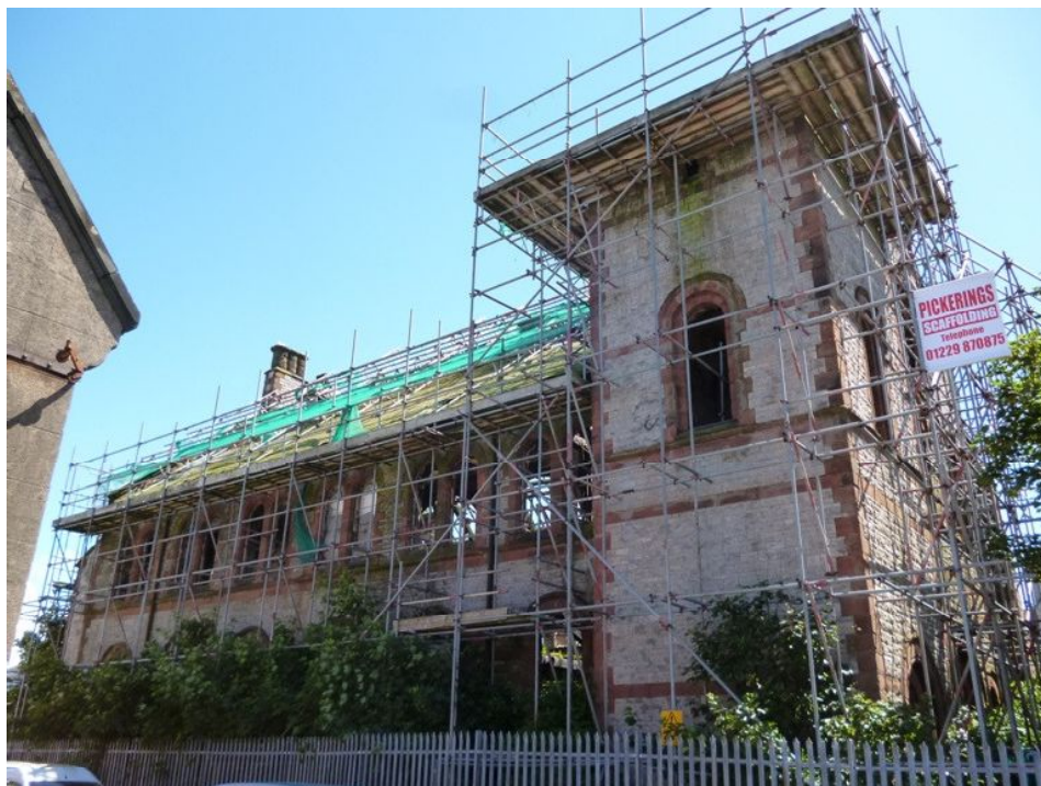
Plate 26 (right): General view of north-west external elevation
