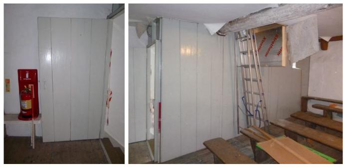
Plate 64 (left): Detail of the door to First Floor room 1 Plate 65 (right): Stud wall along the side of the stairs, viewed from First Floor Room 1
