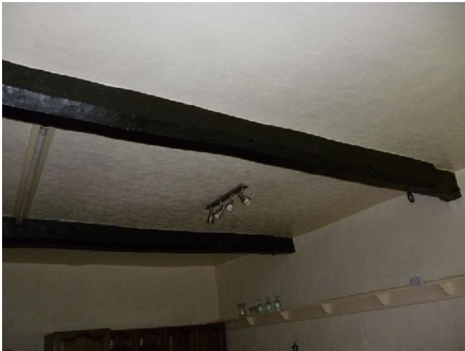
Plate 30 (left): North/south beams in Ground Floor Room 4
