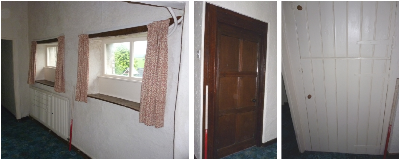
Plate 70 (left): Windows in the west elevation of First Floor Room 3
