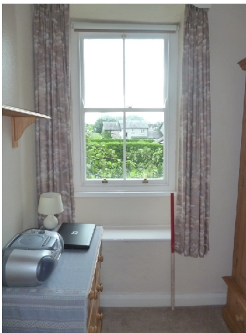
Plate 83: Window in the south elevation of First Floor Room 9
