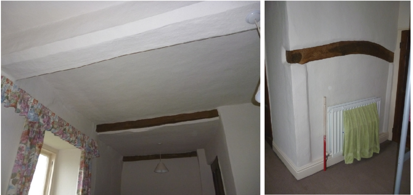
Plate 59 (left): Beams in First Floor Room 2
