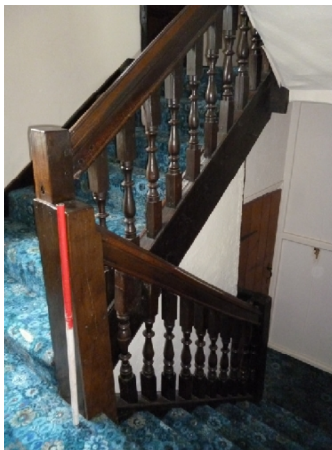
Plate 80: Stairs from First Floor Room 6 to Ground Floor Room 7
