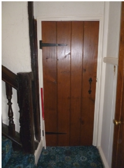
Plate 40: West elevation of Ground Floor Room 7
