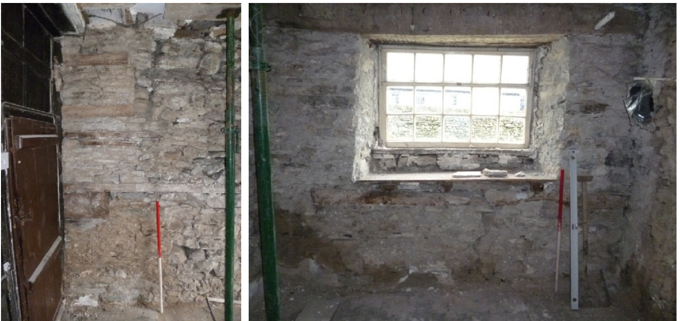
Plate 47 (left): The south-east corner of Ground Floor Room 9
