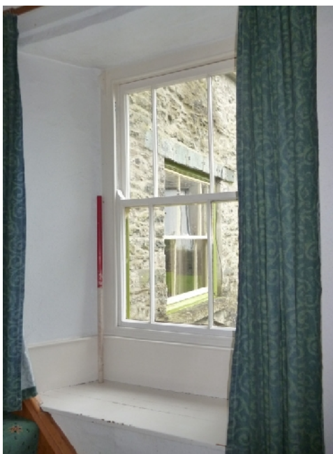
Plate 56: Window in the north elevation of Ground Floor Room 14
