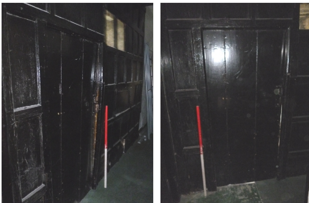
Plate 43 (left): The panel wall in Ground Floor Room 8
