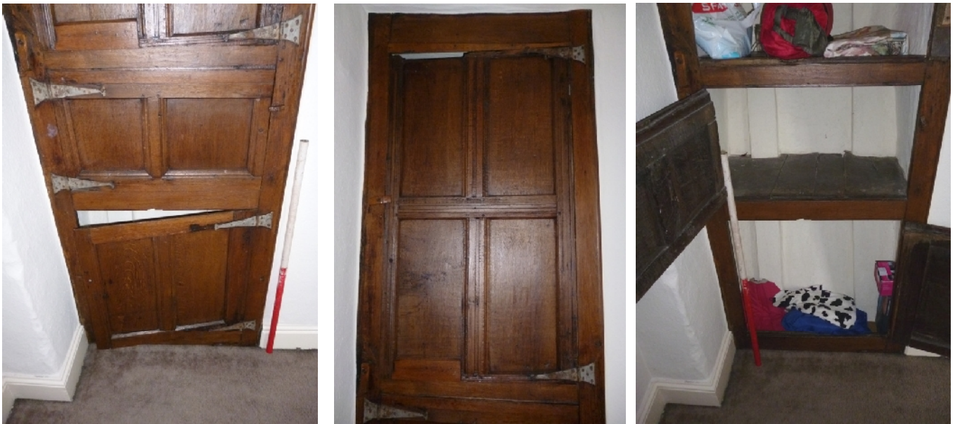
Plate 63 (left): Detail of the lower cupboard doors in First Floor Room 2
