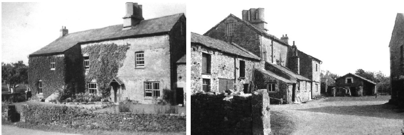
Plate 5 (left): Early 20 th century photograph of the east elevation (after Inglesfield 2006, 44)
