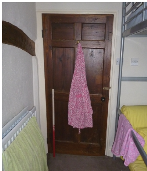
Plate 66: Doorway in the west elevation of First Floor Room 2
