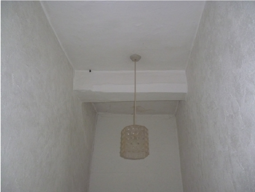
Plate 81 (left): Stop chamfered beam in First Floor Room 7
