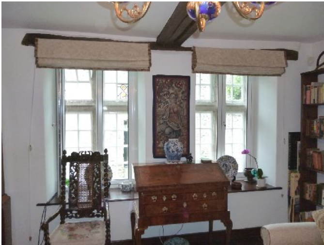
Plate 7 (left): Typical two-light secondary glazing in the southern windows, first floor
