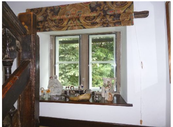
Plate 9 (left): Typical secondary glazing in the southern windows, ground floor
