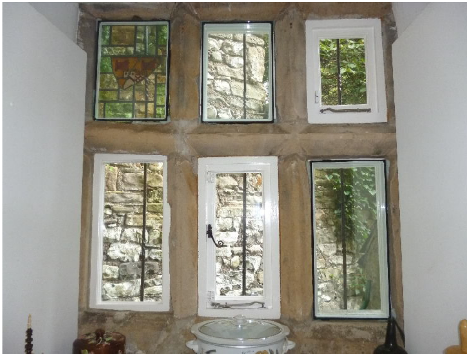
Plate 11: Multiple single-light glazing in the north elevation
