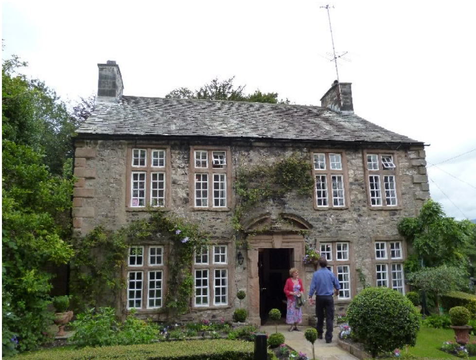
Plate 6: General view of the front (south) external elevation
