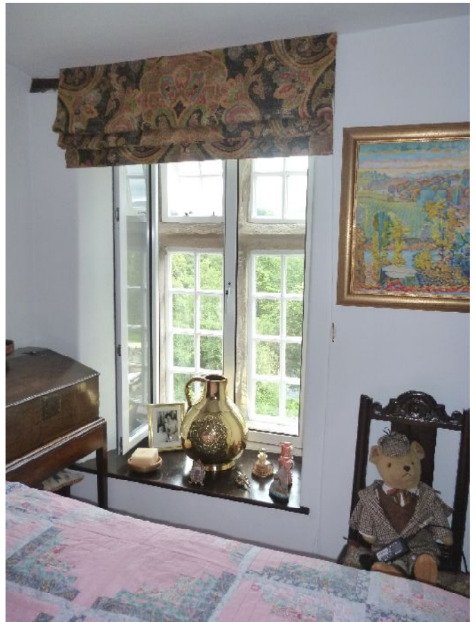
Plate 7 (left): Typical two-light secondary glazing in the southern windows, first floor
