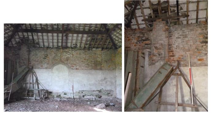
Plate 24 (left): North-east internal elevation Plate 25 (right): Detail of flue on north-west side of north-east internal elevation
