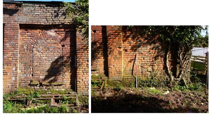
Plate 19 (left): Central blocked window, south-west external elevation Plate 20 (right): Blocked aperture, south-west external elevation
