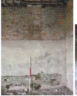
Plate 26 (left): Scar of flue, south-east side of north-east internal elevation Plate 27 (right): South-east internal elevation
