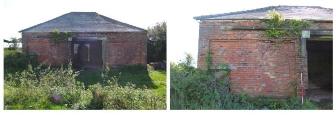
Plate 11 (left): The north-west external elevation Plate 12 (right): Blocked doorway, rebuild, and window, north-east side of north-west external elevation
