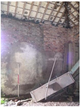
Plate 23: Blocked window and rebuild line, north-east end of north-west internal elevation
