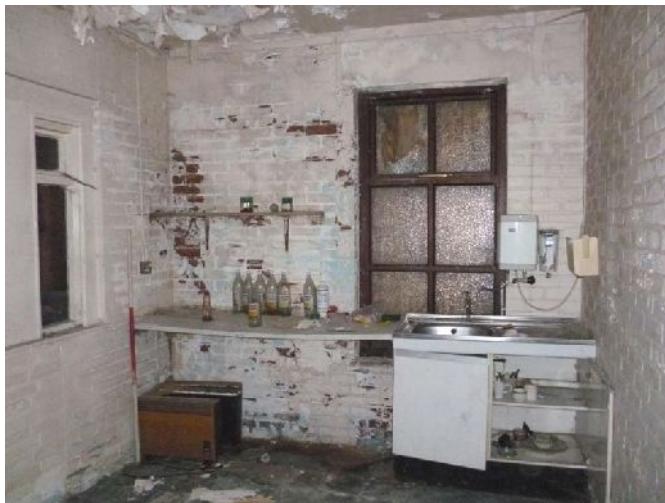
Plate 192: West elevation of West Building, Ground Floor Room 5
