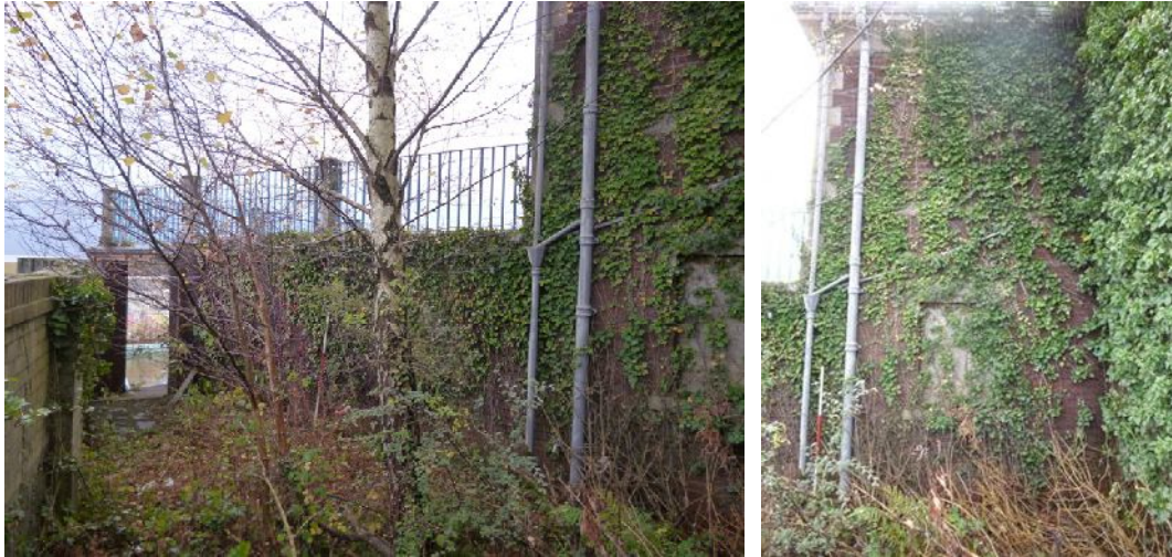
Plate 26 (left): East end of the north elevation of the north building
