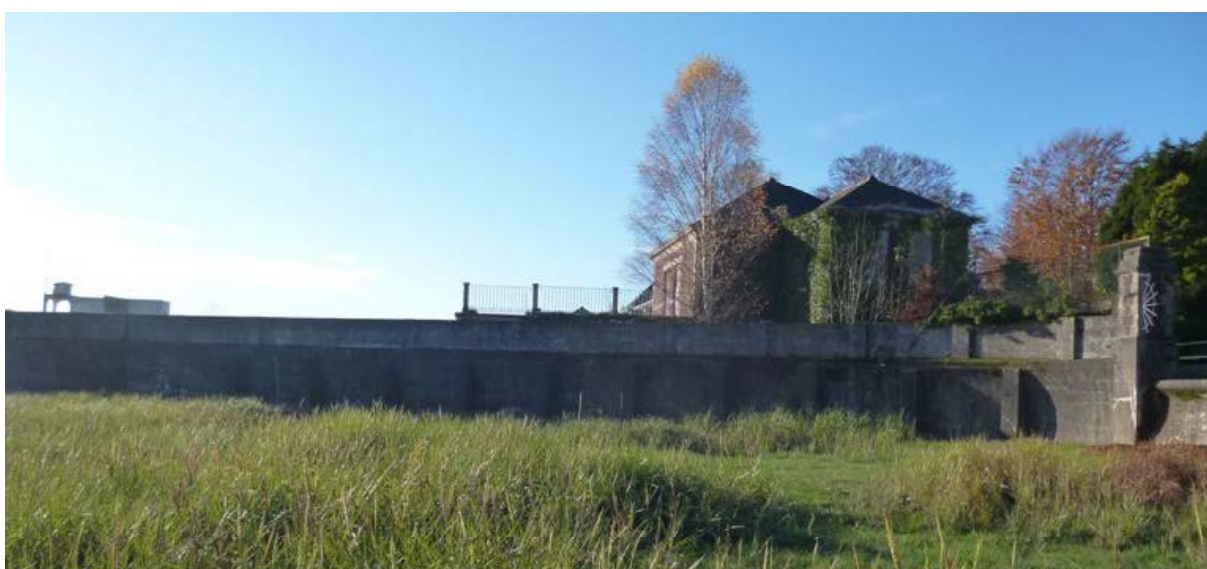
Plate 80: North end of the outer retaining wall
