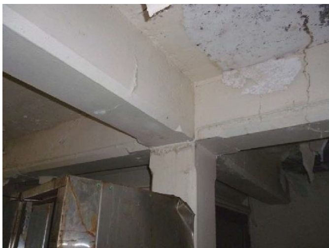
Plate 137 (left): Stop-chamfered beams in South Building, Ground Floor Room 6
