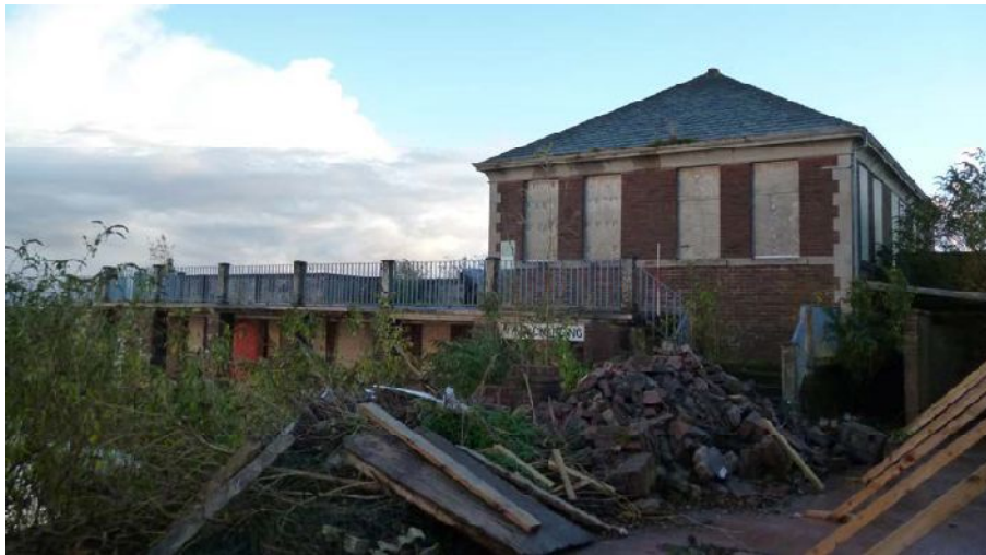
Plate 43: General view of the north elevation of the south building
