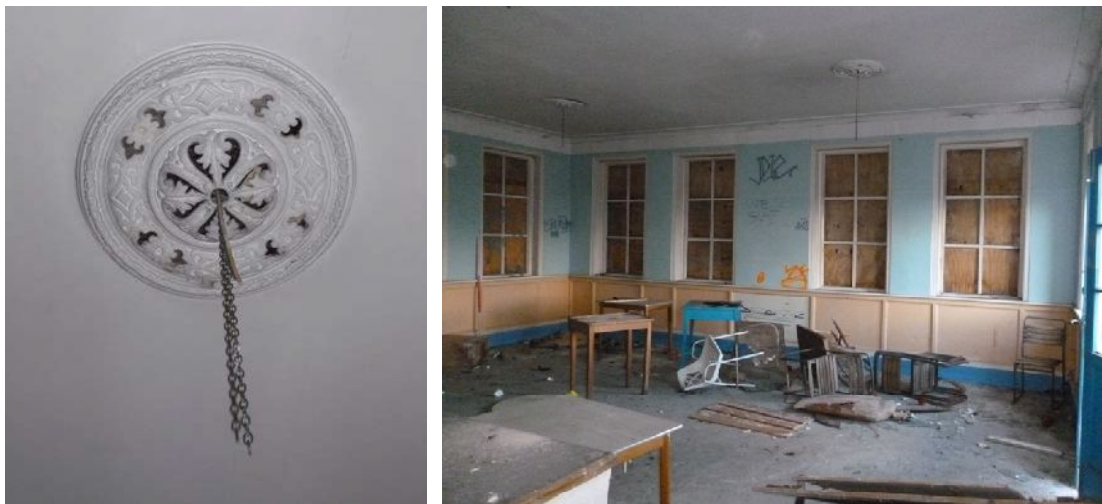
Plate 153 (left): Ceiling rose in South Building, First Floor Room 1
