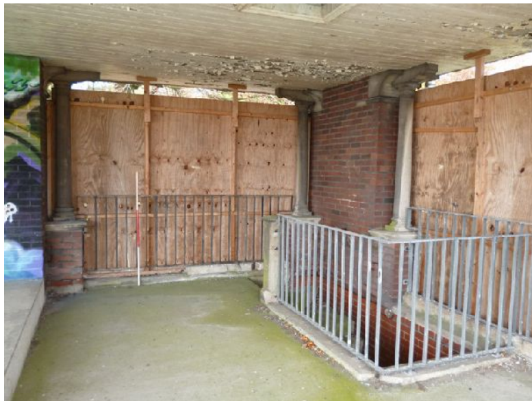
Plate 208: North-west corner of the first floor of the West Building
