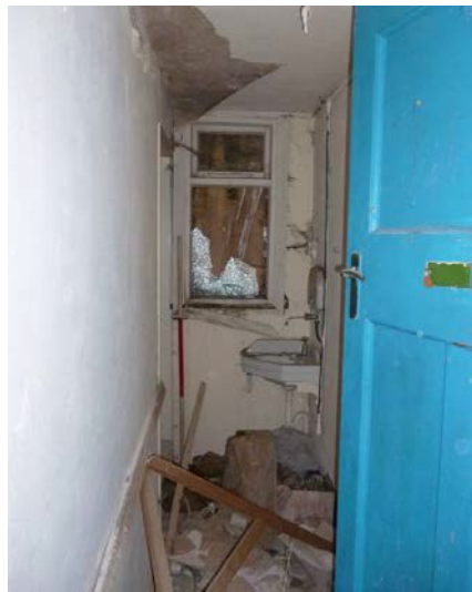
Plate 163: Window in the south elevation of South Building, First Floor Room 3
