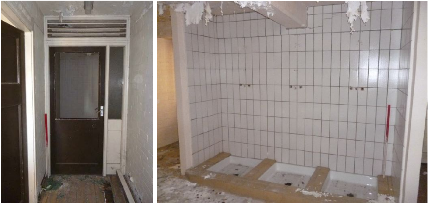
Plate 86 (left): Dividing door in the centre of the corridor in North Building, Ground Floor Room 3
