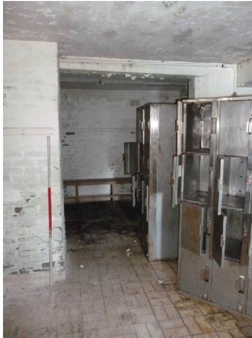
Plate 145: Opening to South Building, Ground Floor Room 7, from Ground Floor Room 6
