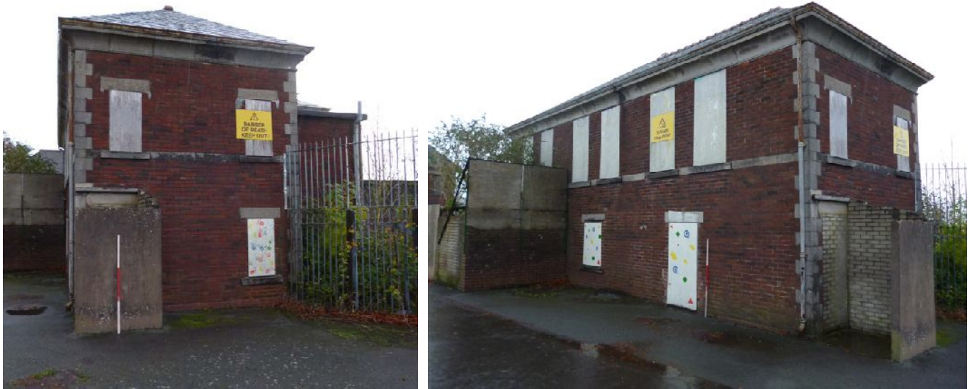
Plate 48 (left): West end of the south elevation of the south building
