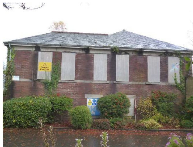
Plate 35: West elevation of the north building
