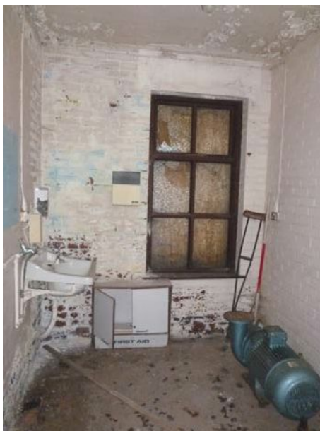
Plate 195: West elevation of West Building, Ground Floor Room 7
