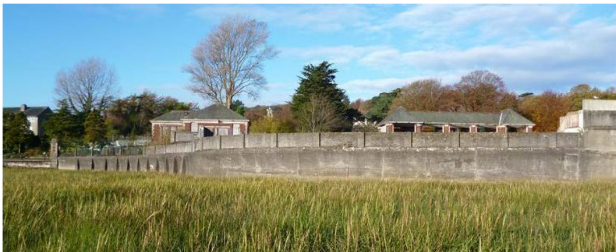
Plate 78: South and east elevations of the outer retaining wall
