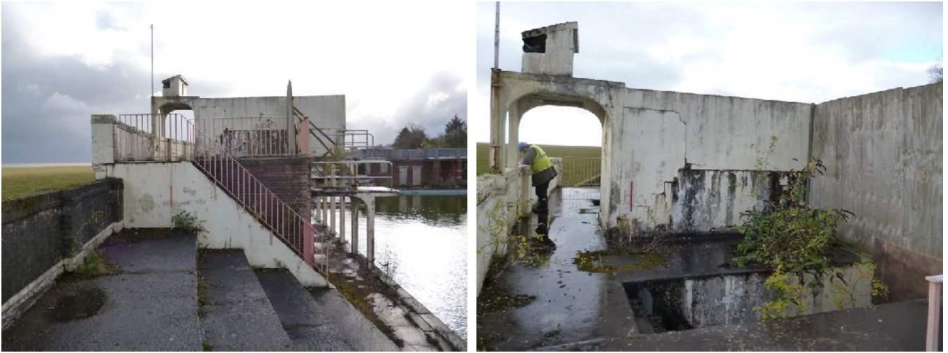
Plate 36 (left): North elevation of the east building
