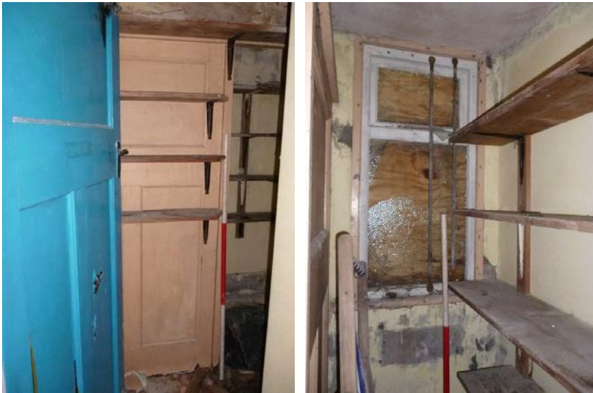
Plate 161 (left): Partition in South Building, First Floor Room 2
