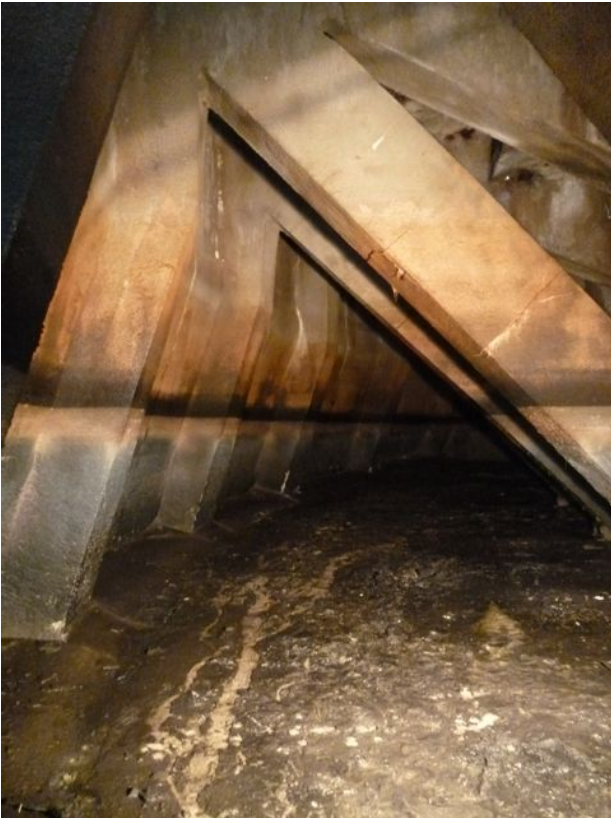
Plate 211 (left): Typical concrete struts in the south sea tank
