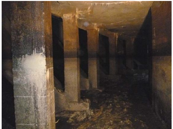
Plate 211 (left): Typical concrete struts in the south sea tank
