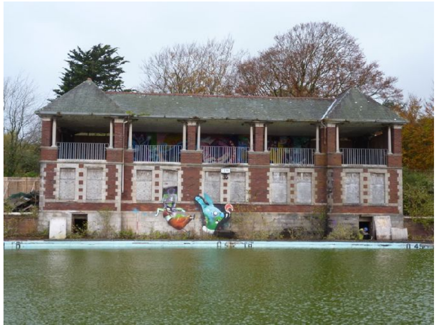
Plate 50 (left): North elevation of the west building
