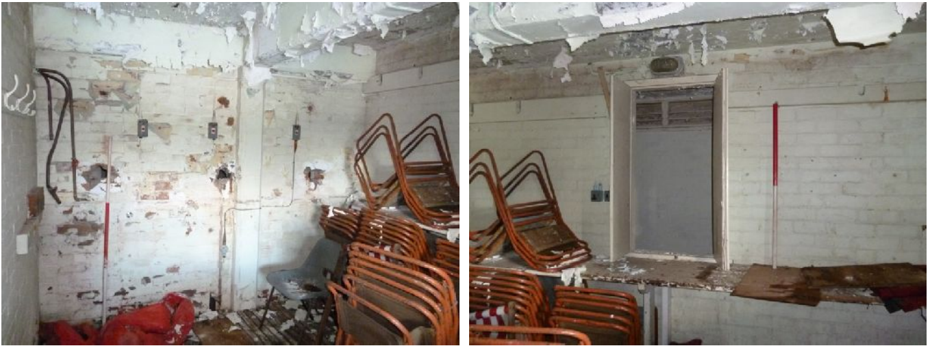
Plate 133 (left): South elevation of South Building, Ground Floor Room 5
