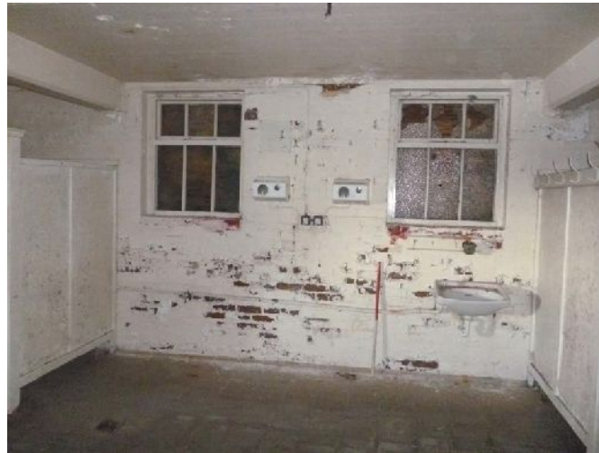
Plate 96: Windows on the west elevation of North Building, Ground Floor Room 4
