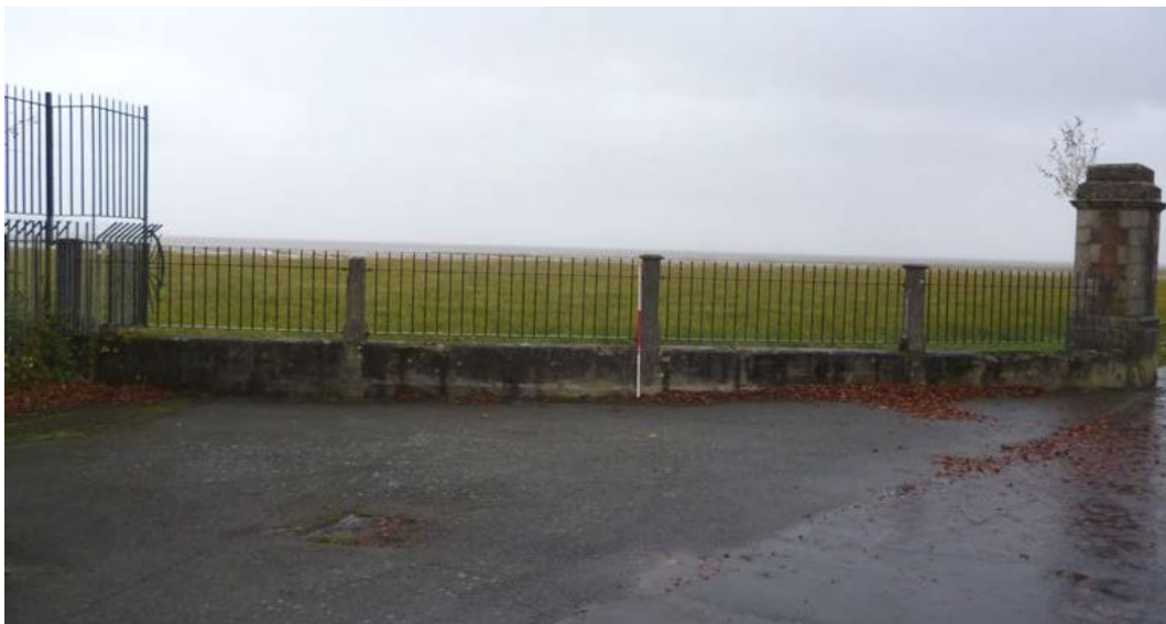
Plate 76: Fencing at the south end atop the outer retaining wall
