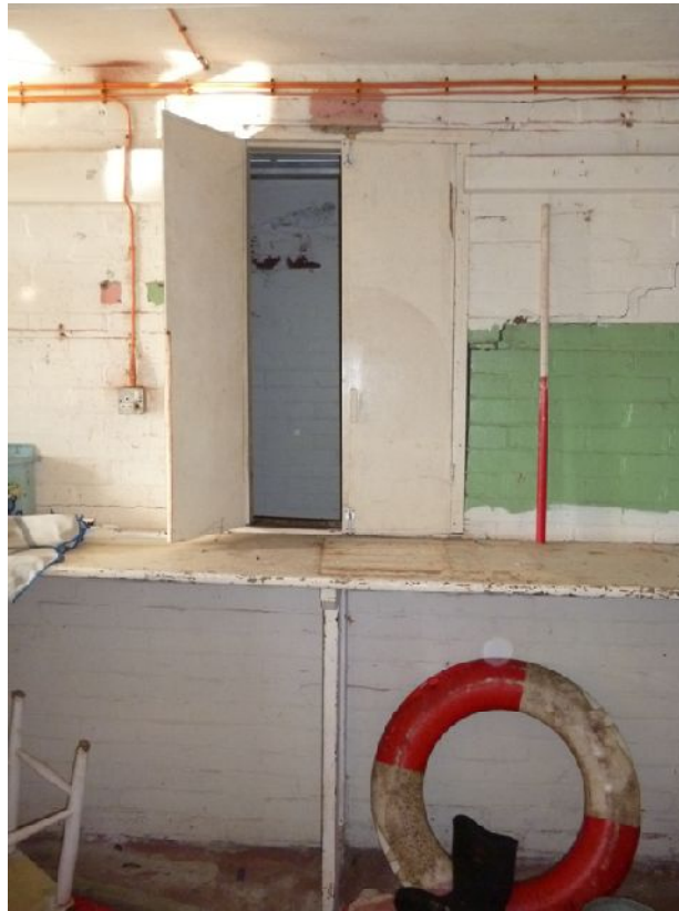
Plate 85: Cupboard on the west elevation of North Building, Ground Floor Room 1
