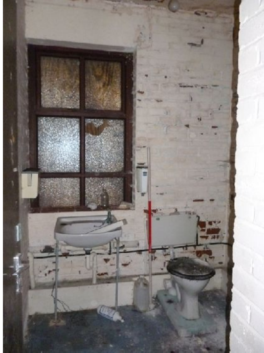
Plate 189: West elevation of West Building, Ground Floor Room 4
