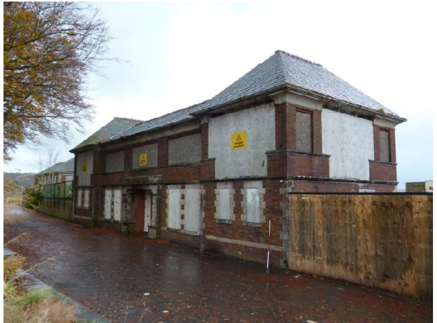
Plate 52 (left): South elevation of the west building
