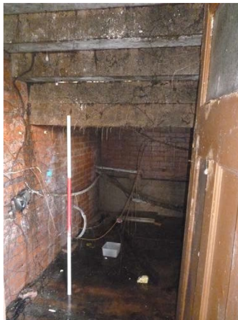
Plate 152: South Building, Ground Floor Room 10
