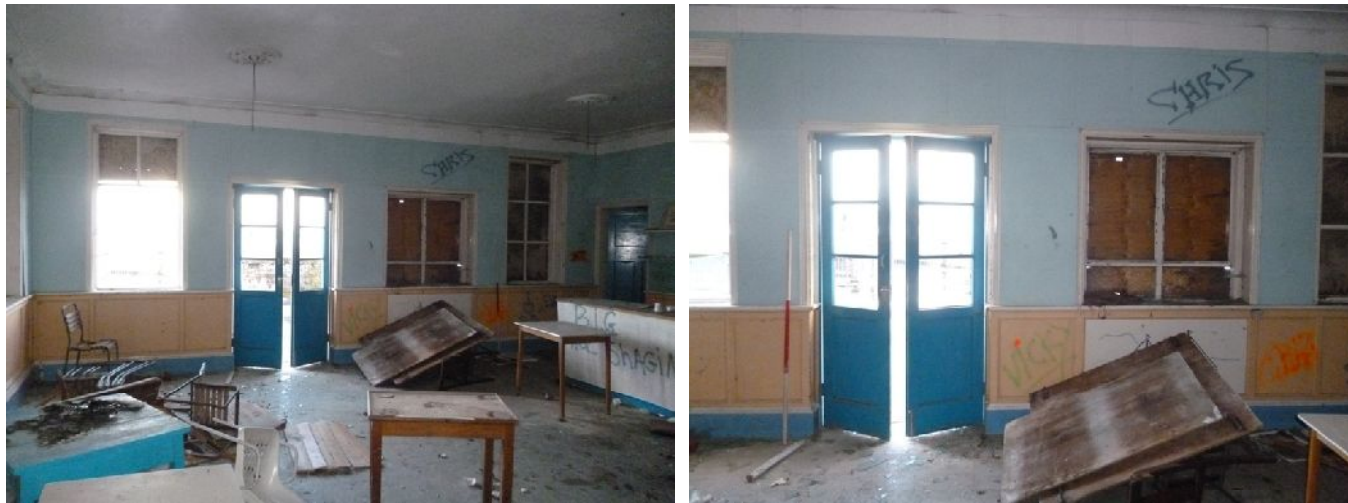
Plate 155 (left): East elevation of South Building, First Floor Room 1
