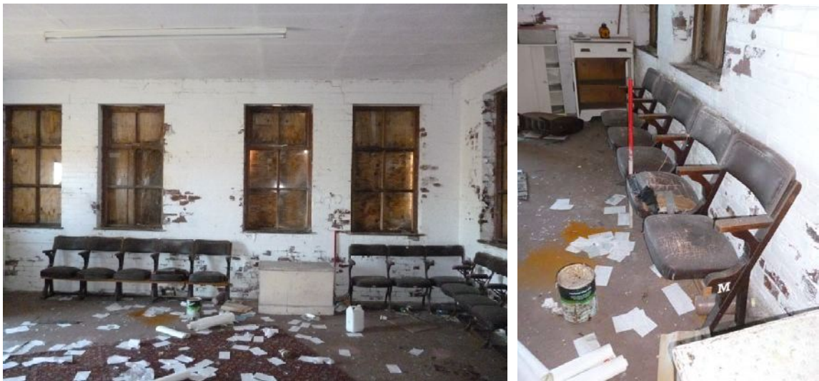
Plate 102 (left): South elevation of North Building, First Floor Room 1
