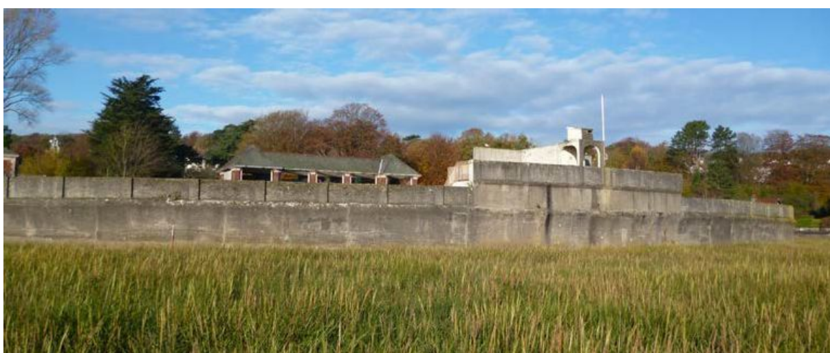
Plate 79: East side of the outer retaining wall
