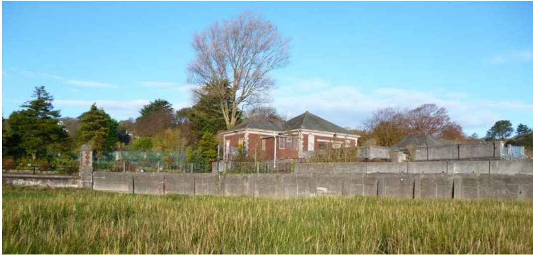
Plate 75: The southern side of the outer retaining wall from the south-east
