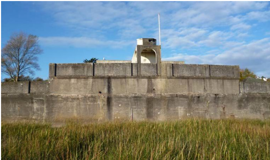
Plate 38: East elevation of the east building, showing the outer retaining wall
