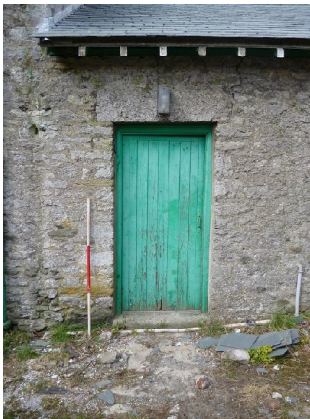
Plate 12: Plank door at north end of east external elevation
