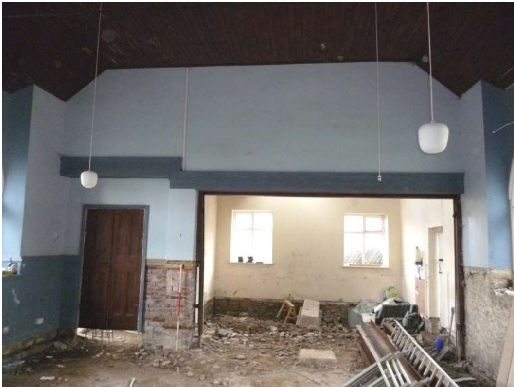
Plate 25: The north end of the south room
