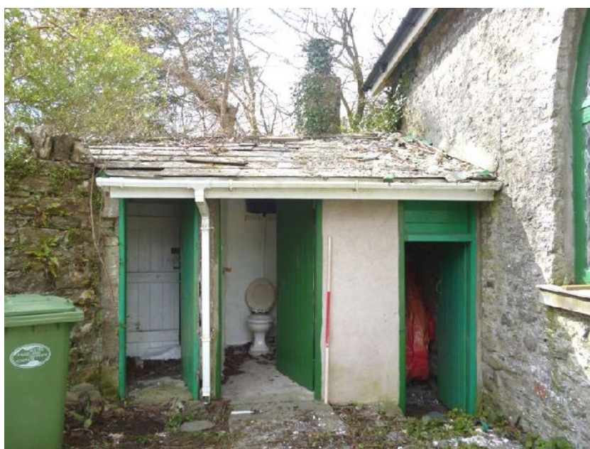
Plate 17 (left): Downpipe and dated hopper
