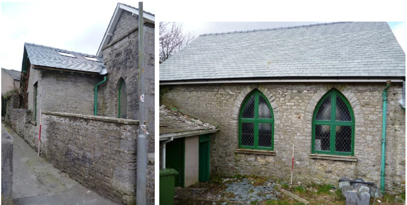
Plate 10 (left): North external elevation
