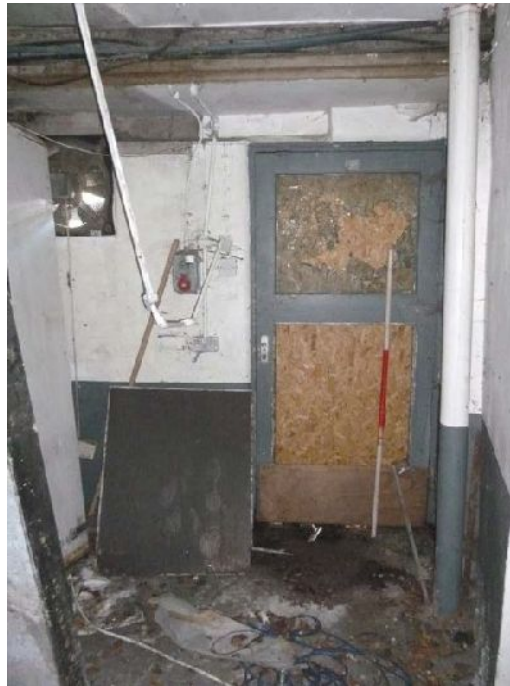
Plate 14: Doorway in the south-east elevation of Room G4
