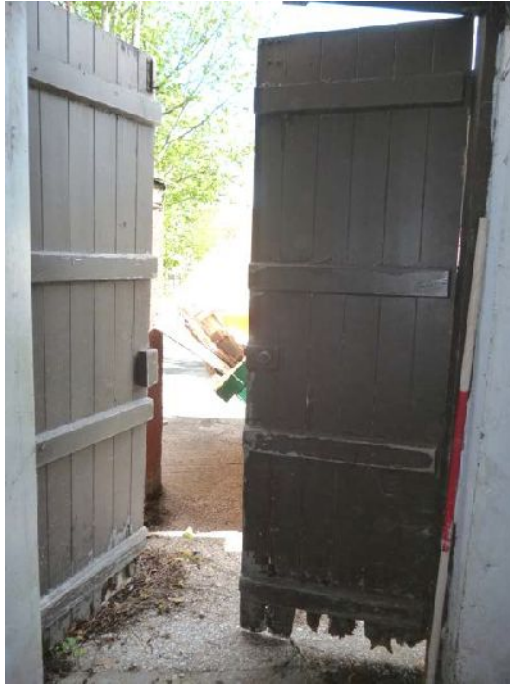
Plate 17: Double door in the south-east elevation of Room G6
