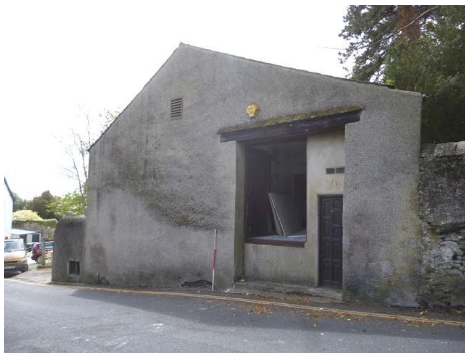
Plate 5: The north-east external elevation
