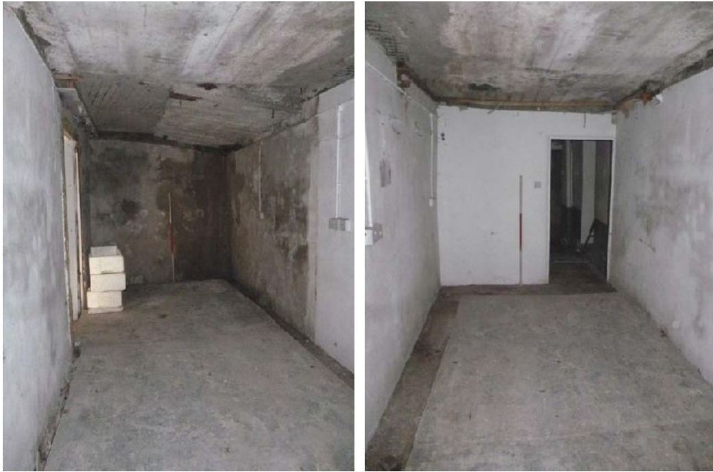
Plate 12 (left): North-west end of Room G2
