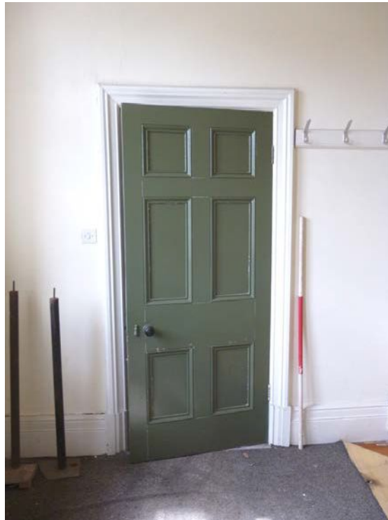
Plate 74: Doorway to the north-west, Room G21
