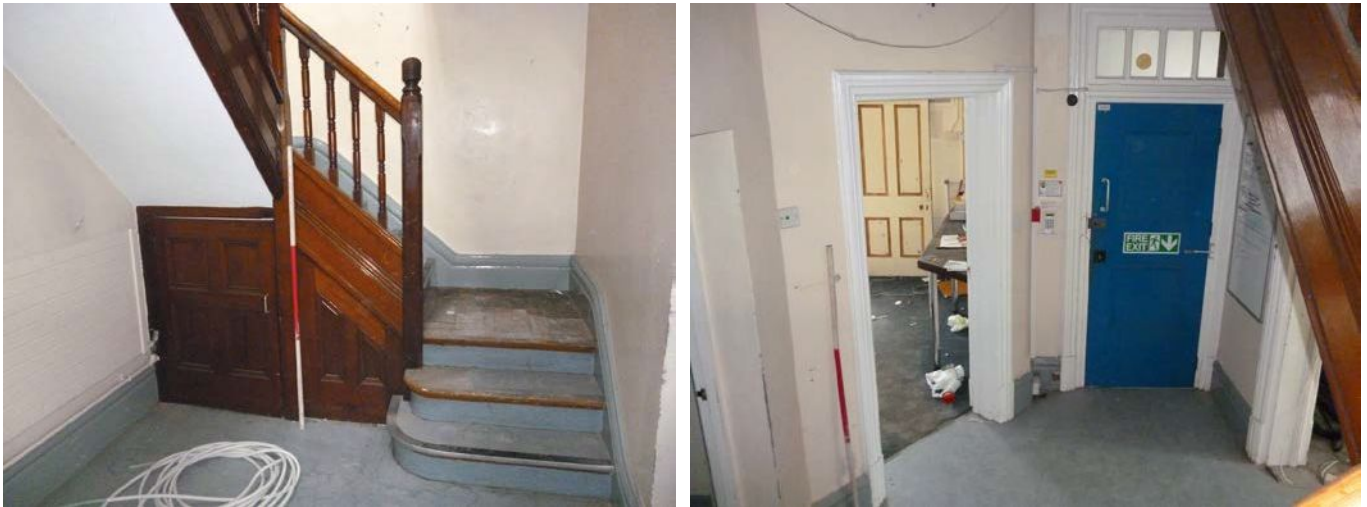
Plate 37 (left): Stairs on the south-west side of Room G3
