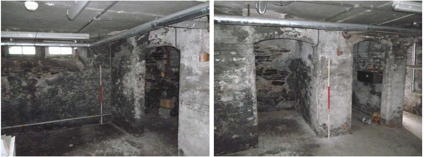
Plate 30 (left): Windows in the south-west elevation, basement main room
