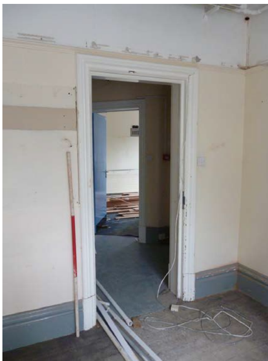
Plate 36: Doorway to north-west, Room G2
