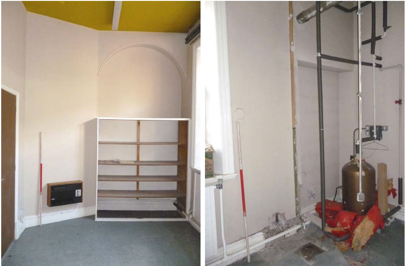
Plate 87 (left): Alcove and angled wall to the south-west, Room G26
