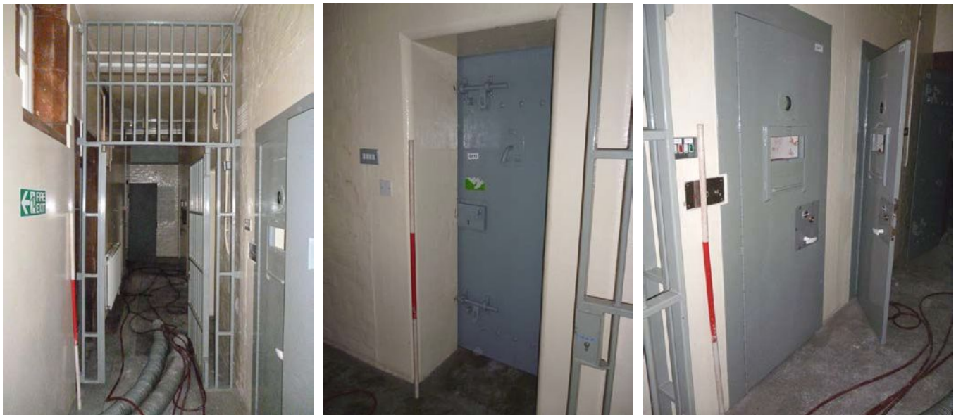
Plate 49 (left): Steel bar gate across Room G10
