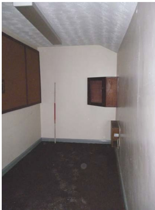
Plate 45: General view of Room G9
