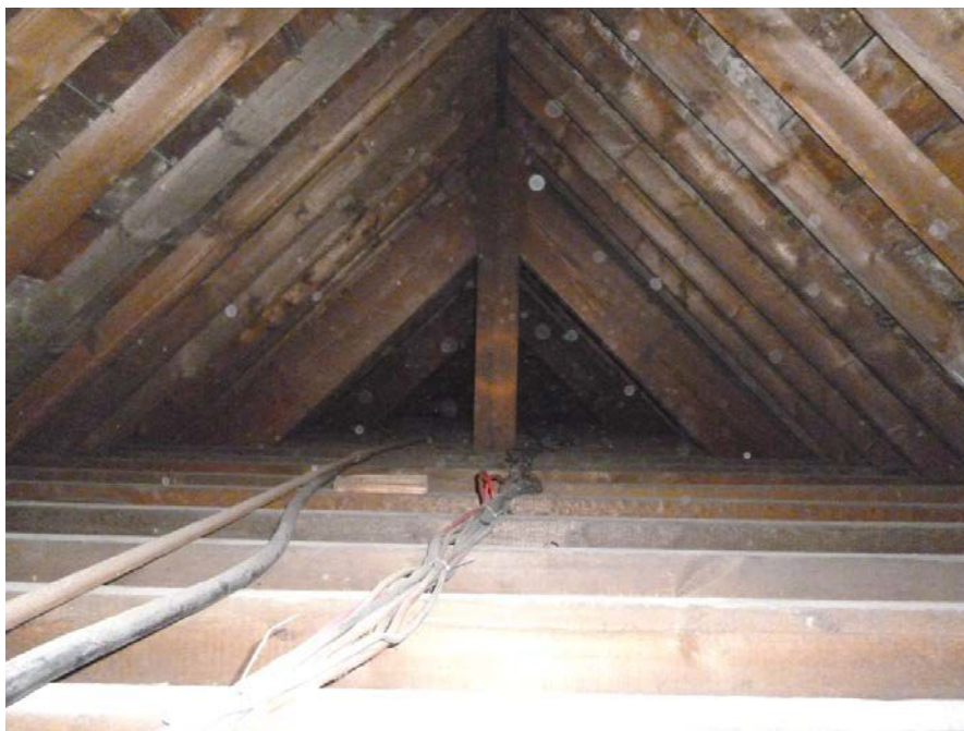
Plate 89: Roof structure above Room G22
