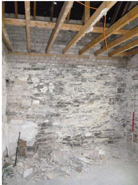
Plate 54: North-west elevation, Room G11
