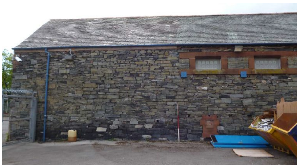
Plate 24: North-east end of the north-west external elevation
