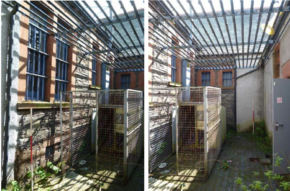
Plate 25 (left): South-east elevation of the yard
