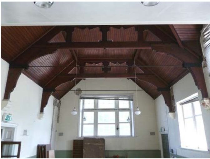
Plate 75 (left): Roof trusses in Room G22
