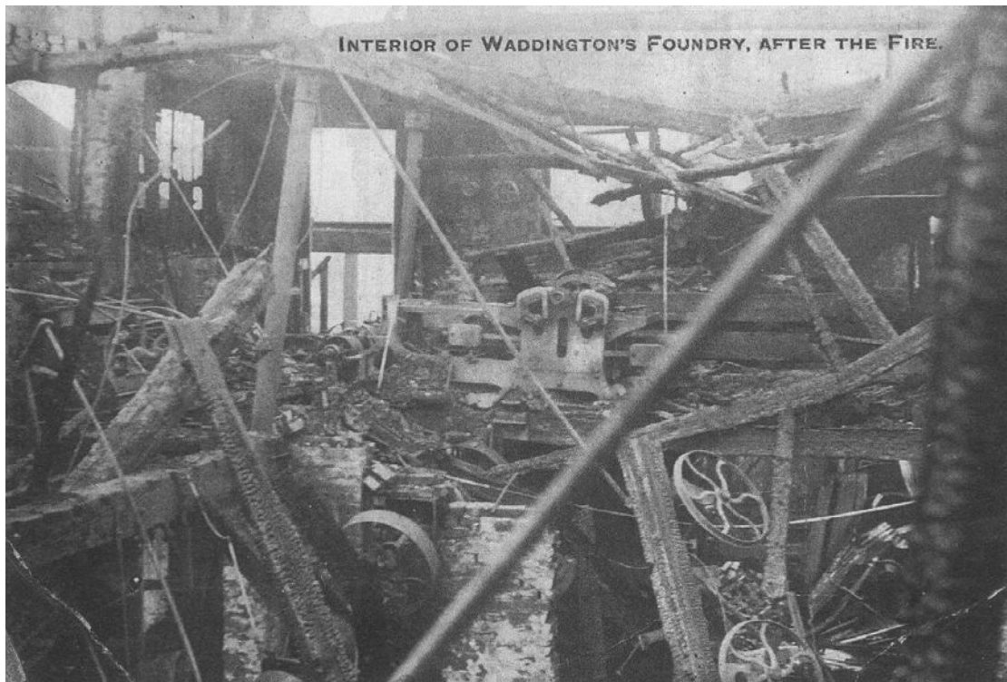
Plate 9: Detailed view of the foundry after the fire (from Myers 2000, 32)
