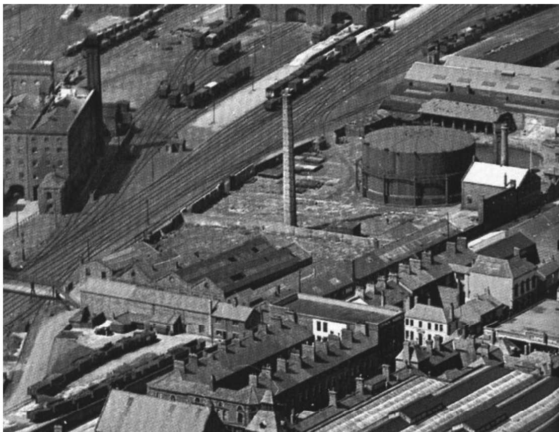
Plate 10: Aerial view of the gasworks and foundry (from Thompson 2005, ref AFR6237)
