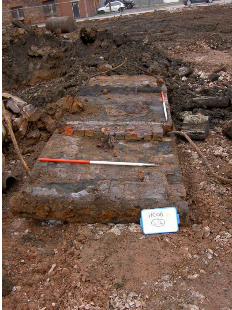
Plate 11: 'Underside' of cast iron 'baseplate' 414
