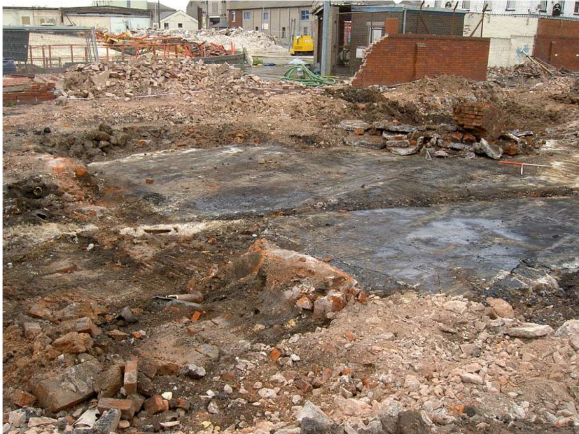
Plate 19: Floor slab 438 of Building 105 in Area C looking north-west
