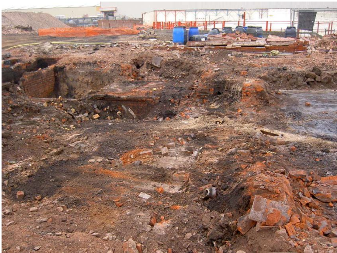
Plate 20: Tanks in or associated with Building 104 looking west
