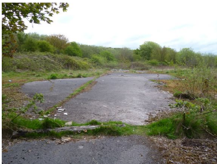
Plate 24: Concrete surface (Site 10)
