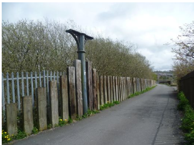
Plate 18 (left): South-west boundary constructed from re-used sleepers showing one of the incorporated bracketed iron columns
