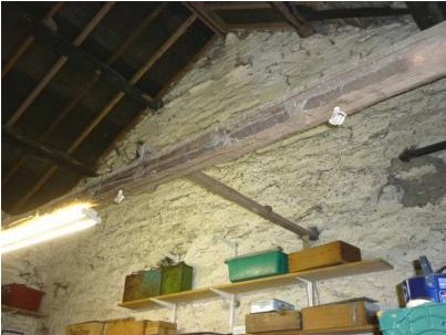
Plate 28 (left): Fire damage in the roof above Ground floor Room 3
