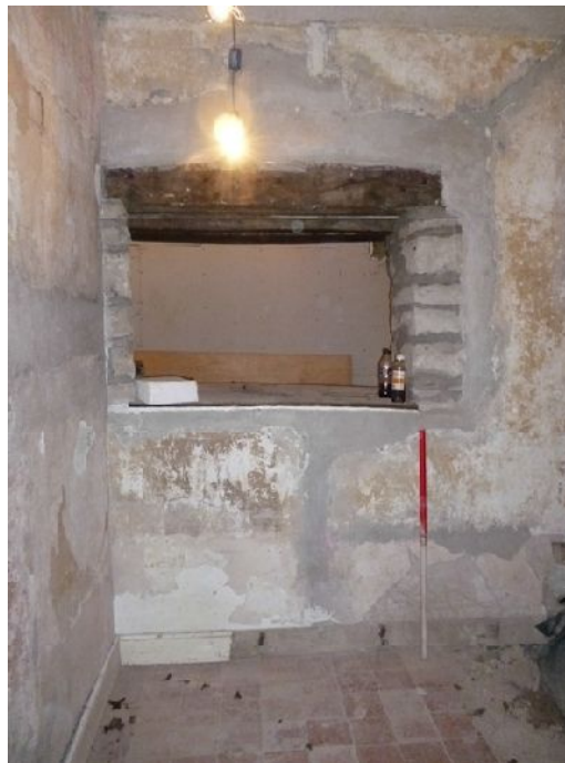
Plate 55: Window reveal in the east elevation of ground floor Room 9
