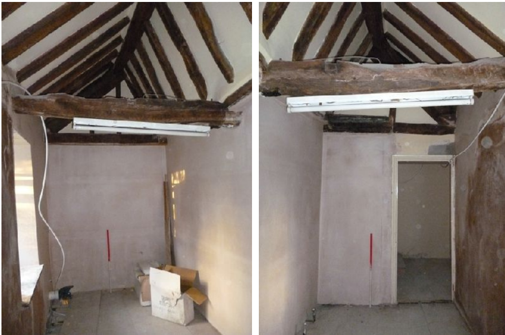
Plate 72 (left): North elevation of first floor Room 5
