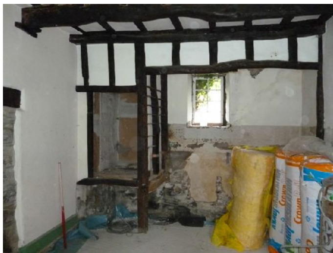
Plate 40: East elevation and cupboard in Room 6 on the ground floor
