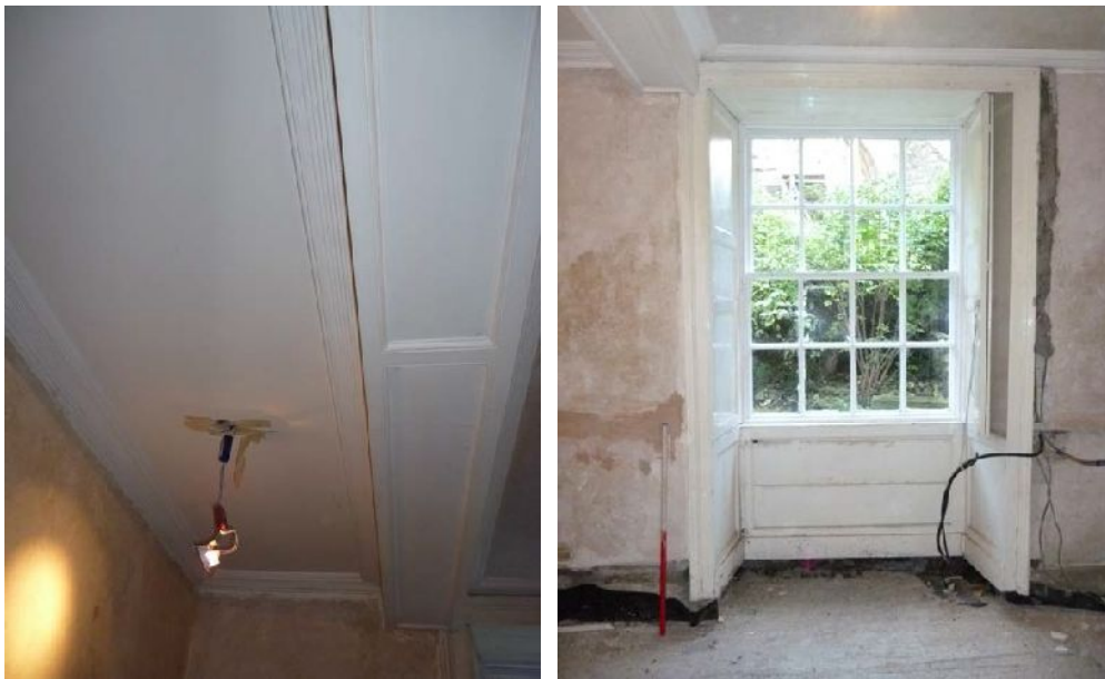
Plate 21 (left): Beam and cornice in ground floor Room 1
