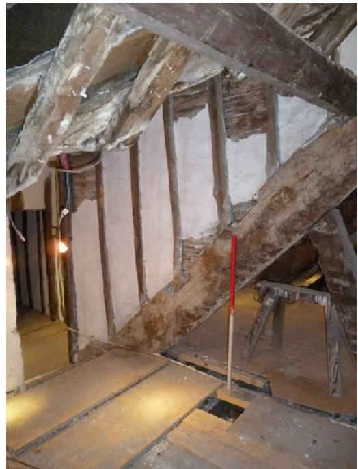
Plate 93 (left): Wind braces cut through to the west, second floor Room 1
