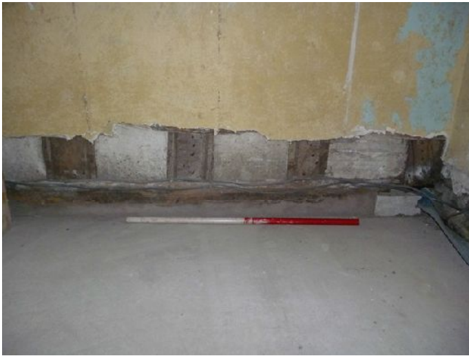
Plate 60 (left): Earlier beaded studs in the south elevation of ground floor Room 10
