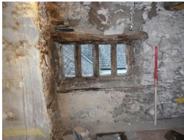
Plate 97: Mullion window in the north elevation of second floor Room 1
