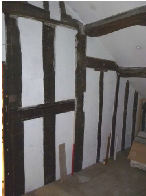
Plate 102: East elevation of second floor Room 2
