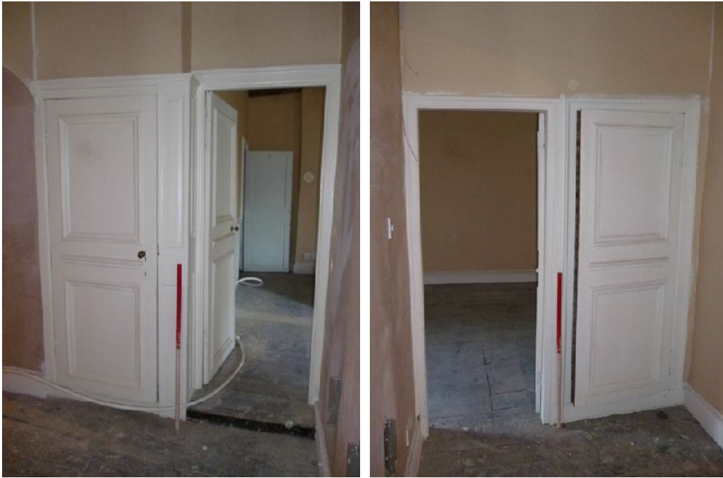
Plate 66 (left): North elevation of first floor Room 2
