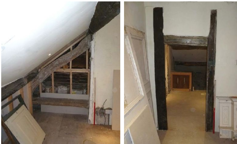
Plate 107 (left): North end of the east elevation of second floor Room 4
