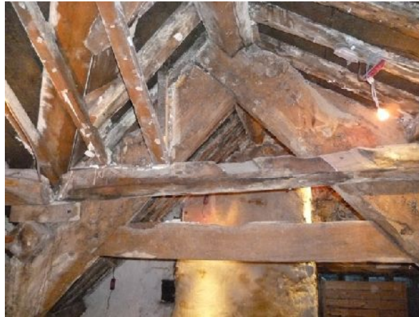
Plate 88: Top of the north truss in second floor Room 1
