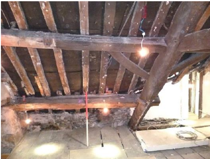
Plate 93 (left): Wind braces cut through to the west, second floor Room 1
