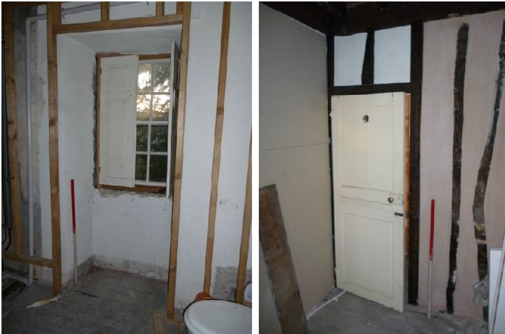
Plate 78 (left): Window in the west elevation of first floor Room 7
