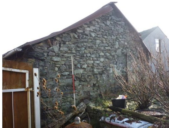
Plate 13: West external elevation
