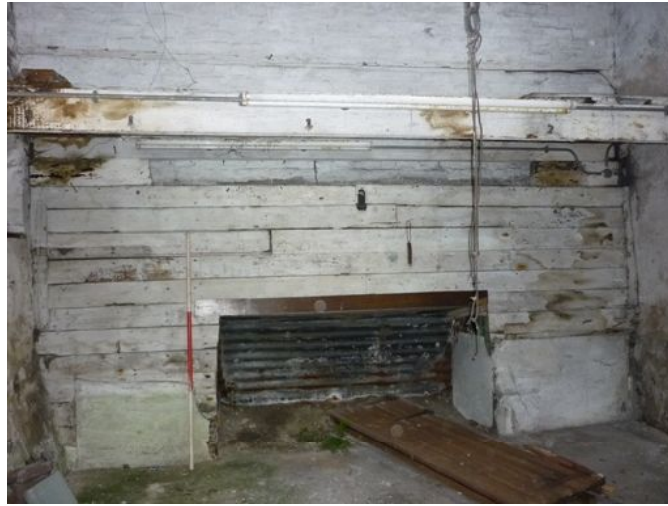
Plate 25: Opening in the west elevation below the half loft
