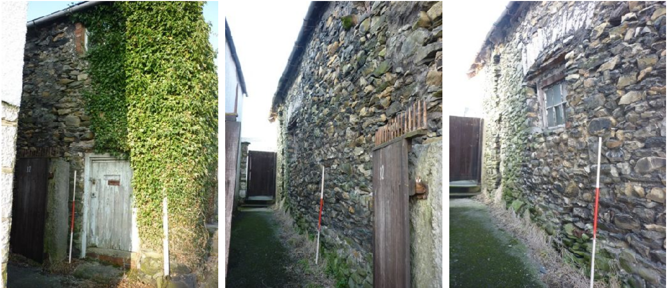
Plate 10 (left): East end of the south external elevation
