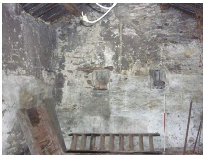
Plate 20: West elevation of Room 1
