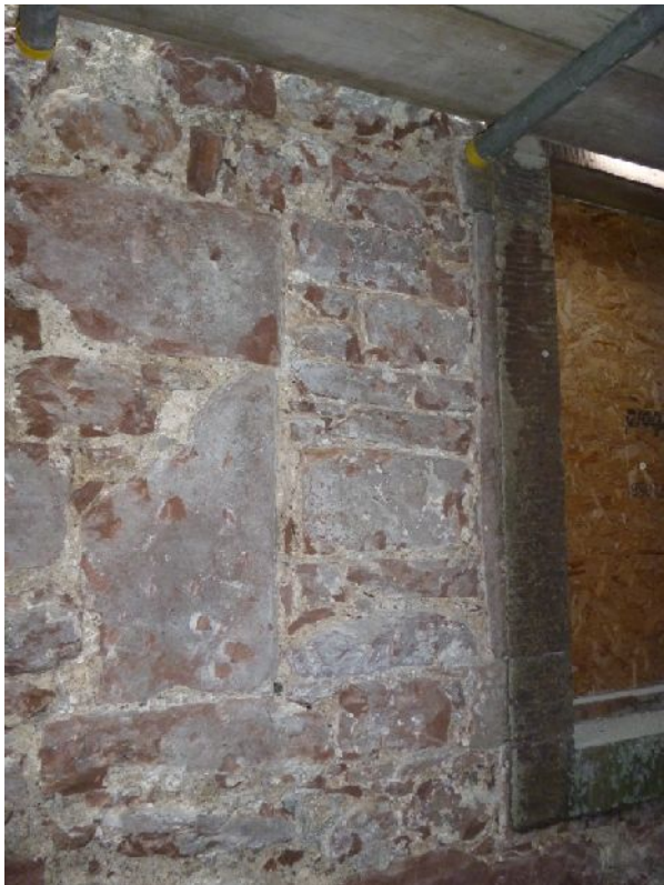
Plate 30 (left): Blocked window truncated by extant window in the north elevation of the nave
