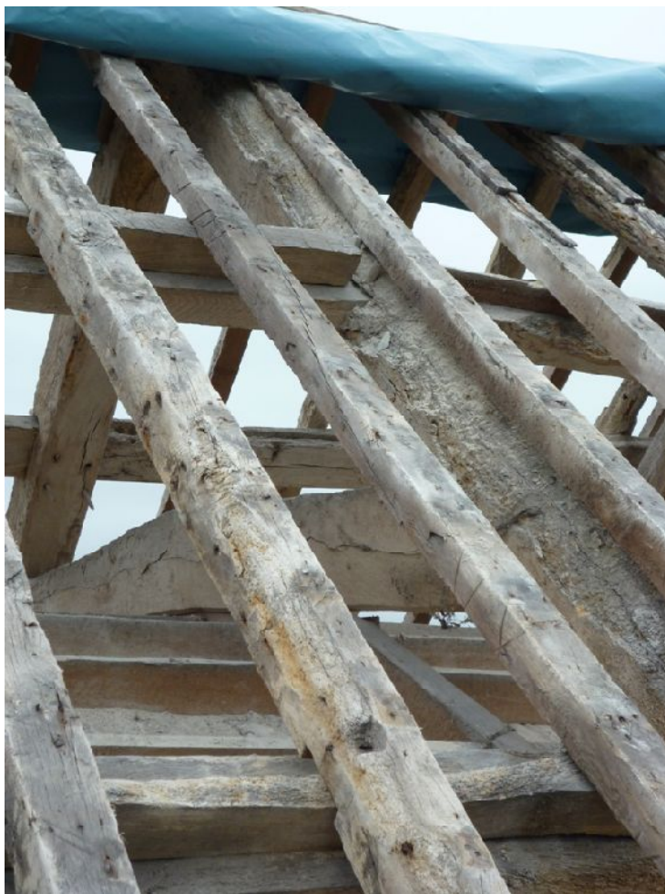
Plate 15: Exposed roof showing truss and rafter with Baltic marks
