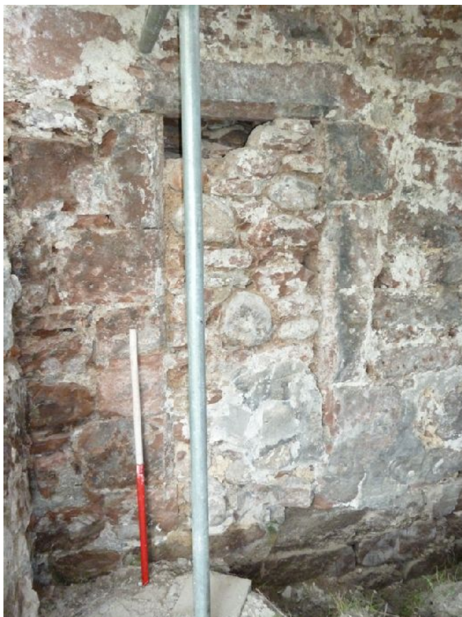
Plate 24 (left): Blocked two-light window with cusped heads, south elevation of the chancel
