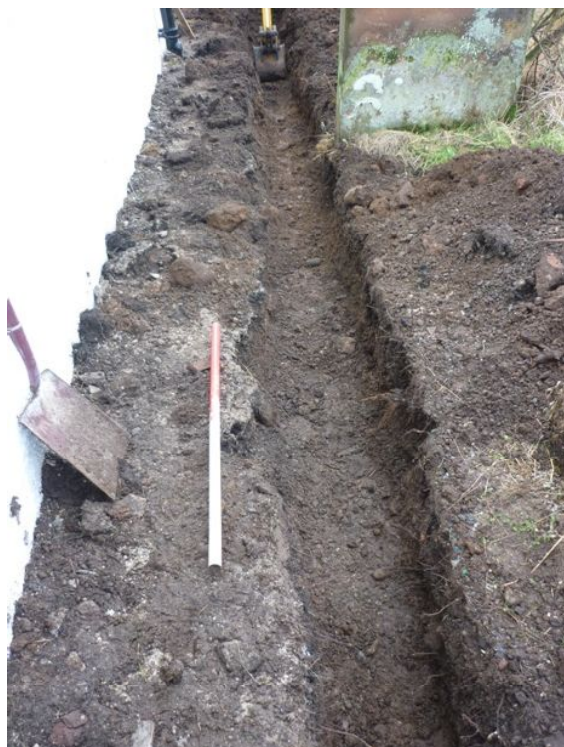
Plate 36 (left): Drainage trench along the north side of the nave
