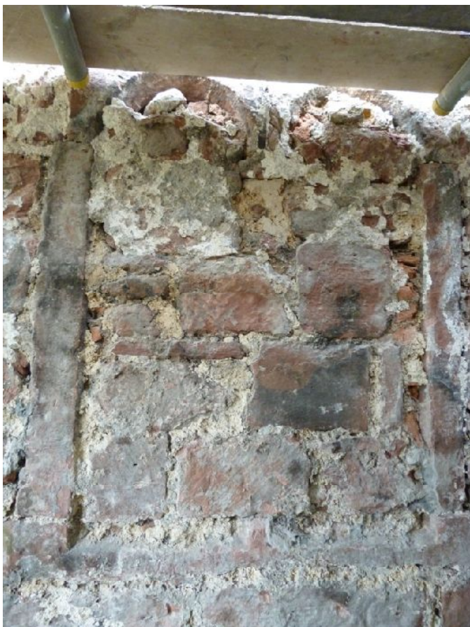
Plate 24 (left): Blocked two-light window with cusped heads, south elevation of the chancel
