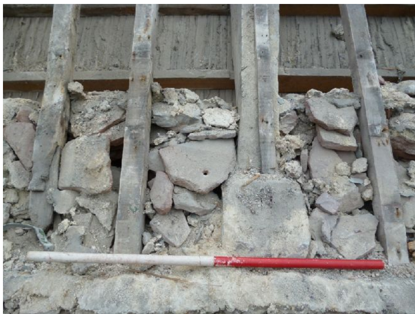
Plate 18: Stone roof tiles exposed on the north side
