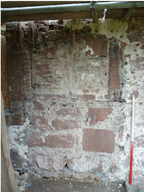
Plate 22 (left): Blocked two light mullion window, south elevation of the chancel in Fabric 2
