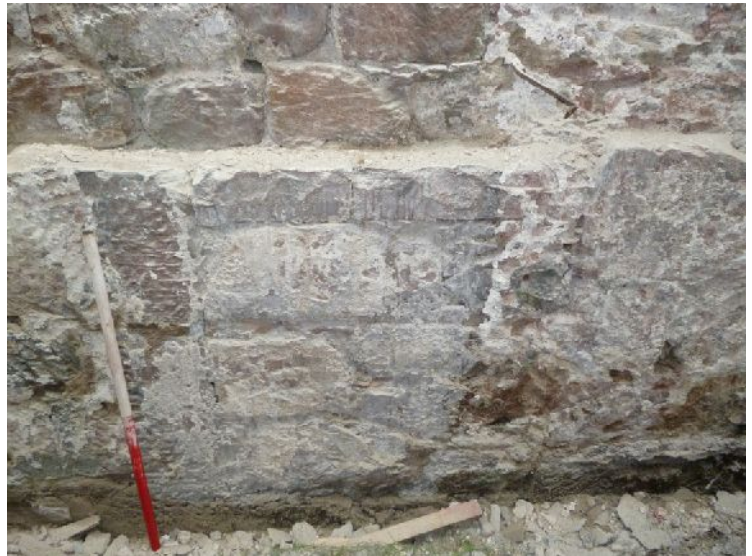
Plate 22 (left): Blocked two light mullion window, south elevation of the chancel in Fabric 2
