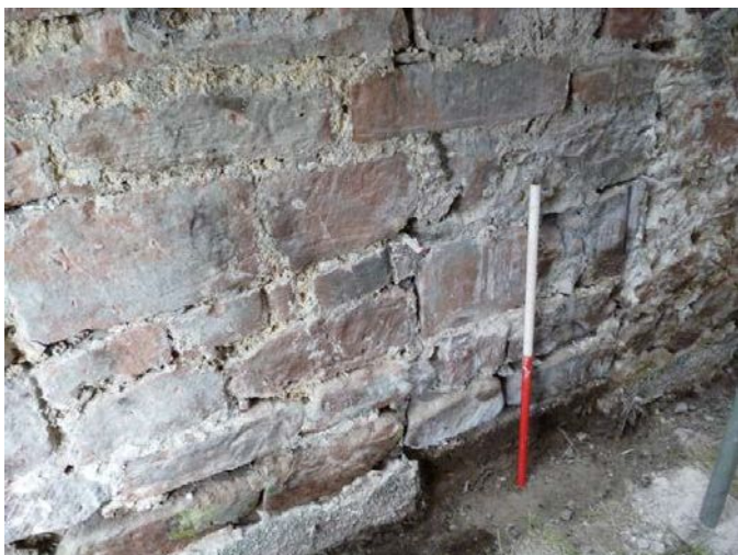
Plate 26 (left): Re-used pieces of dressed and worked stone below the blocked window, south elevation of the chancel
