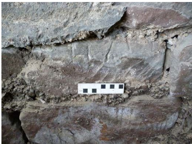
Plate 26 (left): Re-used pieces of dressed and worked stone below the blocked window, south elevation of the chancel
