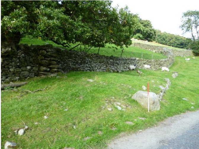
Plate 57 (left): Ruined building, viewed from the west (Site 31)
