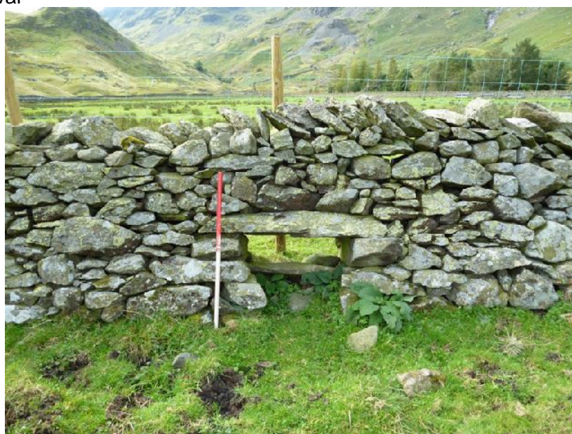
Plate 27: Hogg-hole, viewed from east (Site 9)
