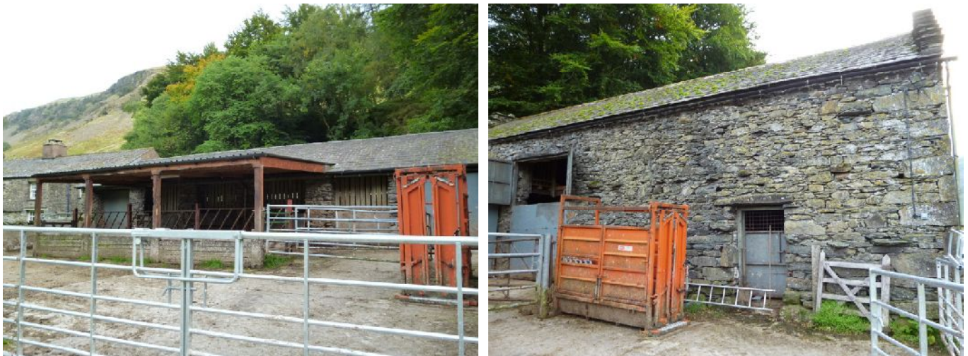
Plate 75 (left): Cart sheds at Elmhow, viewed from the north (part of Site 44)
