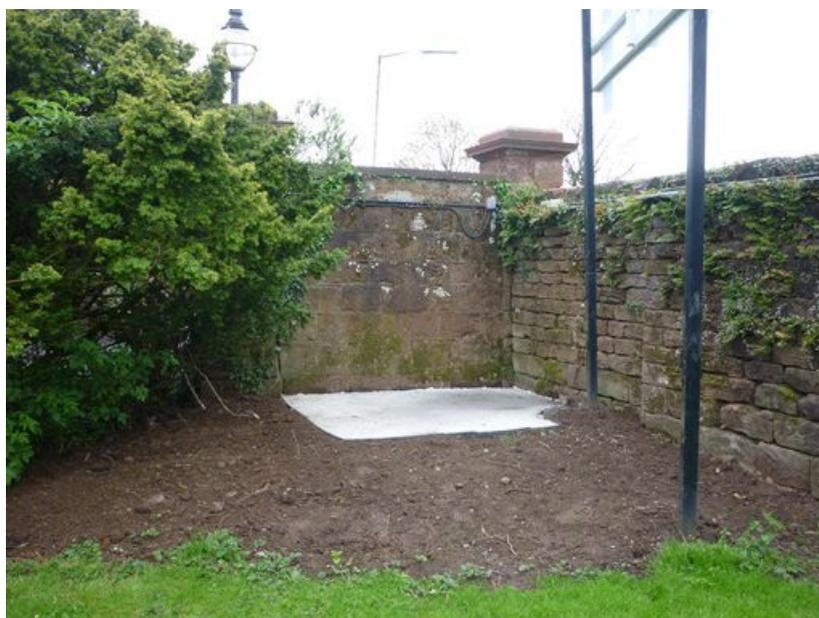
**Plate 1: New sign to be fixed into concrete base at Item 1 location required no excavation**
