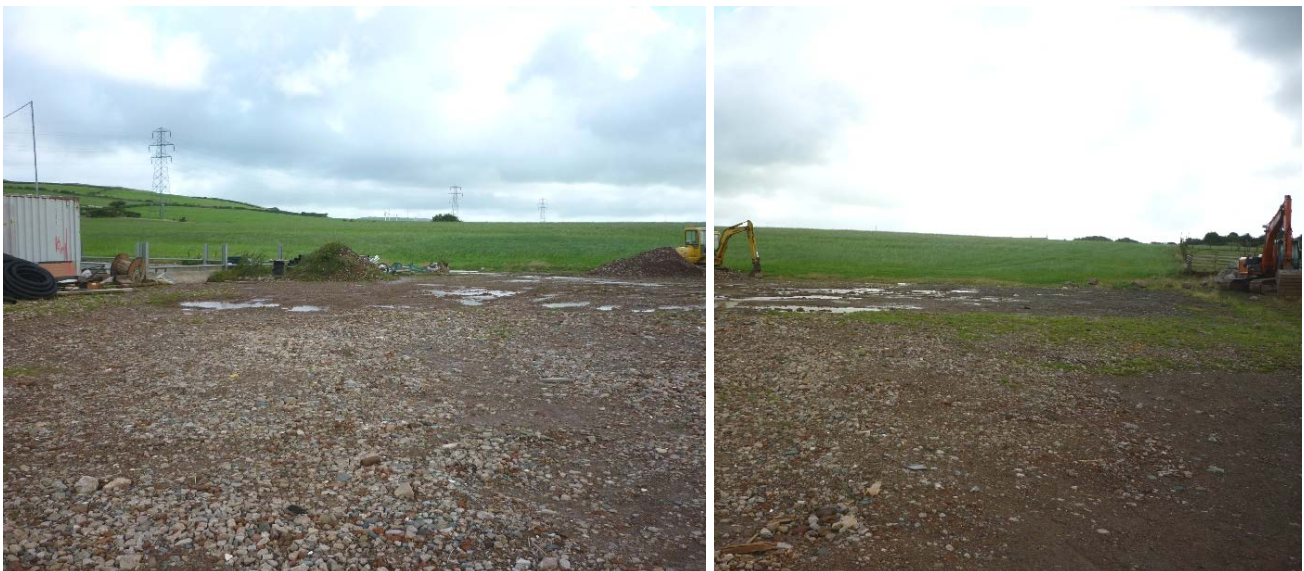
Plate 1 (left): Pre-excitation view of the site from the south-west
