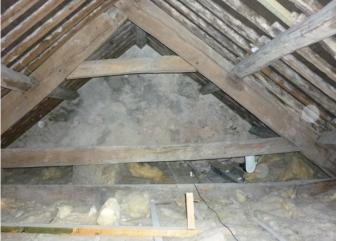
Plate 79 (left): Typical roof truss over the southern section of the hall
