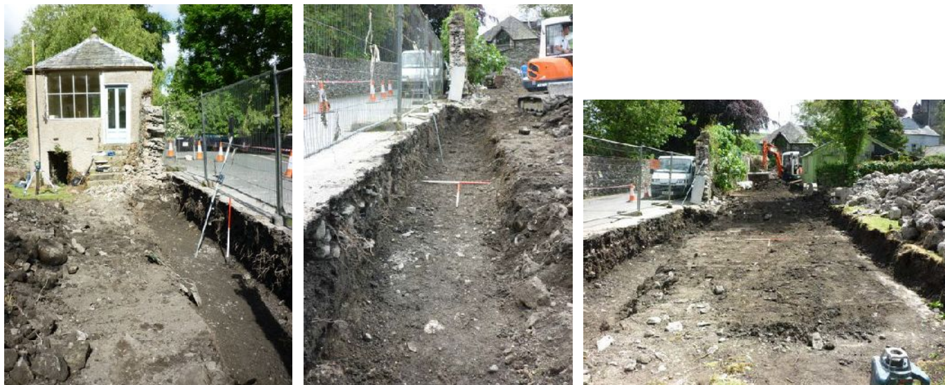
Plate 9 (left): Excavation below the boundary wall along Priest Lane, looking west
