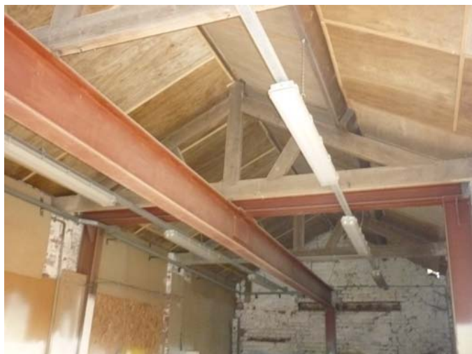
Plate 29 (left): Truss and additional steel beams in Room 1, Building 1, viewed from the east
