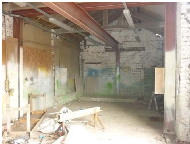
Plate 29 (left): Truss and additional steel beams in Room 1, Building 1, viewed from the east
