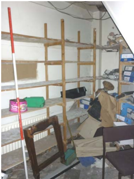
Plate 49: General view of ground floor Room 5, Building 2, viewed from north-west
