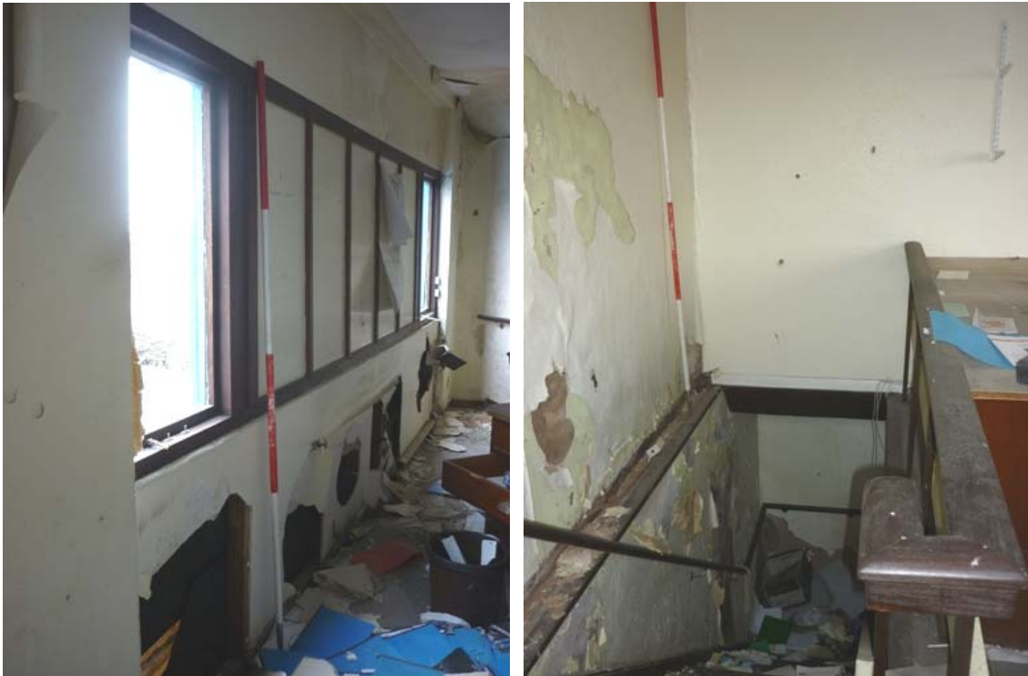
Plate 56 (left): Windows and stud walling in east elevation, first floor Room 4, Building 2
