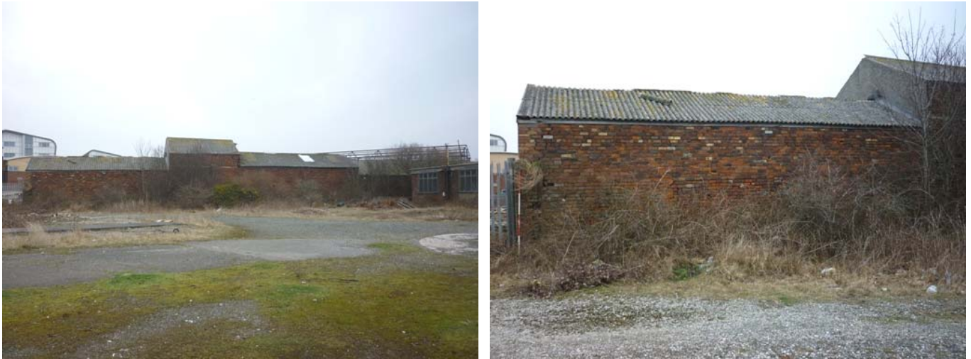
Plate 21 (left): Building 1, south external elevation, viewed from the south
