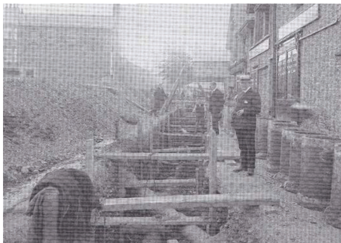
Plate 21 (left): Excavation for mains sewage in Kendal in the early 20 th century, showing timber shoring (from Duff and Duff 1997, 105)
