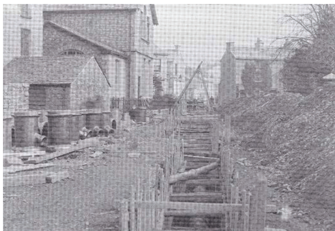
Plate 21 (left): Excavation for mains sewage in Kendal in the early 20 th century, showing timber shoring (from Duff and Duff 1997, 105)
